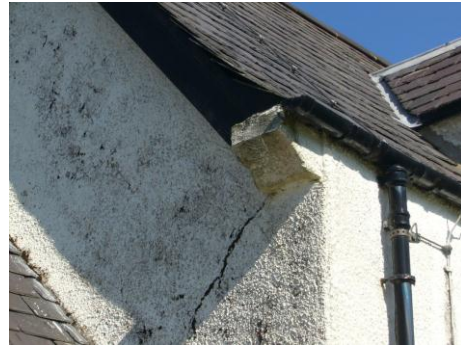
8. North West – Corbel Detail
