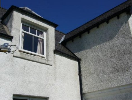
7. South West – Dormer Window
