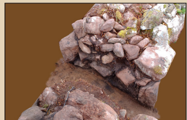
This cross-section shows the outer and inner facings made of large stones, infilled with smaller stones
