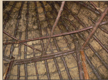
A reconstruction: rafters, and the upper ring-beam with extra tension beams
