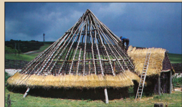
Another reconstruction (wooden-walled) being thatched
