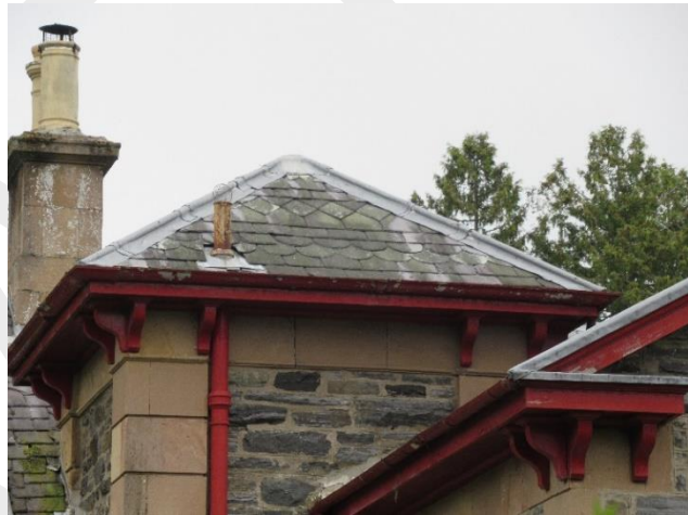
Fig. 38 Fish-scale and diamond slate tiling detail
