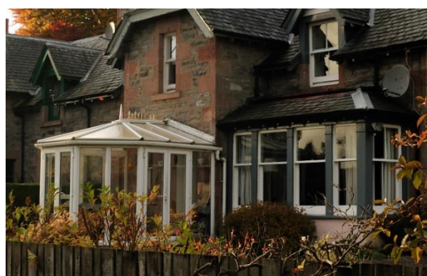
Fig. 70 Inappropriate conservatory extension
