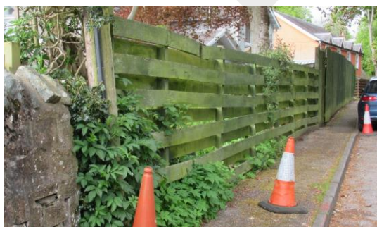
Fig. 71 Inappropriate timber fencing
