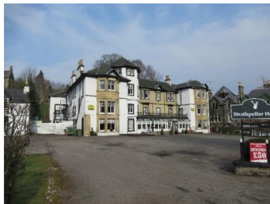
Fig. 72 Hard landscaping, Strathpeffer Hotel
