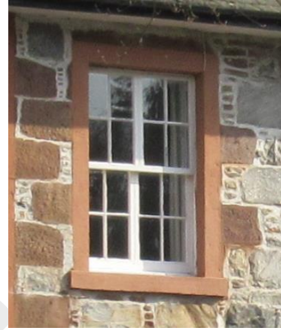
Fig. 44 8 over 8-pane sash and case window
