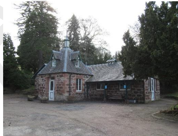
Fig. 27 Upper Pump Room
