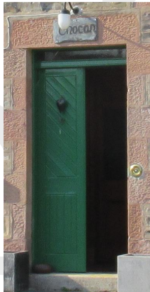
Fig. 46 Double leaf, plank and batten timber door with top light
