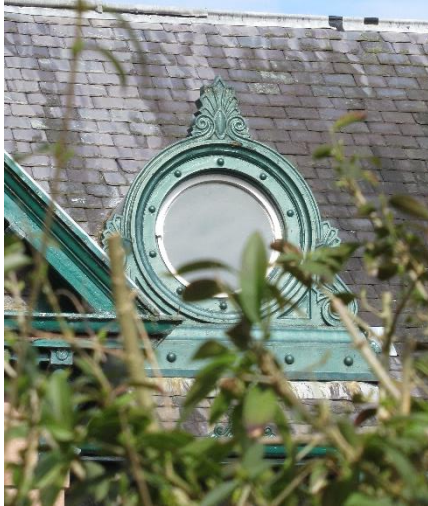
Fig. 42 Ornate cast iron dormer window
