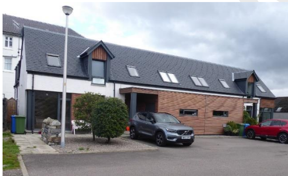
Recent example of sympathetic new development in the Conservation Area maintaining a low storey height and long form typical of traditional outbuildings in the backland areas. Slate roof and contemporary design for elevations.
