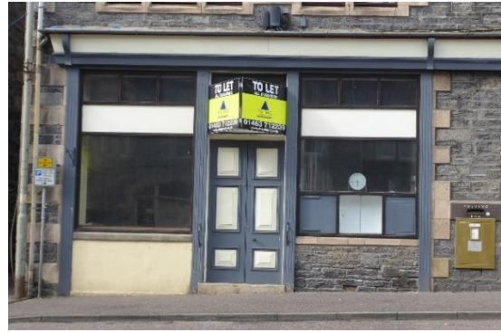
No. 7 High Street, the former Post Office, had a very large late Victorian shop frontage, the basic form of which survives (right), although there has been some adaptation and replacement. Note the individually mounted lettering on its original fascia, a suitable signage approach today and used on the neighbouring Mortimer's.
