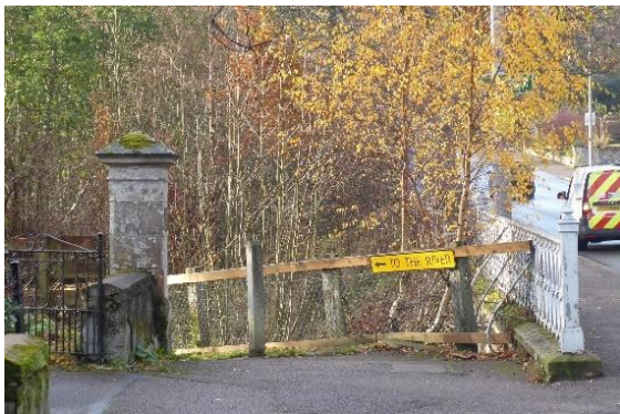
Low quality timber/wire fencing and concrete bollard detract from the historic setting with decorative iron bridge railings; the standard yellow & black signage is highly visible but could be provided with a more sympathetic signage design and material for this attractive historic and natural setting.
