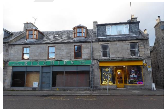
No. 7 High Street, the former Post Office, had a very large late Victorian shop frontage, the basic form of which survives (right), although there has been some adaptation and replacement. Note the individually mounted lettering on its original fascia, a suitable signage approach today and used on the neighbouring Mortimer's.
