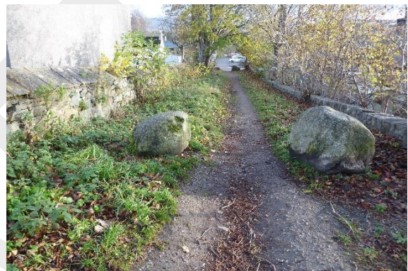
View towards South Street on the lane next to the Grant Arms hotel, traditional stone walls, trees and vegetation add interest but the footpath's surface condition and width makes it difficult for some users.
