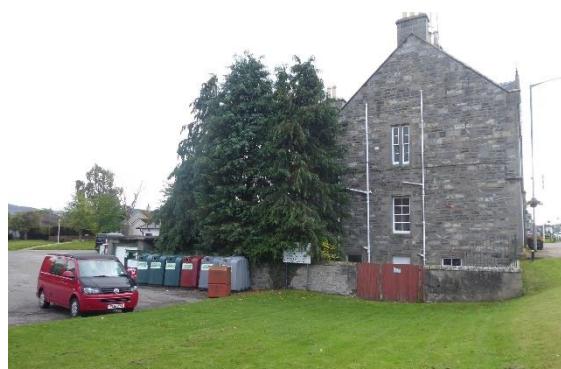
Recycling facilities at the east side of the Court House are unattractive.
