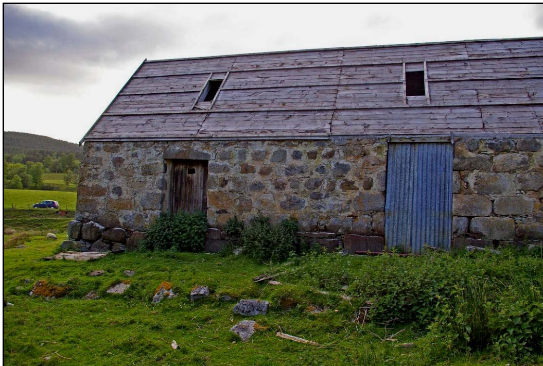
Figure 4 Barn, showing foundations and ashlar stonework
