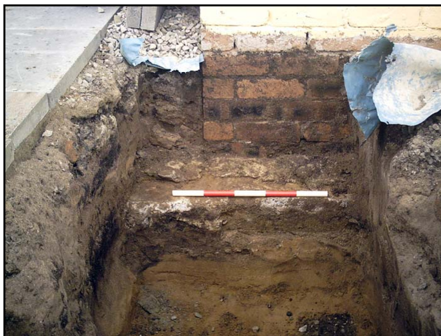
Figure 6 Footings of present house (50cm scale in 10cm divisions)
