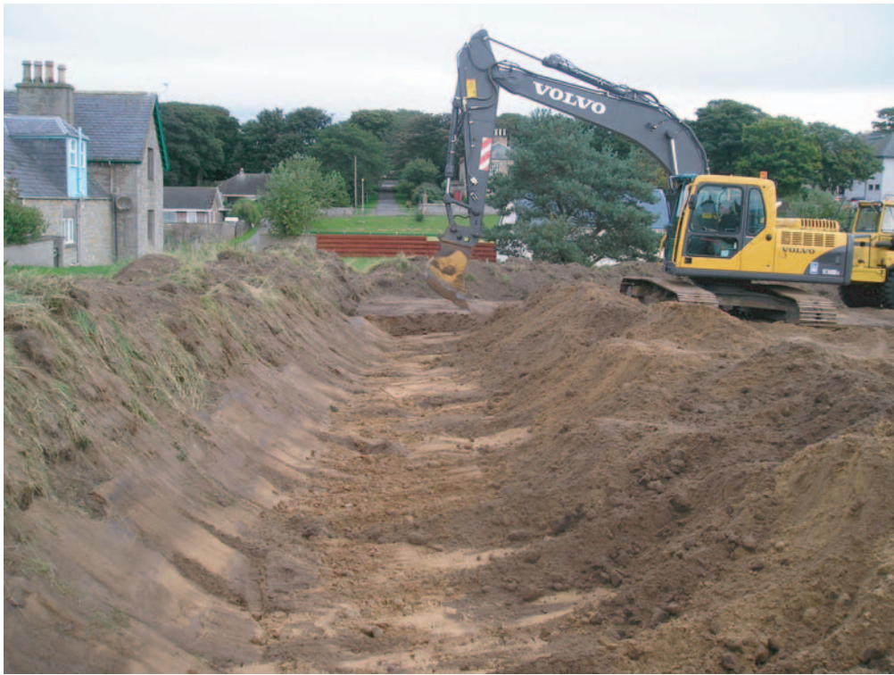
Plate 3: View of the site looking N showing the gravel 'beach' beneath the sand
