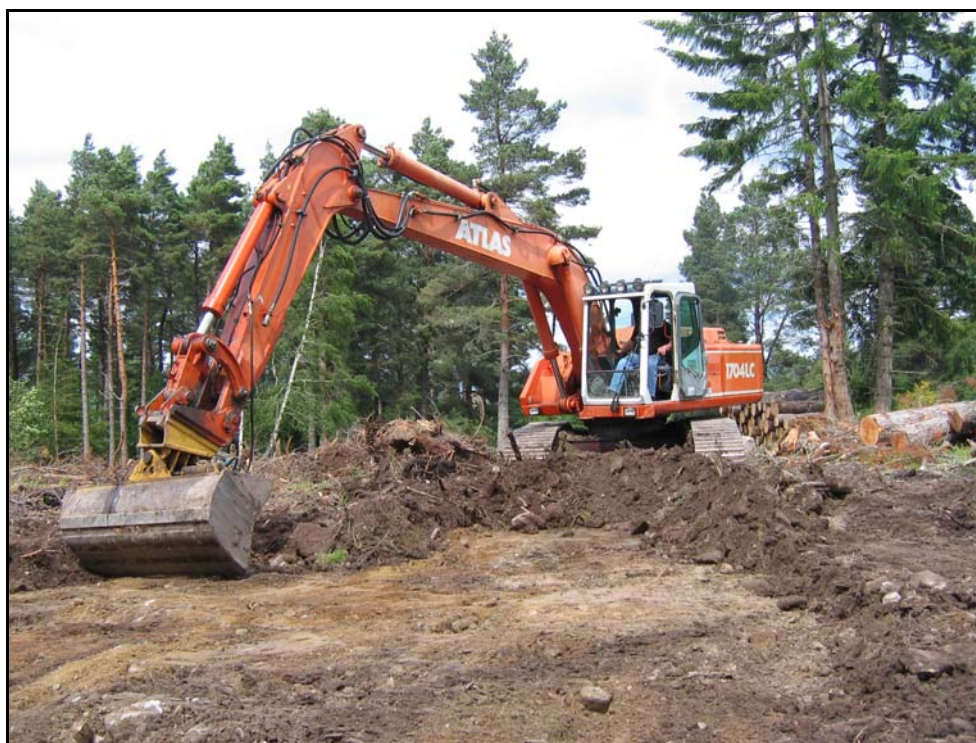
Figure 7 Extending trench to septic tank
