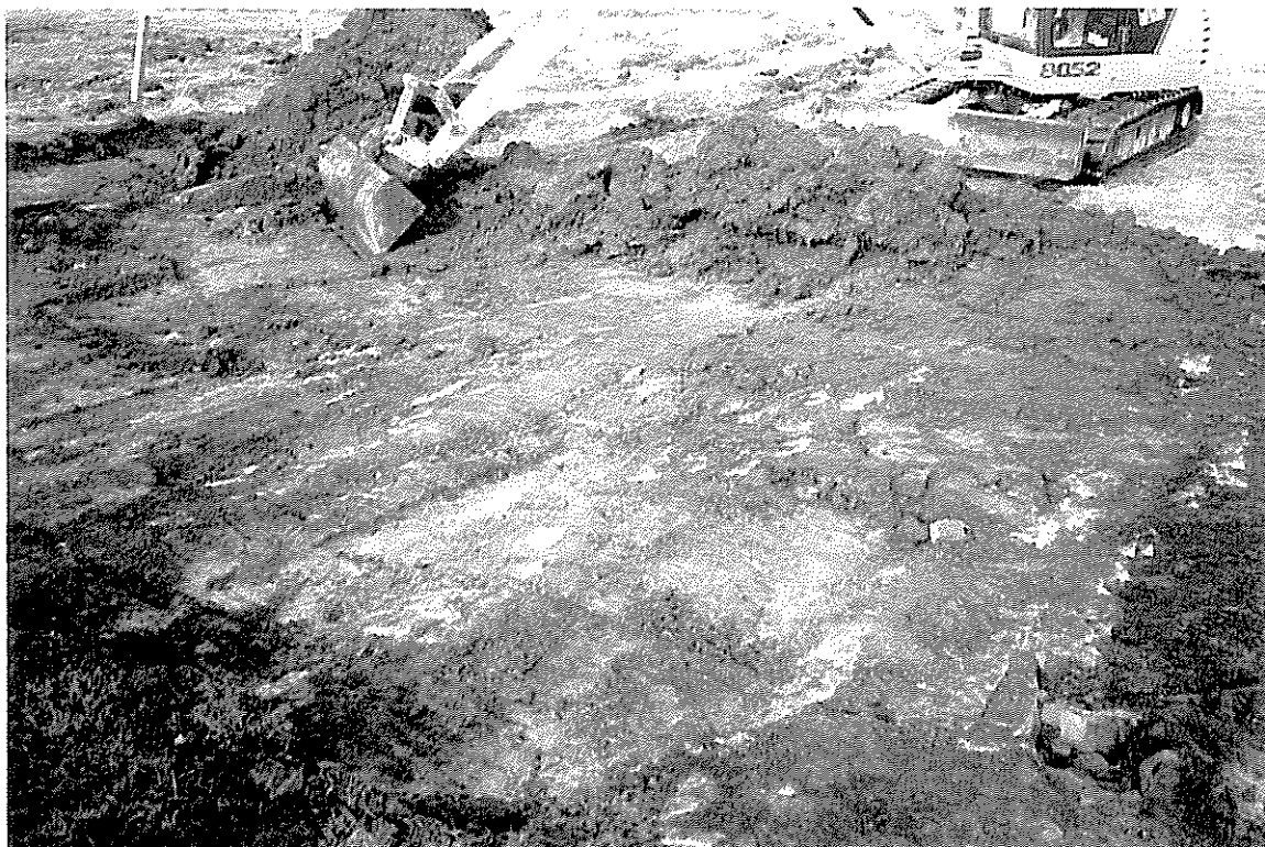
Bedrock as exposed during removal of the topsoil.
