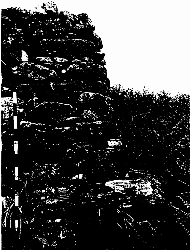
No. 189a. W corner and plinth.
