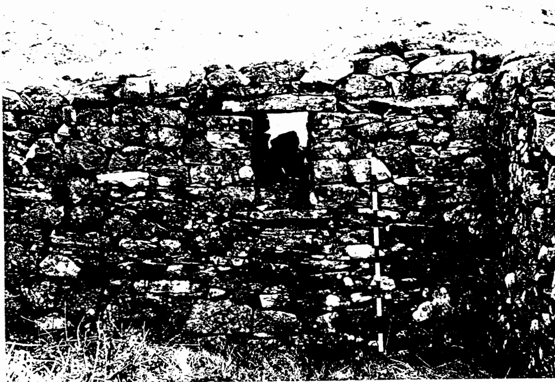
No. 28a Internal face of W end, showing cruck slot, window and drain.
