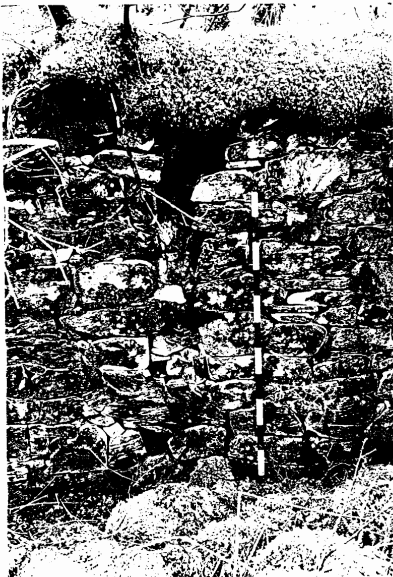
No. 34 Cruck slot iii) in W wall of N compartment.
