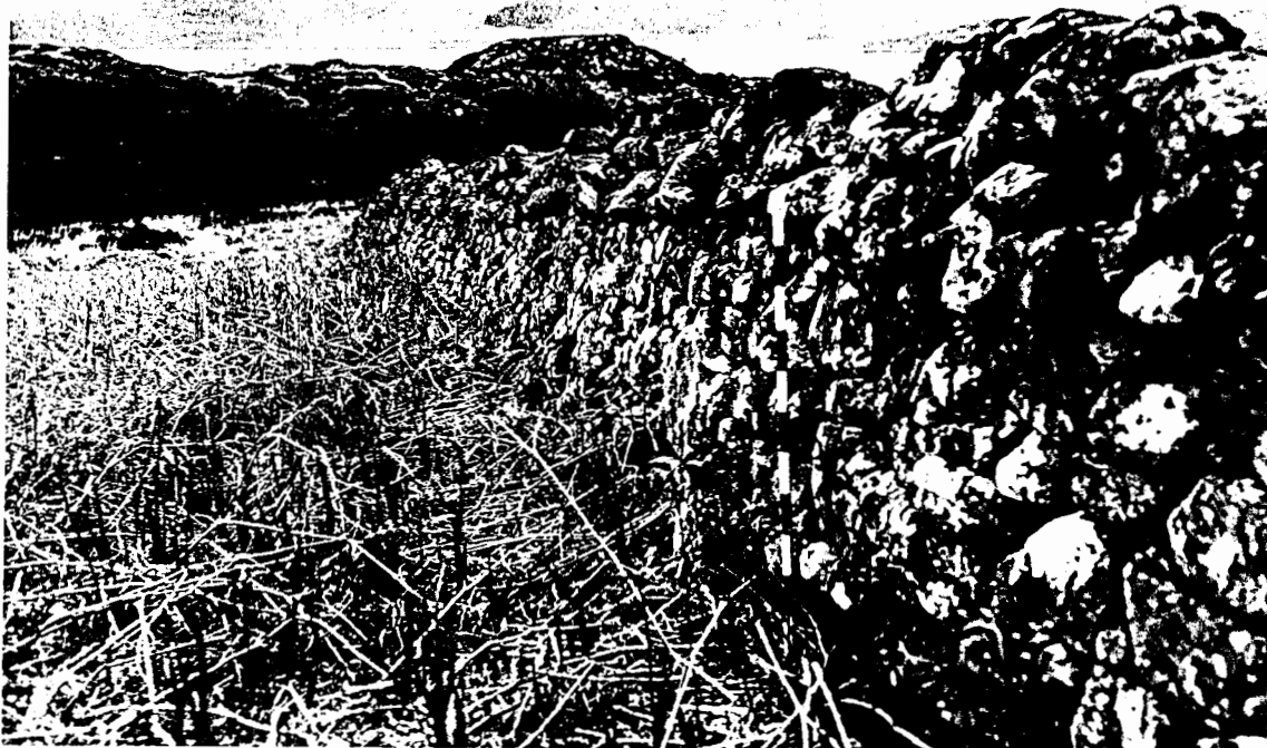
No. 176a. Boundary wall, from SE. Note course of transversely-set stones.
