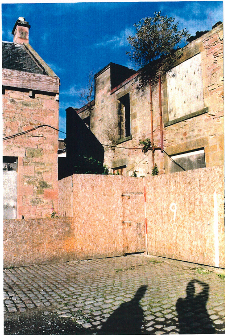
Building 2, south facing wall
