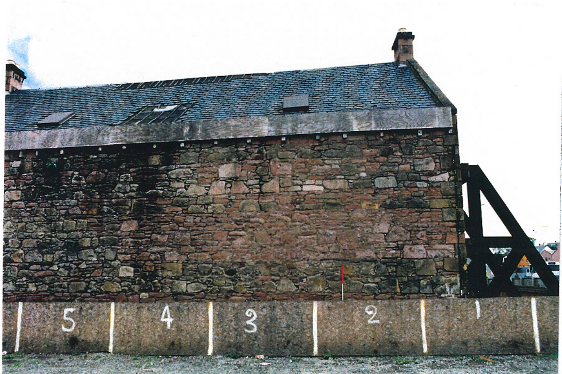
Building 1, west facing wall
