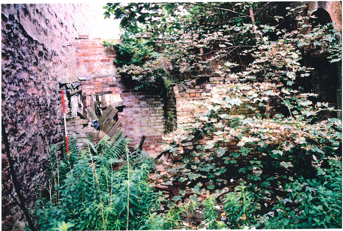
Building 3, south facing wall
