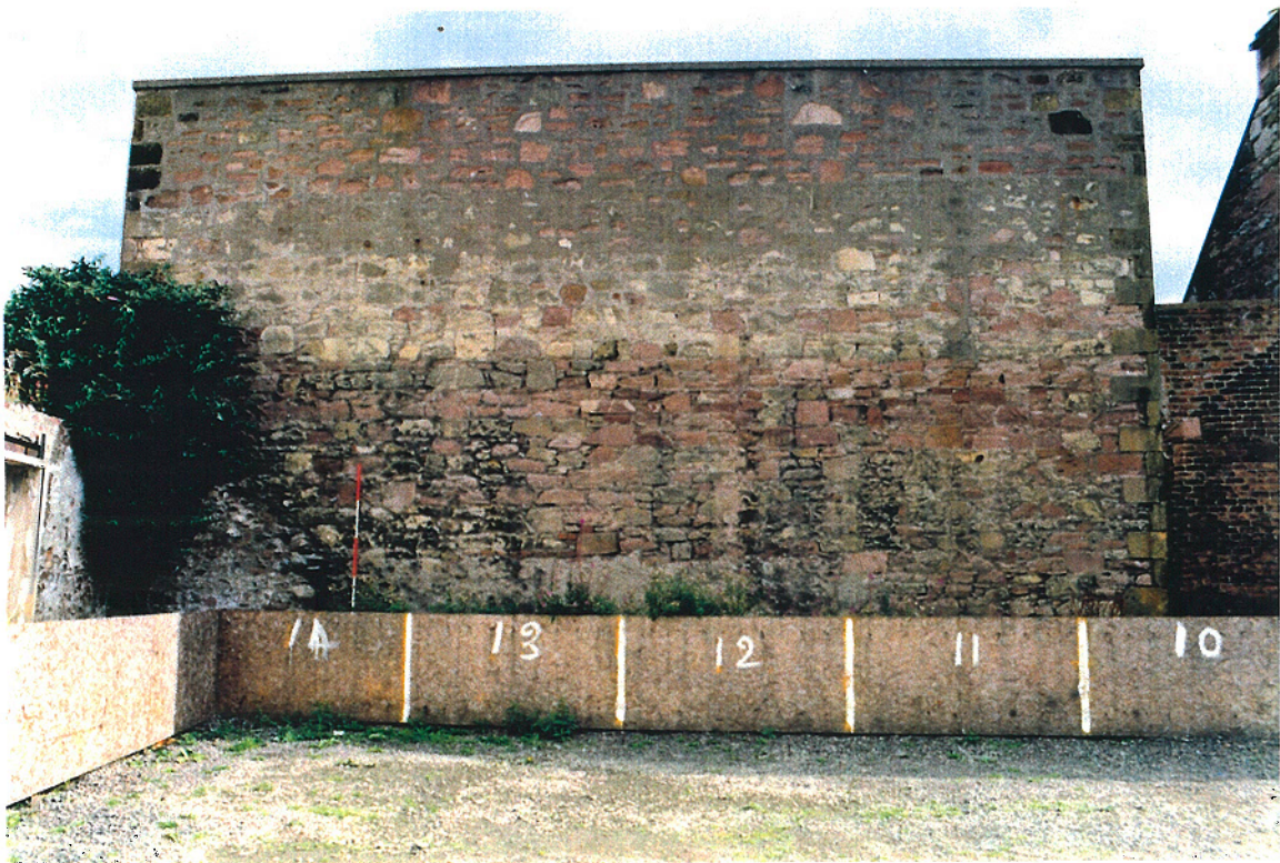
Building 2, west facing wall
