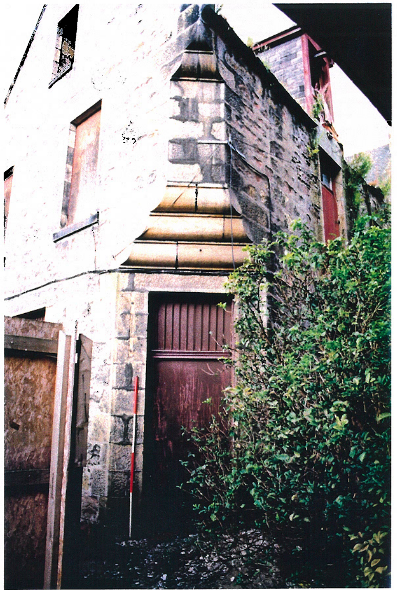
Building 2, detail of south-east corner
