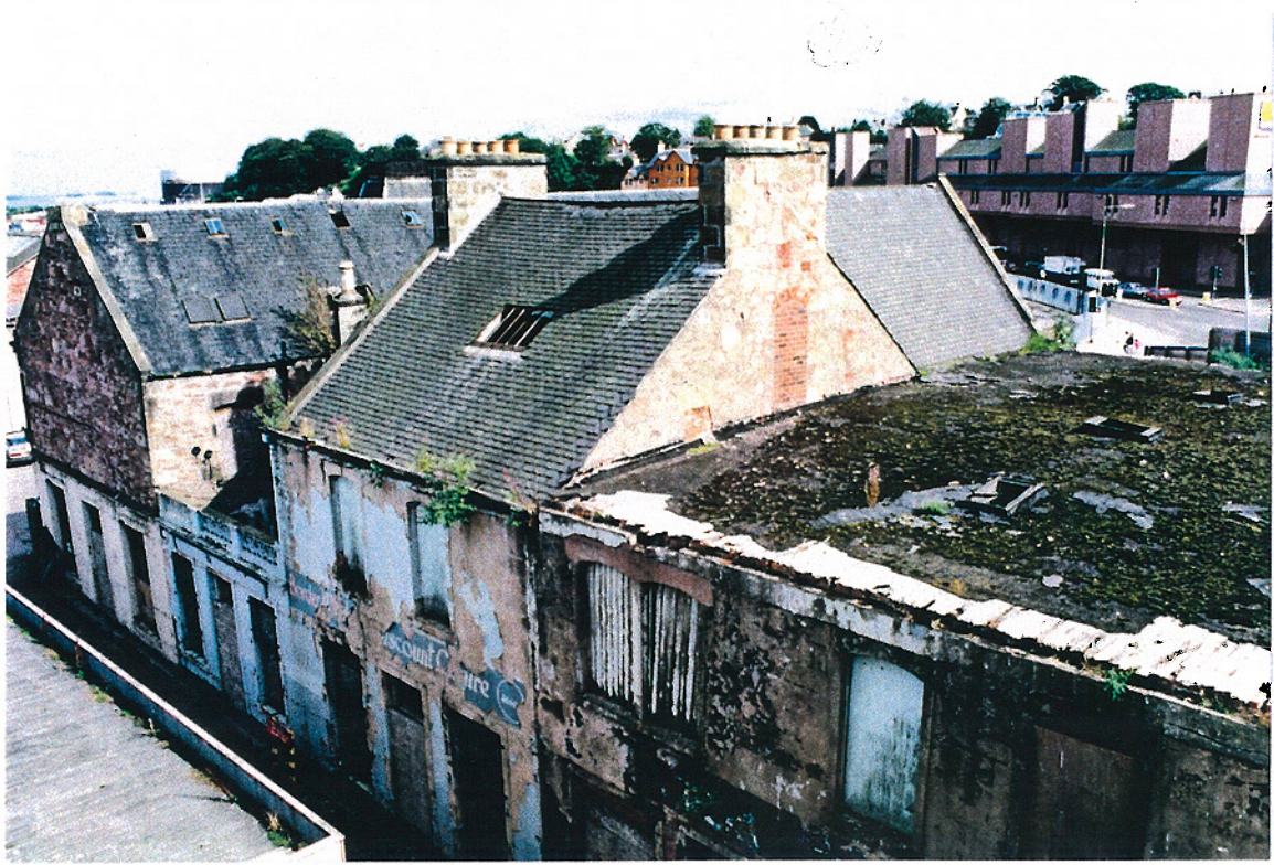
Buildings 2 and 3, north facing wall
