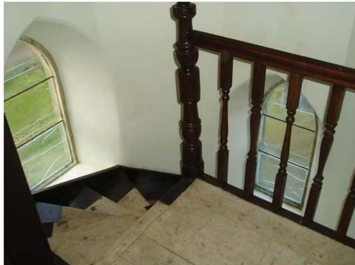
20 - stairs in NW tower showing windows W5 and W6
