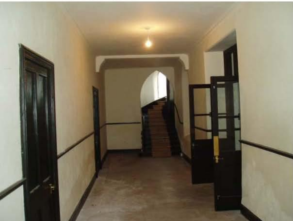
19 - looking S along the vestibule, porch doors D1 on the right
