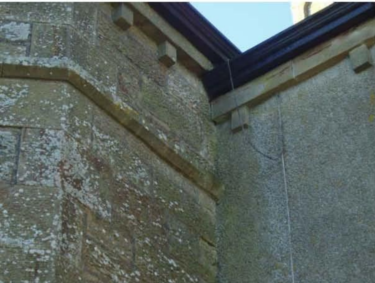
7 - join between upper SW tower and S wall
