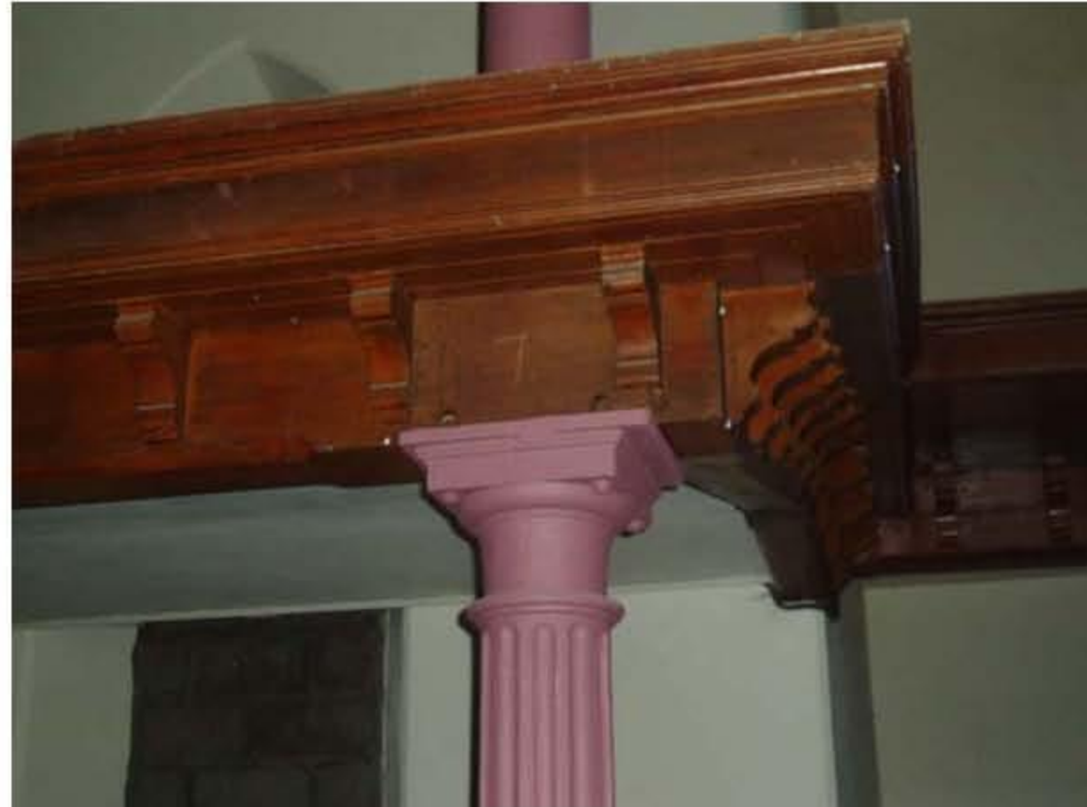
14 - detail of capital of column LP1 and corner of balcony
