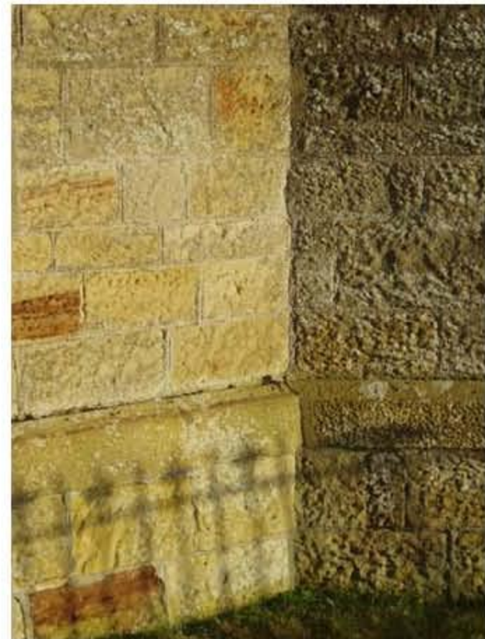
8 - join at base of SW tower
