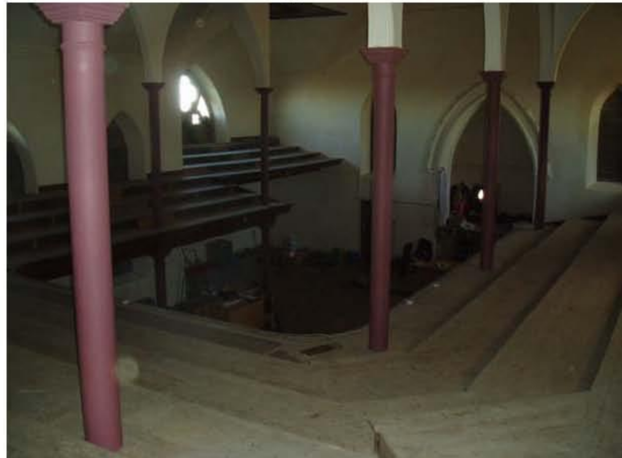
22 - view from SW corner of upper balcony
