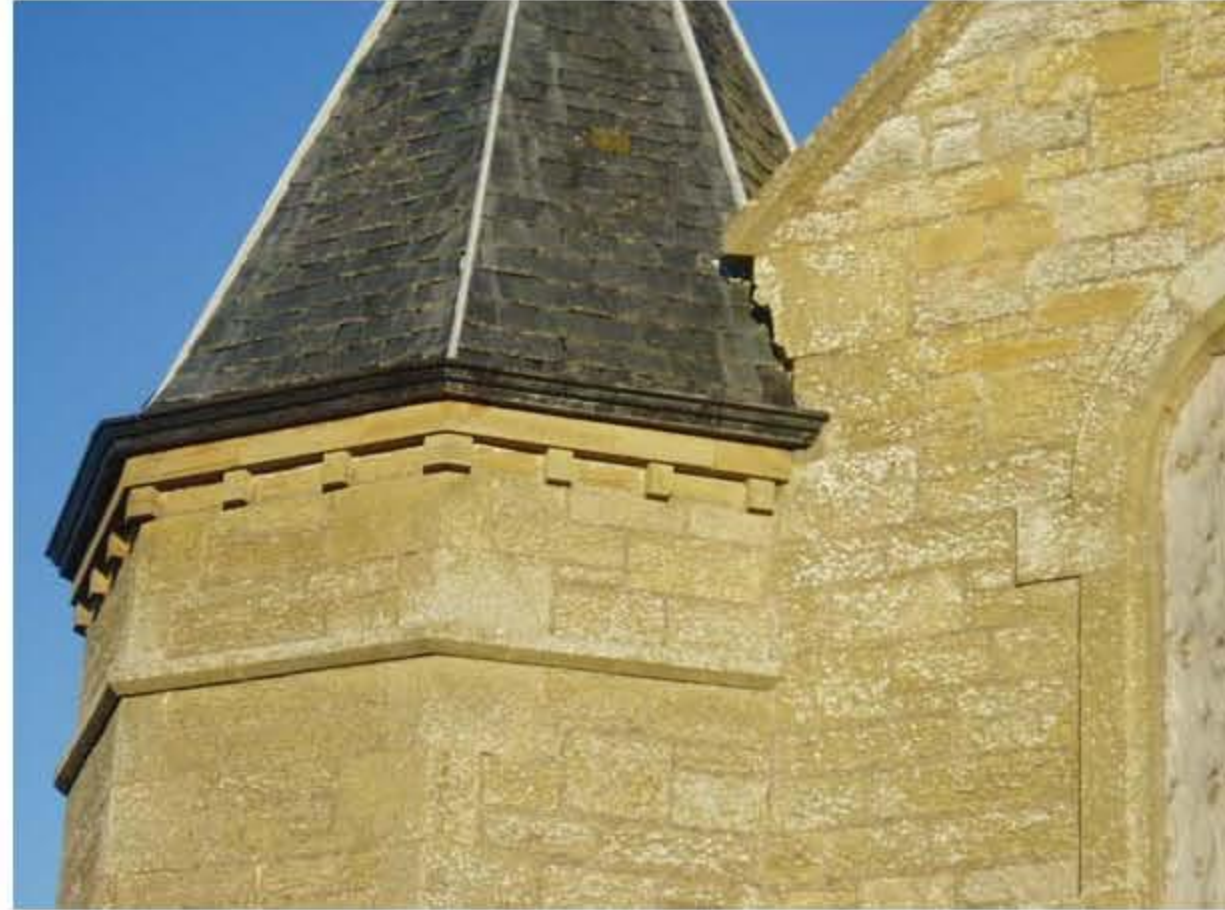
6 - join between upper NW tower and W gable roof line
