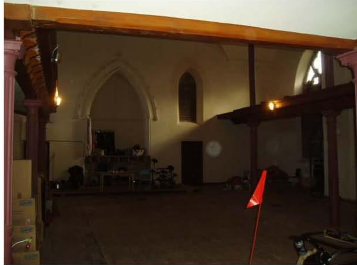
18 - looking E along the nave
