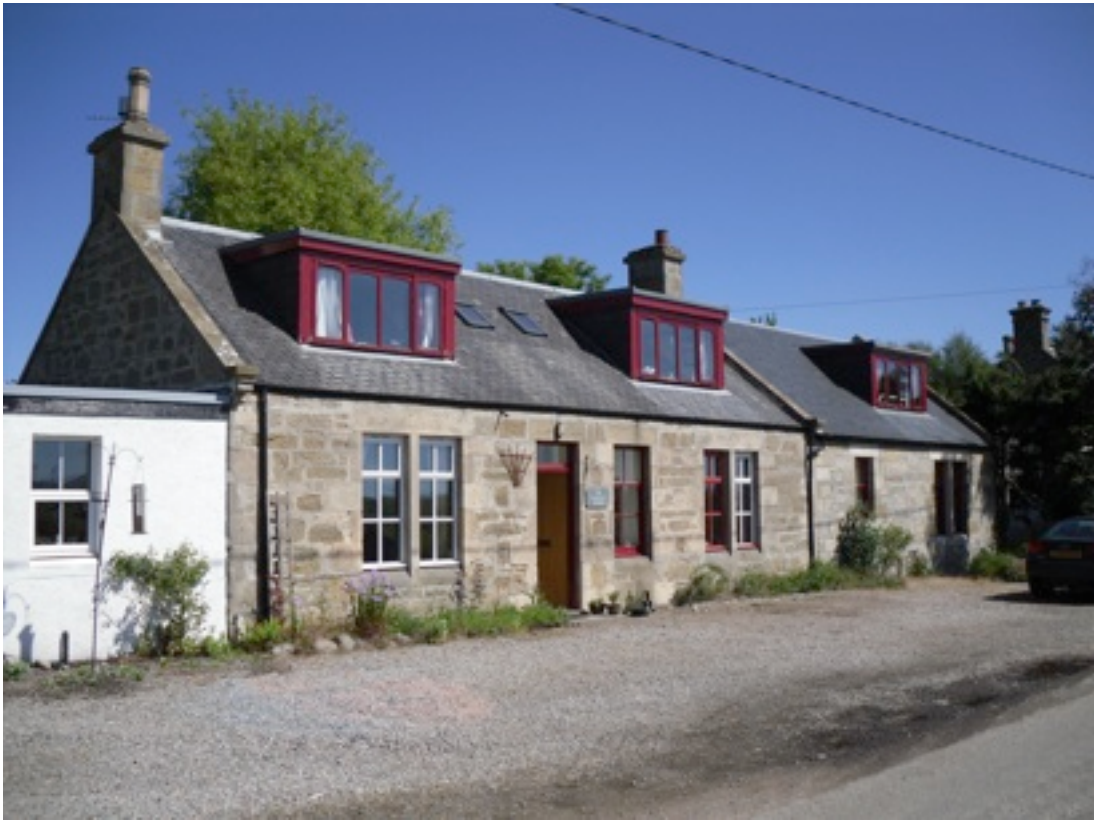
Photo 1 showing front elevation and parking area.
