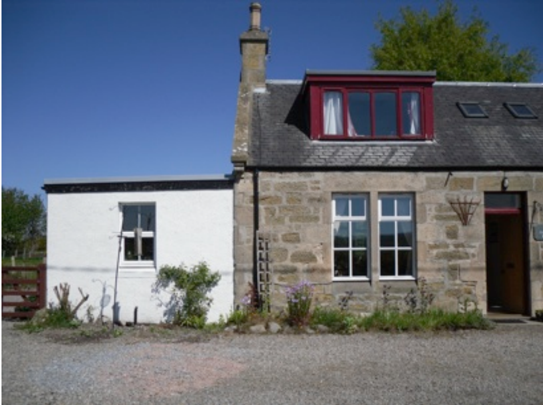
Photo 3 Showing modern blockwork extension housing the kitchen (formerly the garage).
