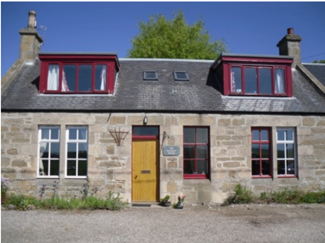
Photo 2 showing front elevation of the original part of the building.
