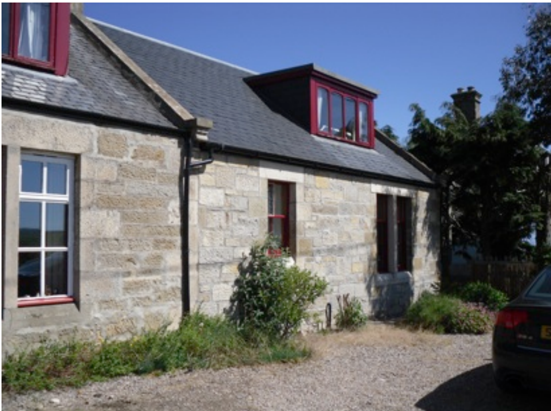
Photo 4 Showing modern stone & block cavity wall extension housing three bedrooms, bathroom, utility and study, constructed in 1999.
