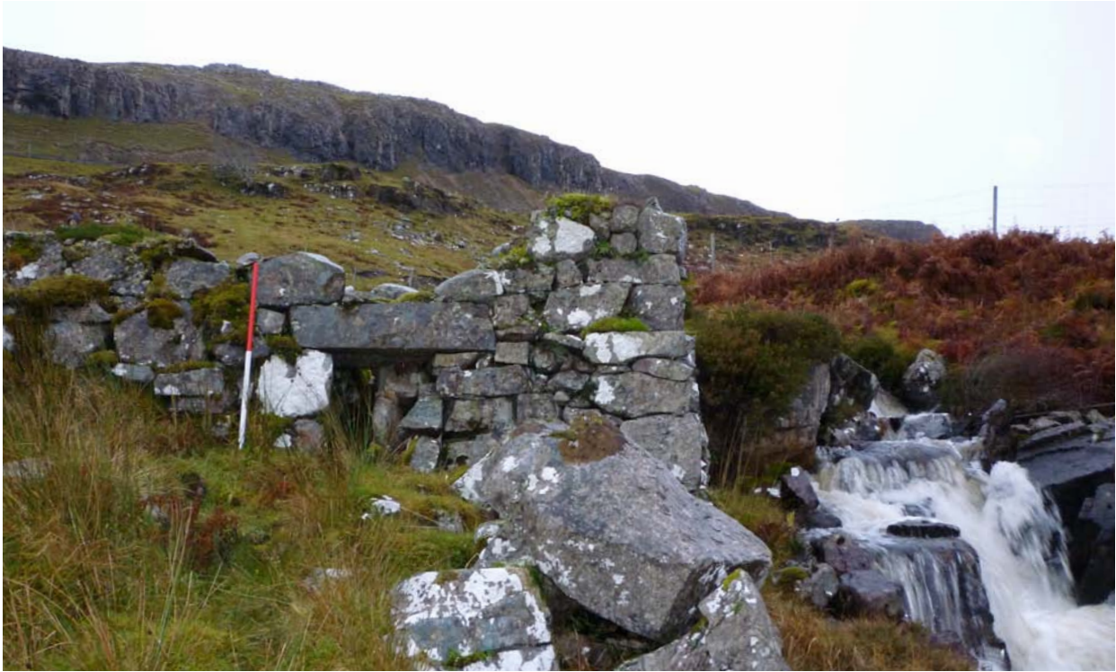
HLP 107, mill building, C.
