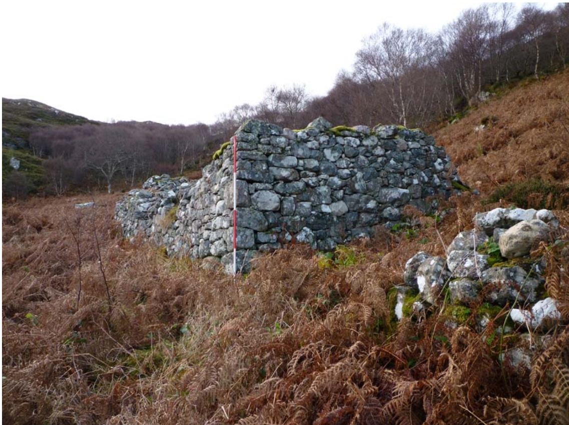
HLP 80, structure B.
