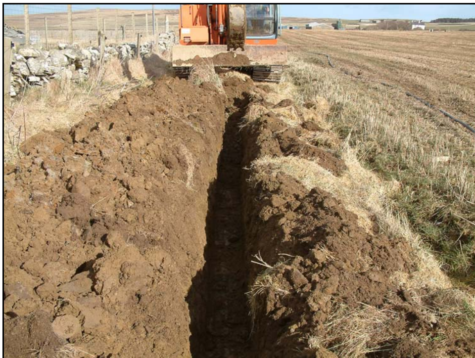
Plate 5 Cable trench excavation
