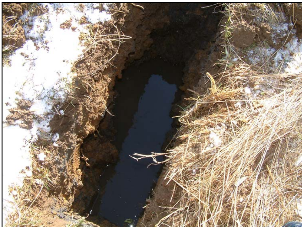
Plate 4 Pole excavation detail
