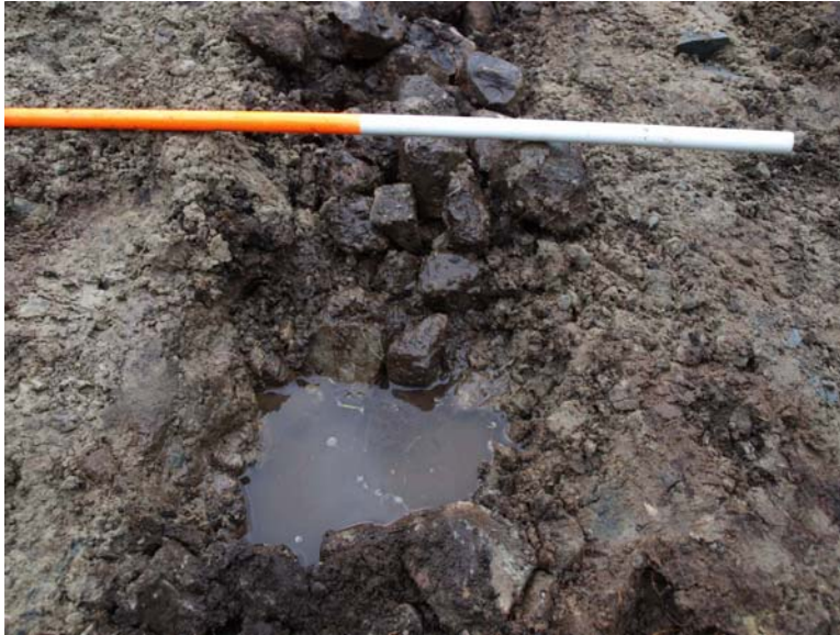
Figure 5 Section across the French drain
