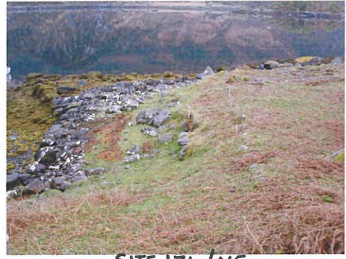
SITE 171/NE 2004_0424Image0045.JPG GENERAL VIEW OF REVETMENT
