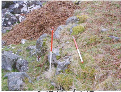
SITE 171/ENE 2004_0424Image0044.JPG DETAIL OF REVETMENT
