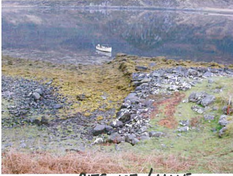
SITE 107/NNE 2004_0424Image0046.JPG GENERAL VIEW OF PIER
