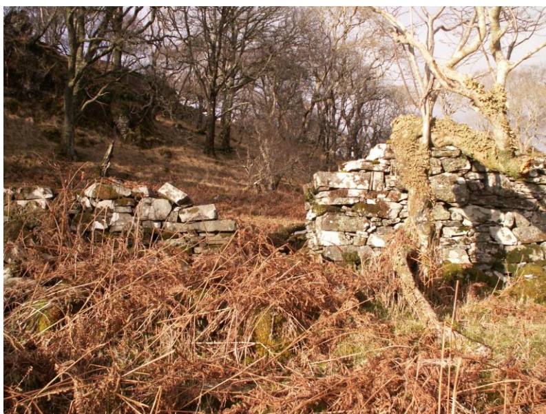
Rough joint of two halves of the building
