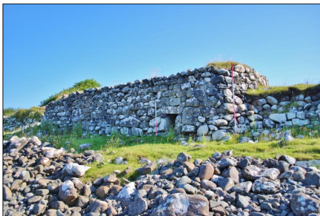
Plate 4 - Site A3 (facing SE), showing one drain
