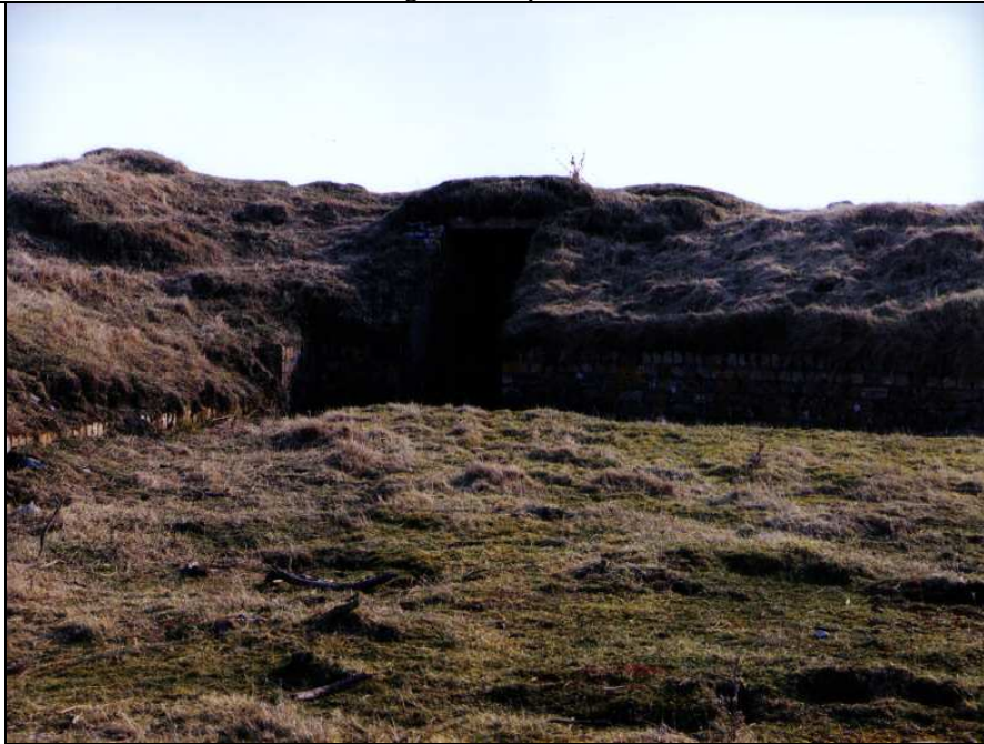
Photograph B28 showing entrance to underground shelter
