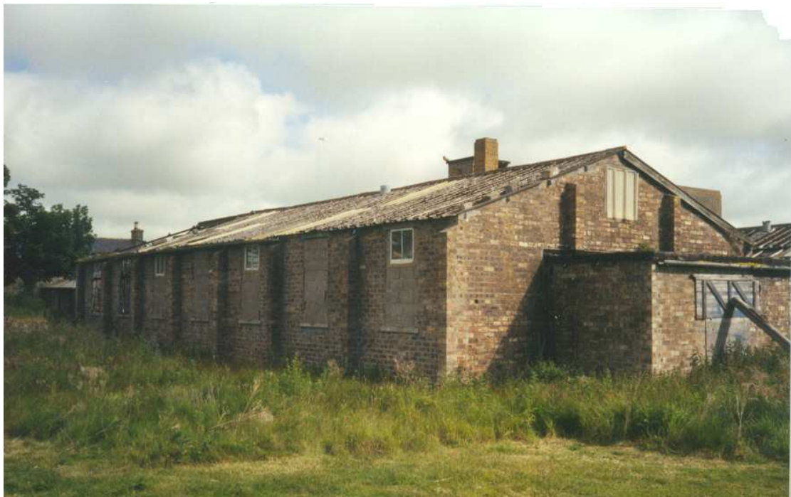
Photo No 18 Hospital Building NH8570 7705 View of western block from the S.W.
