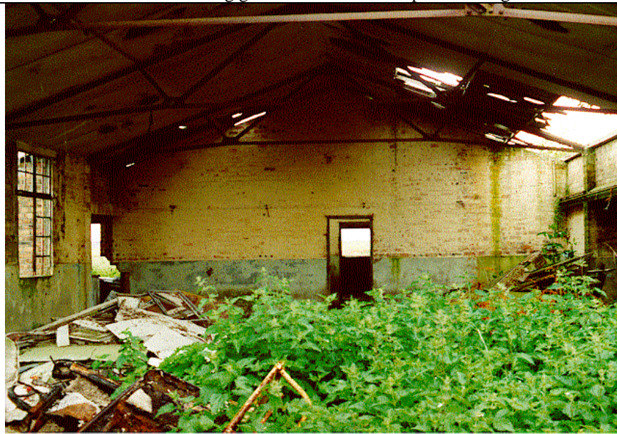
Photograph W51: internal view of hospital block
