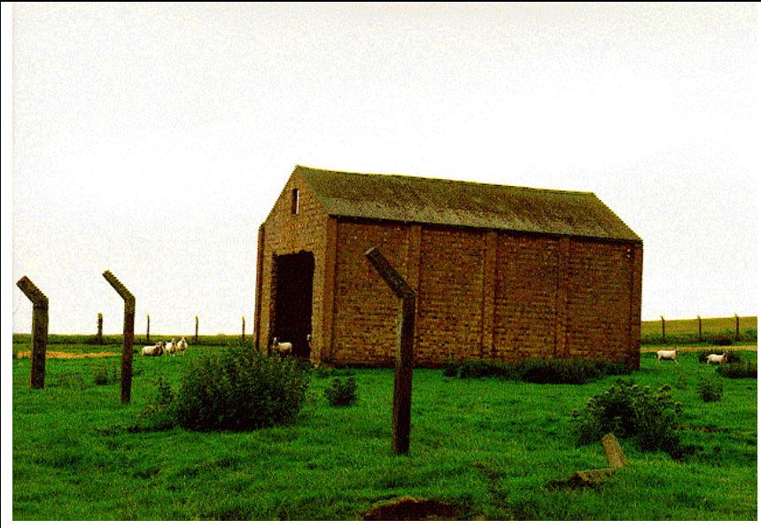
Photograph J6: fire engine building view from north west
