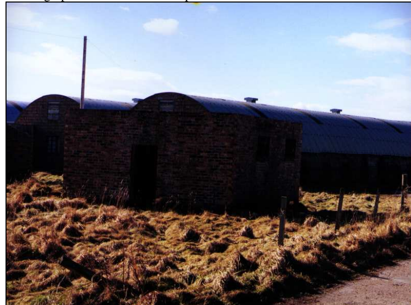
Photograph A12: Torpedo shed from access road
