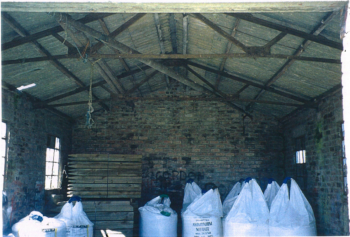
Photograph No. 33C Looking NW at roof of Building C.1
