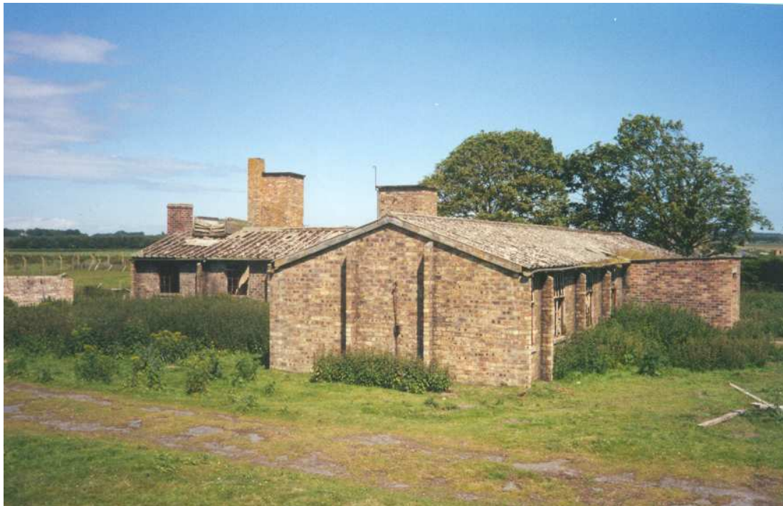
Photo No 26 Officers Mess (East) NH 8564 7708 General view from the S.W.
