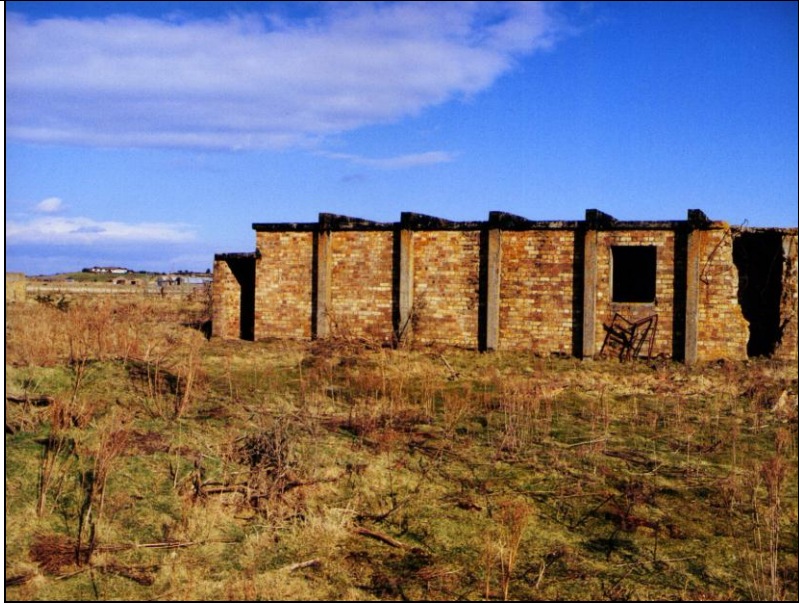
Photograph B35 munitions store
