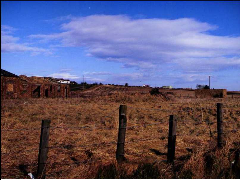
Photograph A20: view of technical building from the west FEARN AIRFIELD – PHOTOGRAPHIC SURVEY AREA A/G
