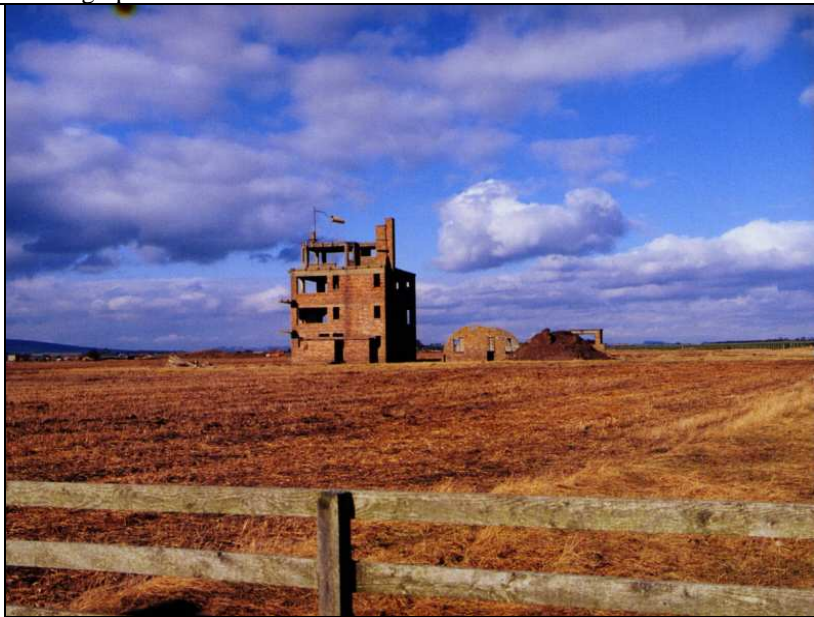
Photograph A8: Control Tower west elevation
