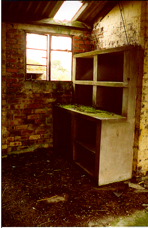
Photograph W47: interior view of store showing concrete shelving
