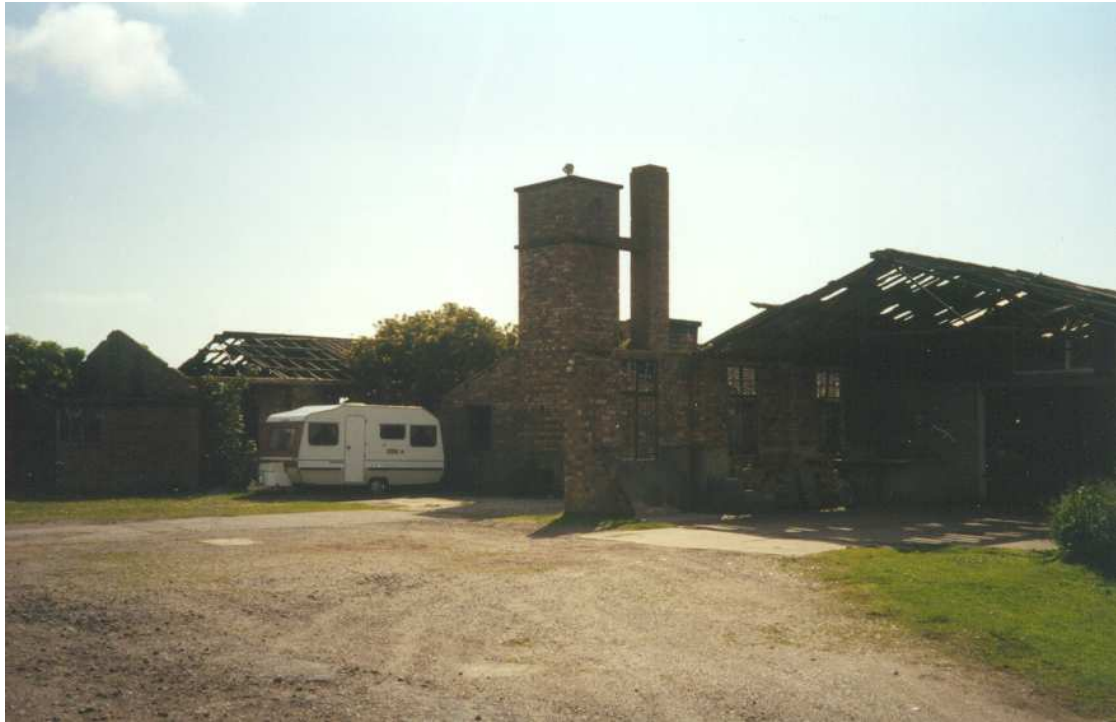
Photo No. 17 Hospital Building NH 8570 7705 View of front elevation facing N.W.
