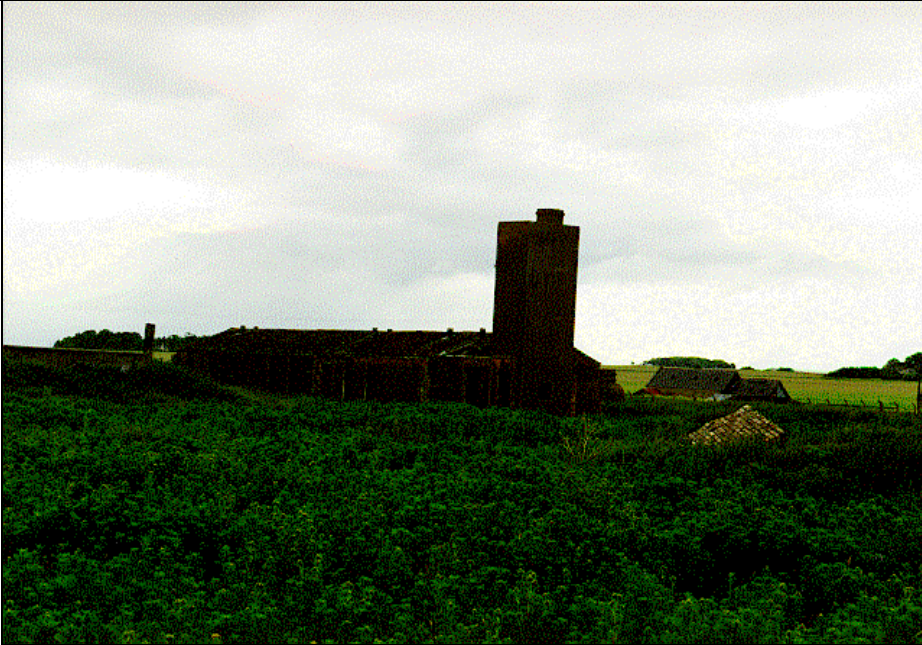
Photograph H12: building on eastern portion of the Wrennery site
