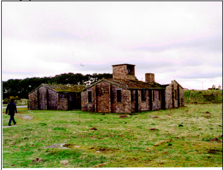
Photograph W24: officers mess north and east elevations FEARN AIRFIELD – PHOTOGRAPHIC SURVEY AREA H
