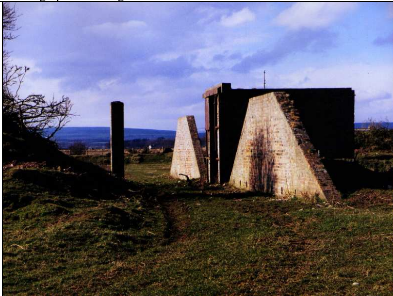
Photograph D42: bomb store with soil removed from behind blast walls FEARN AIRFIELD – PHOTOGRAPHIC SURVEY AREA D
