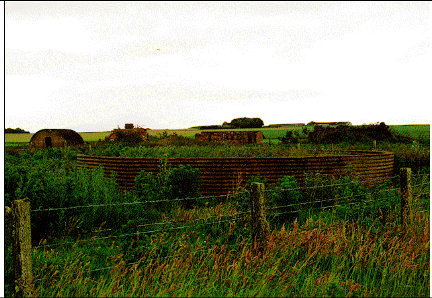
Photograph H8: watertank, the Wrennery
