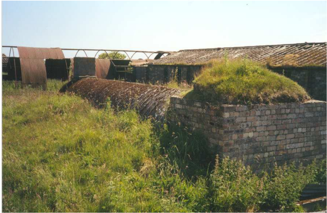
Photo No 25 Air Raid Shelter NH 8565 7695 View from the N.W.
