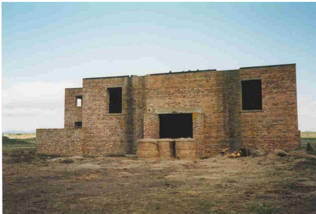
Photograph 9 Engine Test House – view from south west
