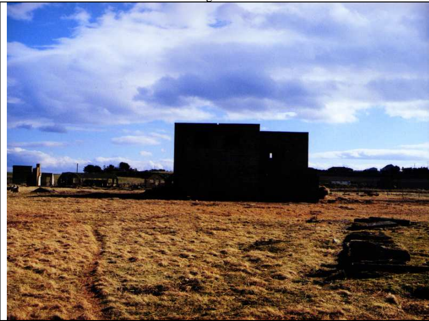
Photograph B34 showing engine test house
