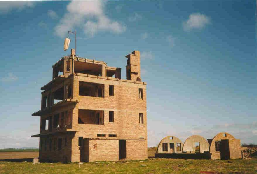
Photo 2 Control Tower viewed from the south
