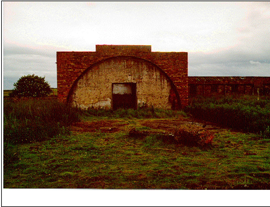
Photograph W44: Brick gable end to former nissen hut
