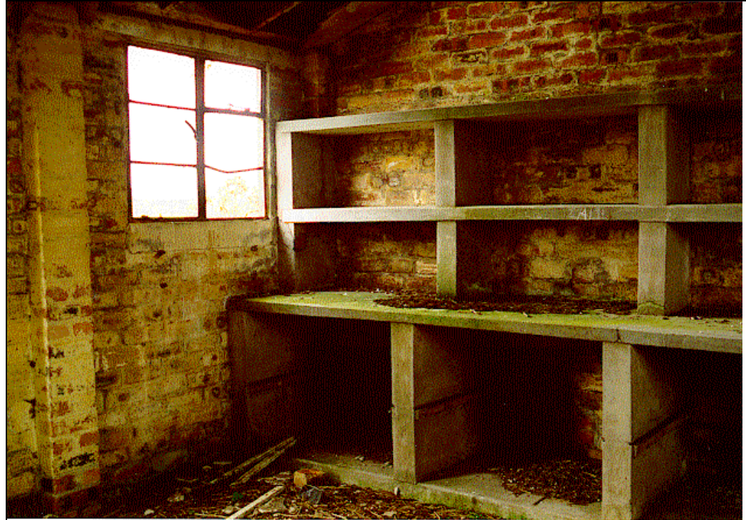
Photograph W48: interior view of store showing concrete shelving
