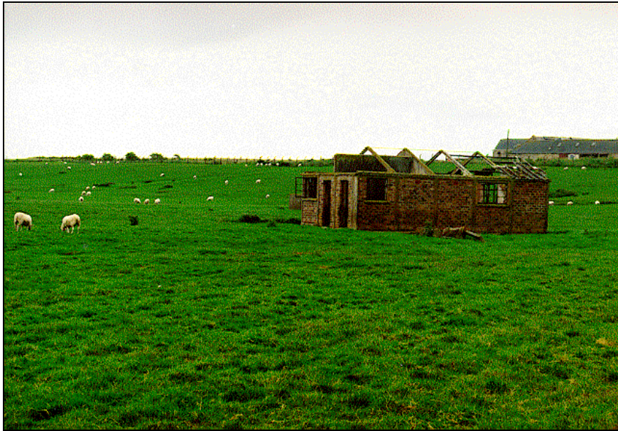
Photograph J20: building opposite stores
