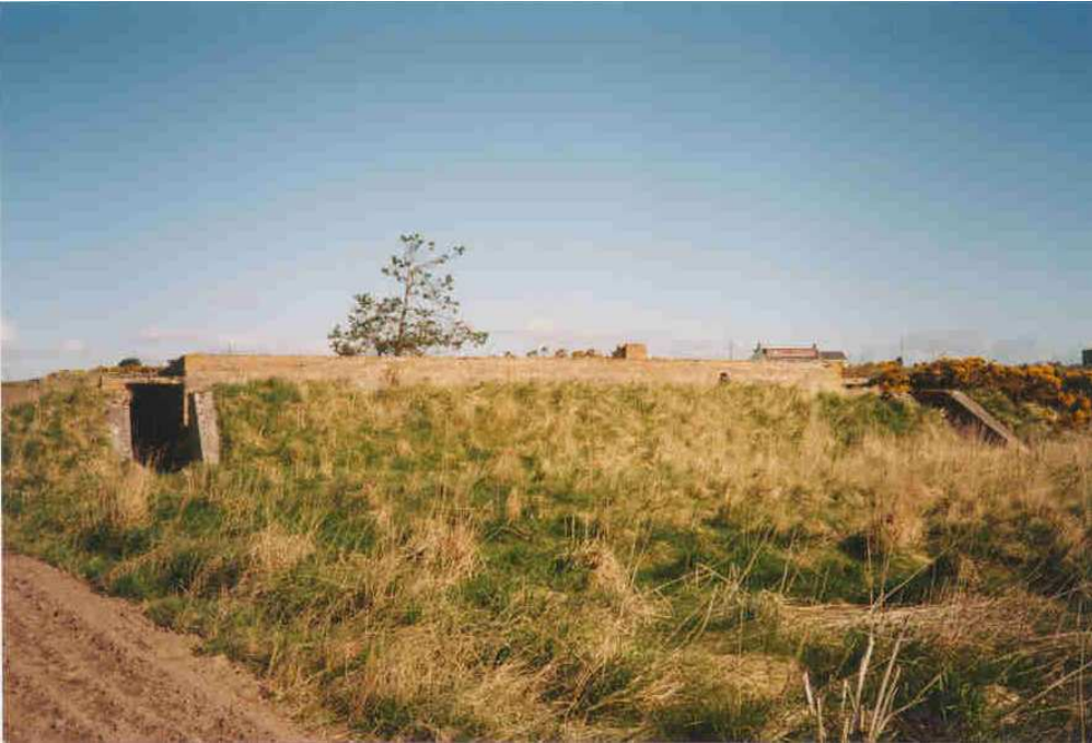
Photo 1 Operations block viewed from the south
