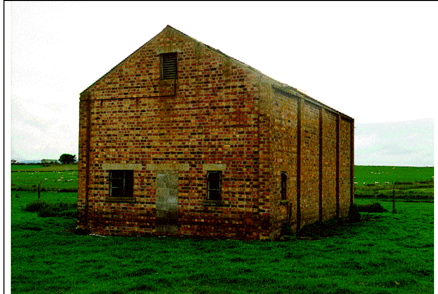
Photograph J7: fire engine building view from north west
