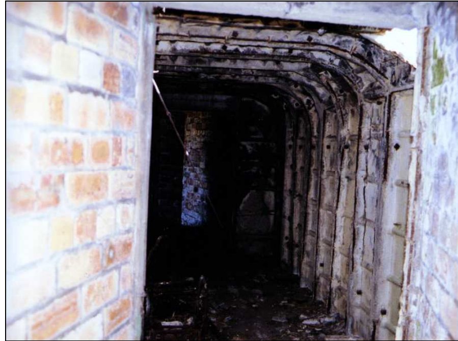
Photograph B29 showing interior of underground shelter
