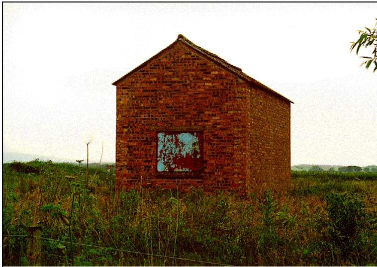
Photograph C41: northern gable of fire engine garage
