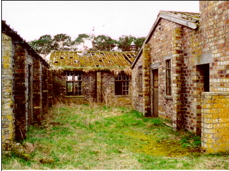
Photograph W10: cookhouse and dining area east elevation
