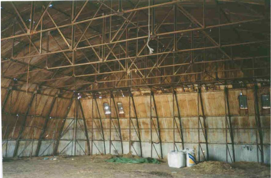
Photograph 12 Hangar NH 840 751- interior
