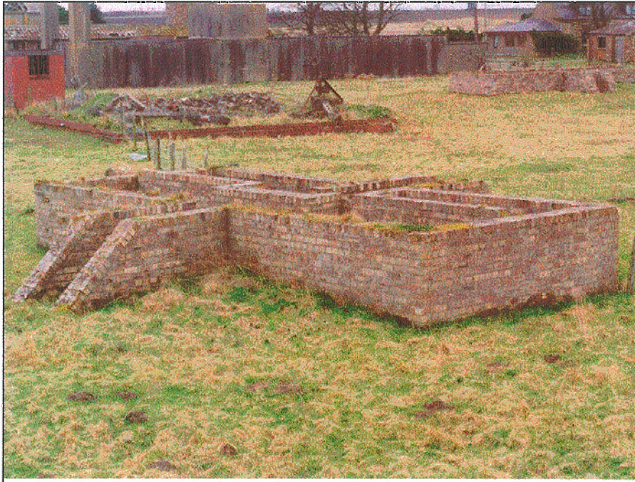
Photograph W5: air raid enclosure
