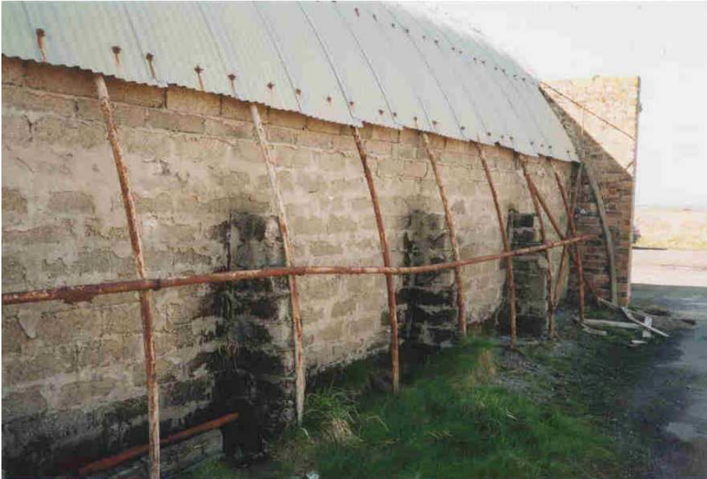
Photo 6 Torpedo sheds exposed framework on north wall and non original blockwork walls
