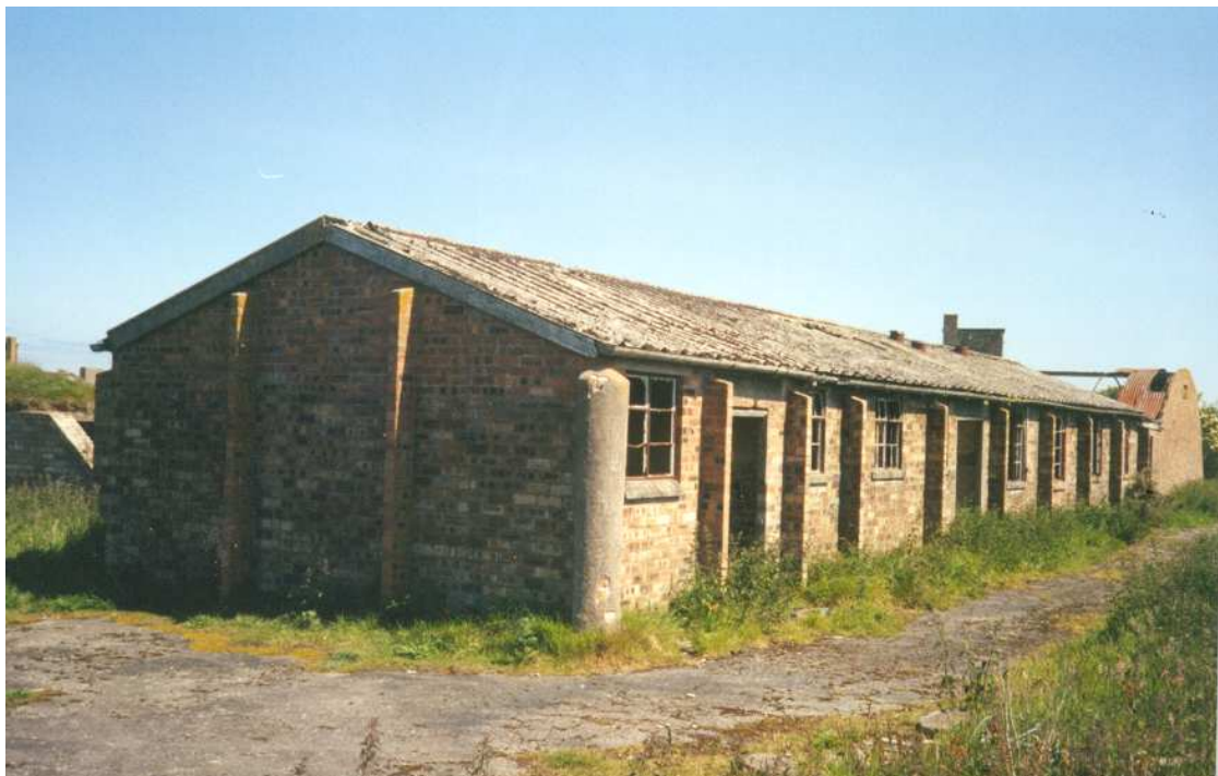
Photo No 22 Stores Building NH 8568 7694 West gable and south elevation
