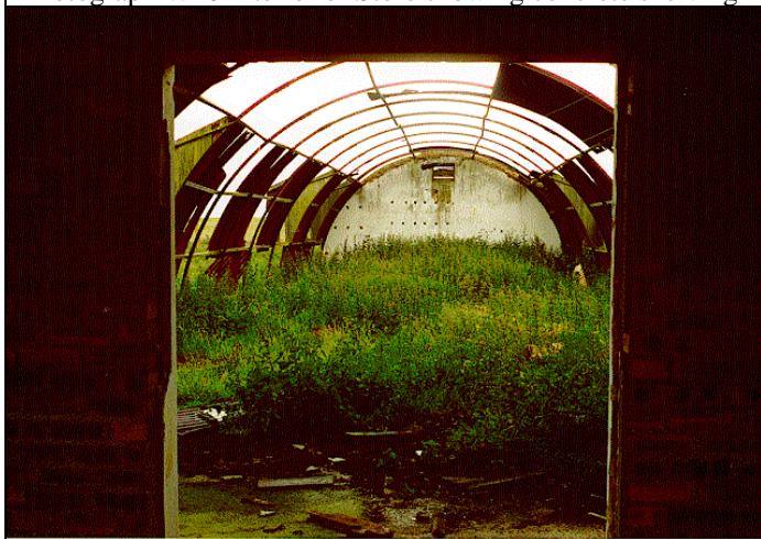
Photograph W45: interior view of nissen structure
