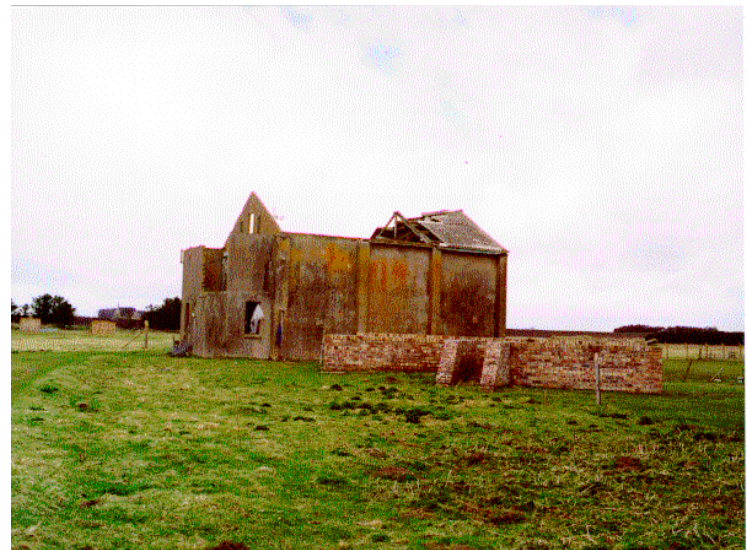
Photograph W21: cinema west and south elevations
