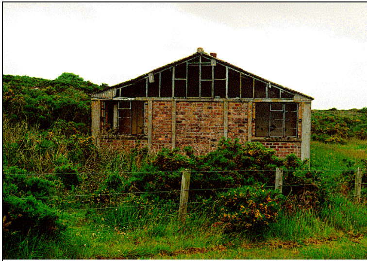
Photograph J13: stores building – east elevation
