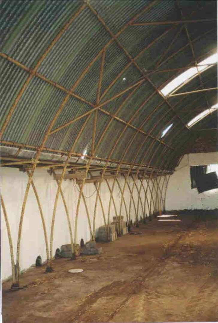
Photo 5 Torpedo sheds interior showing valley gutter
