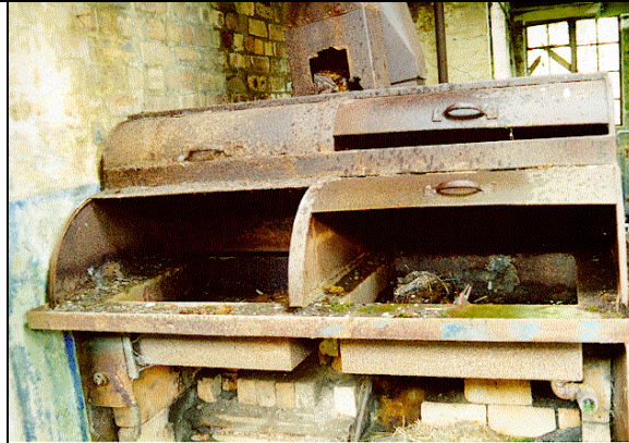
W57: Interior view in hospital block
