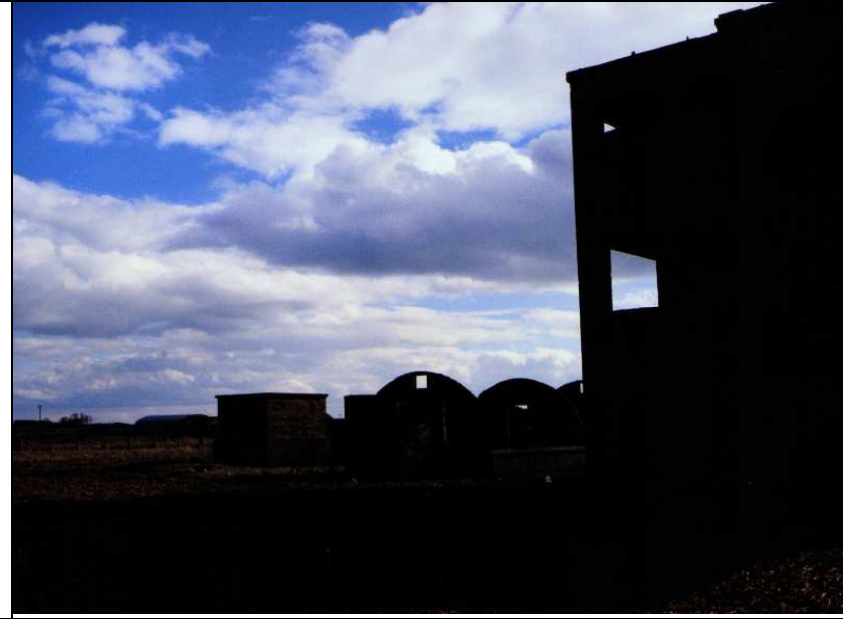
Photograph A7: buildings adjacent to Control Tower – north elevation
