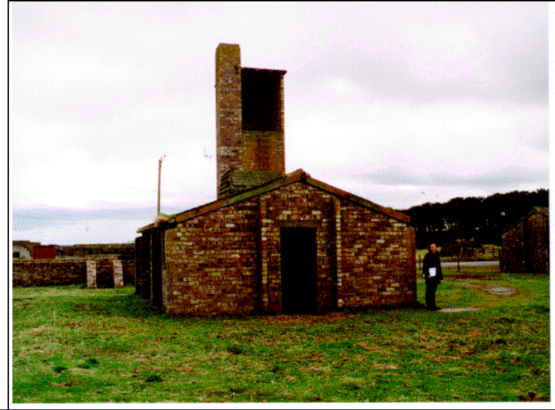
Photograph W23: ablutions block north elevation
