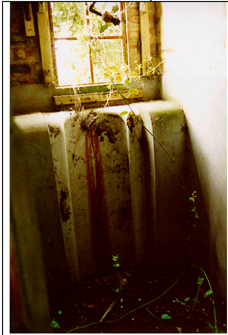
W59: interior view of hospital block
