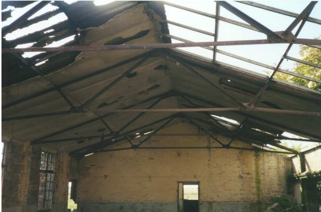
Photo No 19 Hospital Building NH 8570 7705 Typical 28'0" span roof construction
