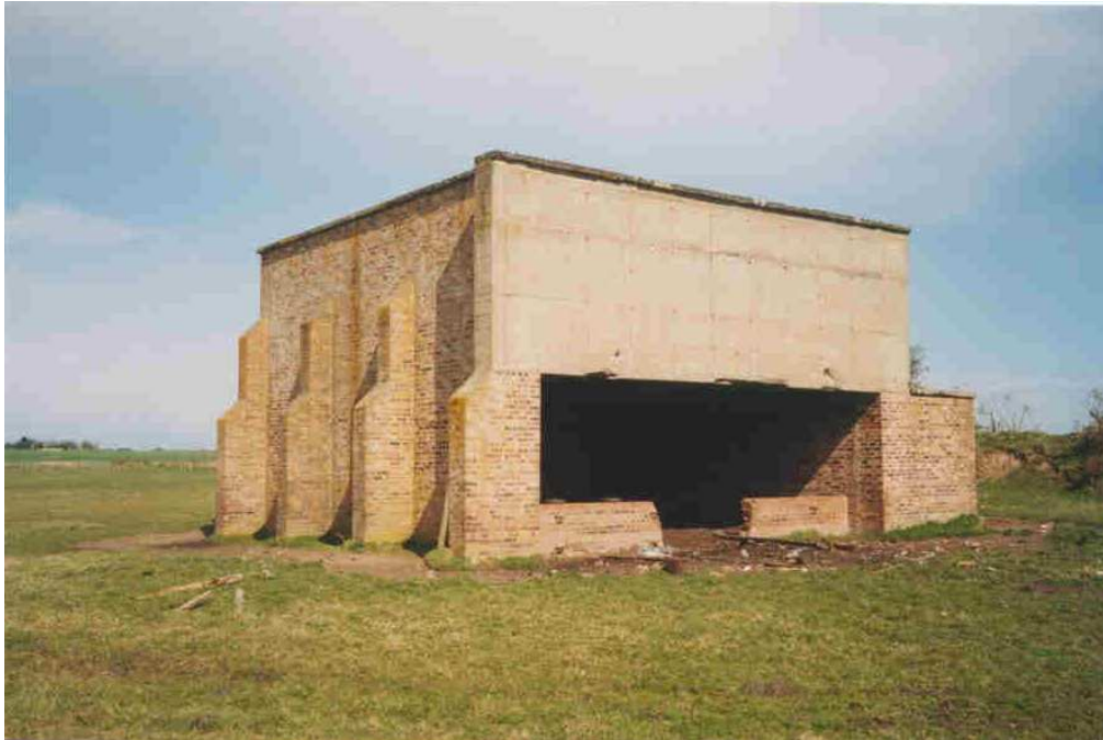
Photograph 16 Stop Butt - view from south west
