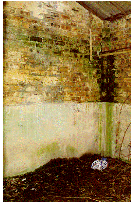
W60: interior view of hospital block
