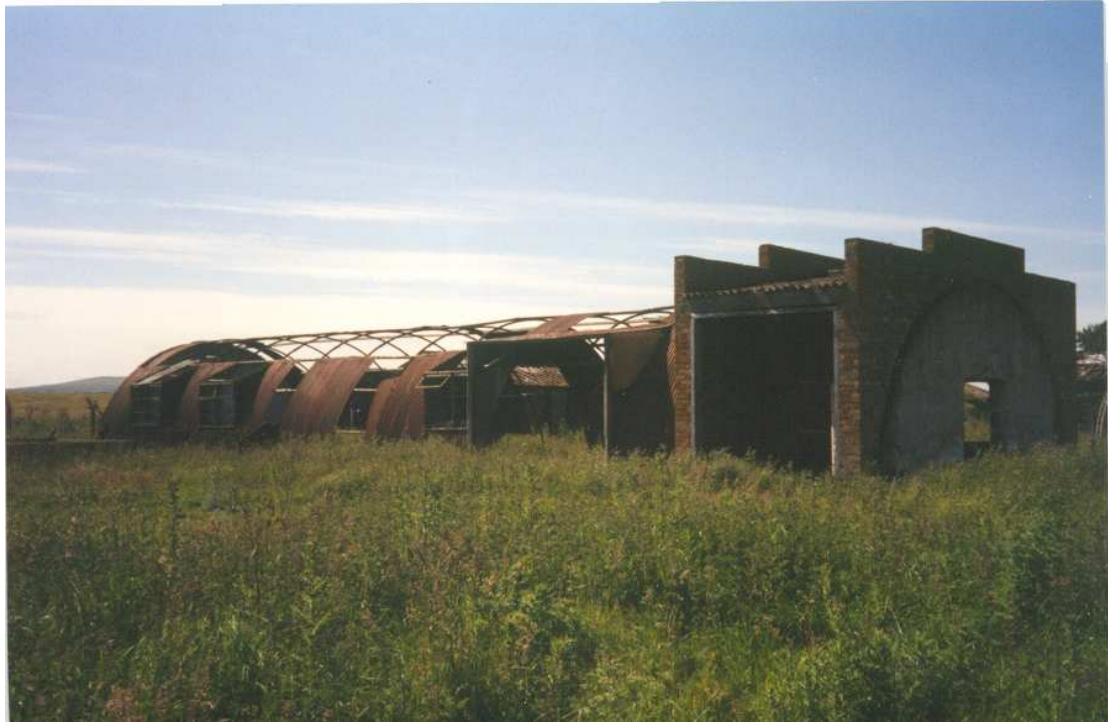
Photo No 23 Stores/Workshop Building NH 8568 7694 Nissen Hut section viewed from the N.E.
