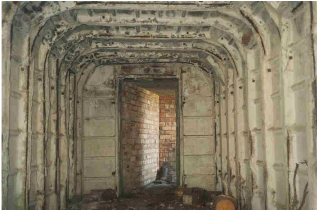
Photograph 8 Underground shelter - interior
