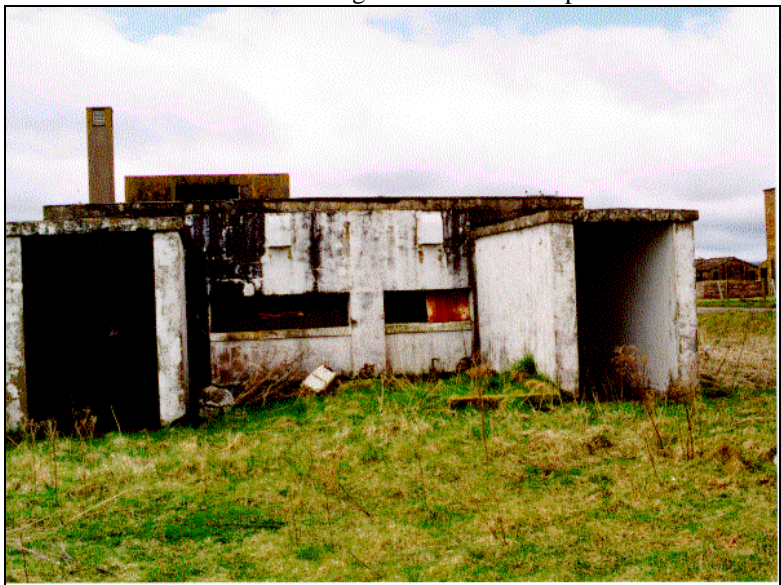
Photograph W16: Decontamination Centre east elevation
