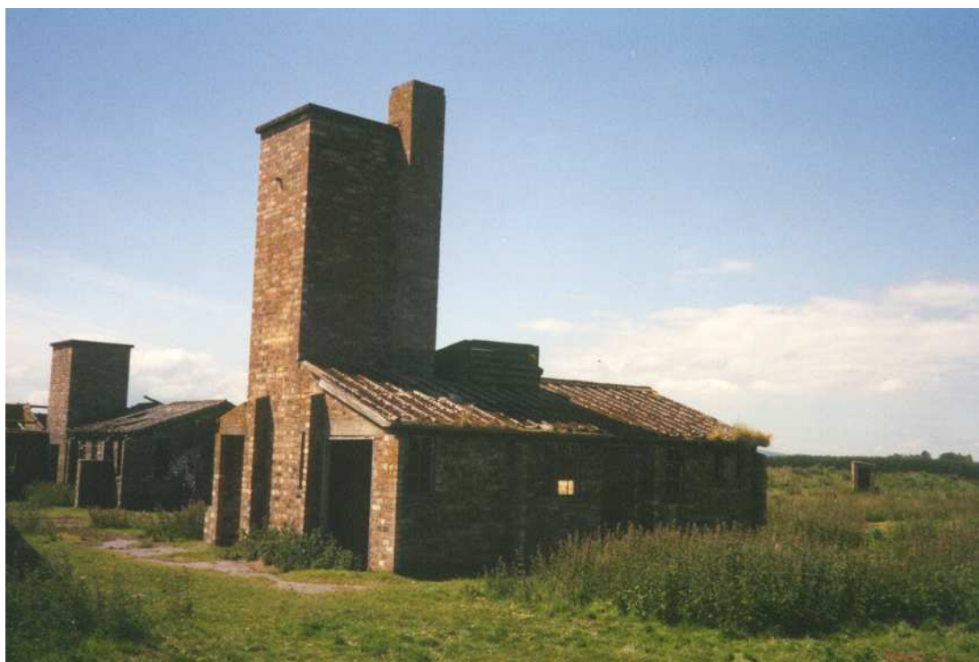
Photo No 31 Ablutions Block NH 8560 7707
