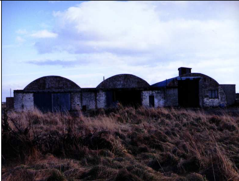
Photograph A9: Torpedo shed west elevation
