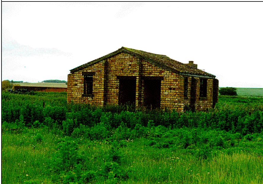
Photograph H4: building close western side of eastern portion of Wrennery FEARN AIRFIELD – PHOTOGRAPHIC SURVEY AREA H
