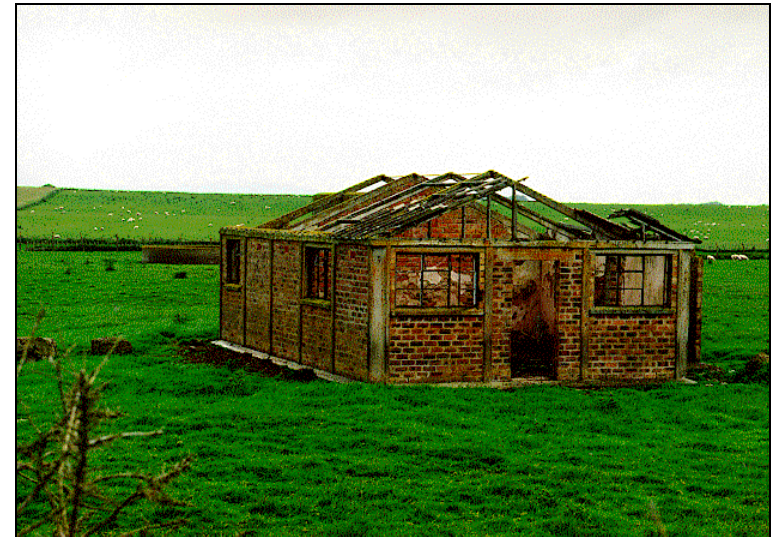
Photograph J14: building opposite stores
