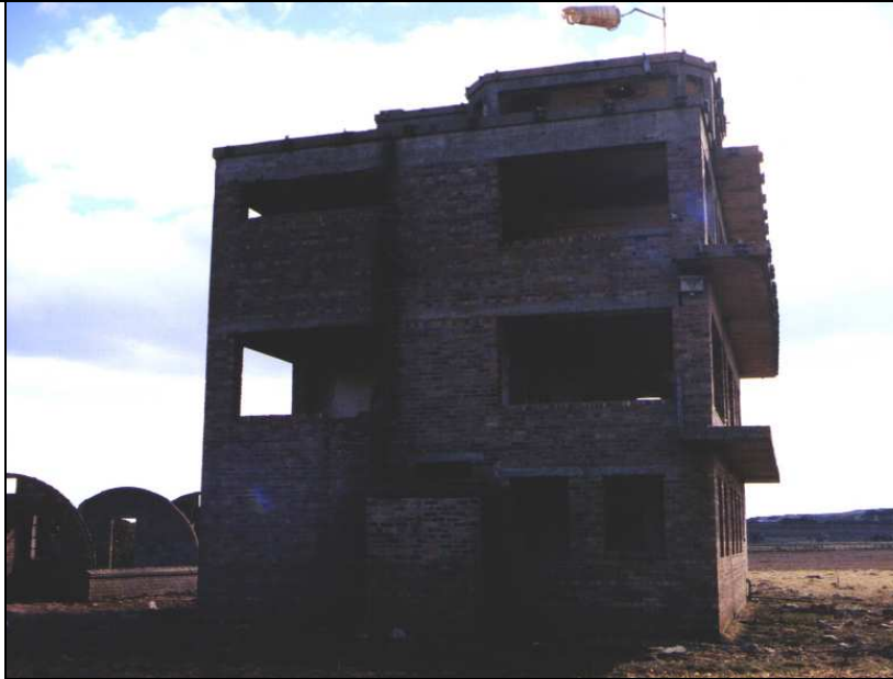
Photograph A6: Control Tower: north elevation
