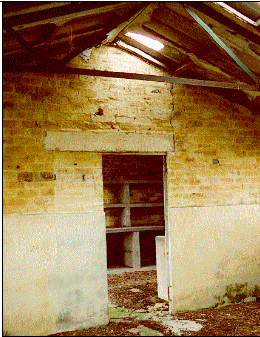
Photograph W40 Interior of Store showing concrete shelving
