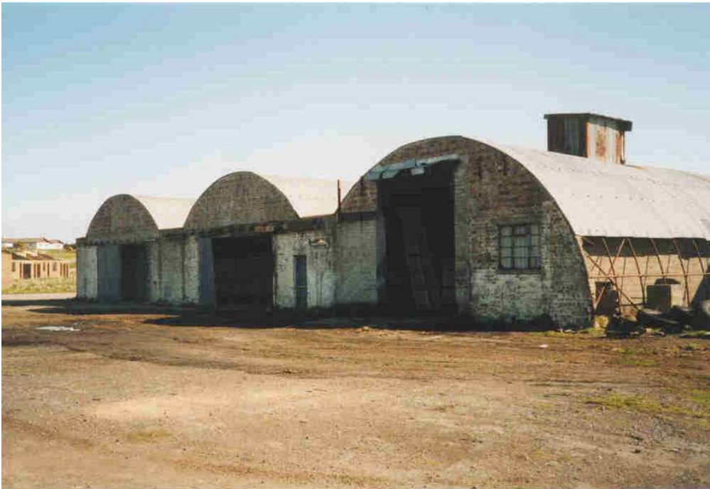
Photo 4 Torpedo sheds viewed from the south
