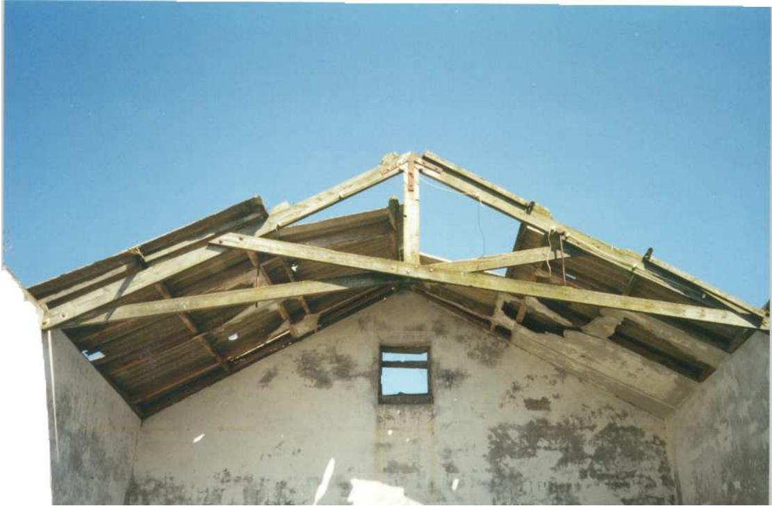
Photo No 29 Cinema Building NH 8562 7711 Roof Construction
