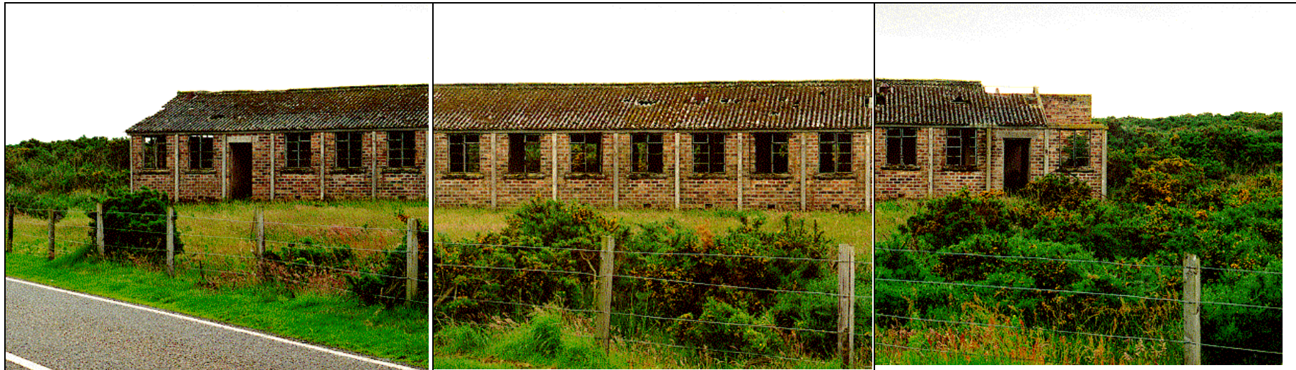
Panorama J8/J9/J10: stores building northern elevation
