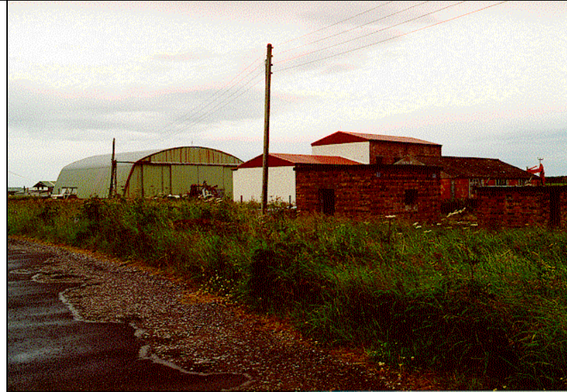
Photograph A23: hangar in use
