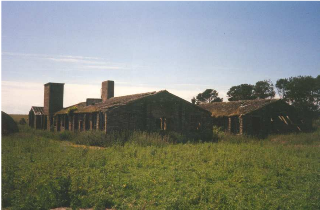
Photo No 21 Canteen Building NH 8563 7694 General view from the north
