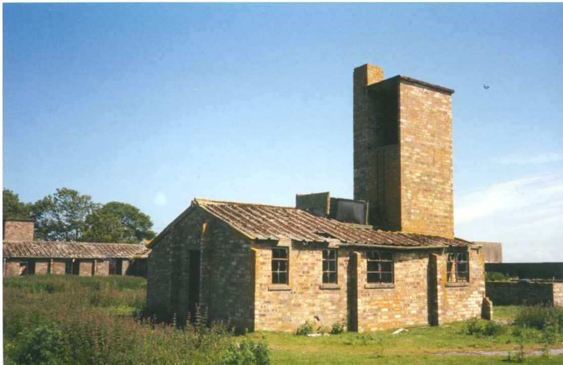
Photo No 30 Ablutions Block NH 8560 7707 View from the West
