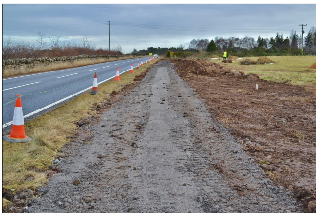
Plate 1 Culloden Footpath on 8 Feb 2013, facing E
