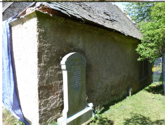
Fig 14 Overhanging trees are placing the mausoleum at risk on the east boundary; the photograph shows also further gravestones in this area which would need to be recorded and protected before works commence
