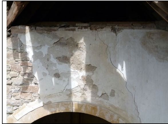
Fig 25 Cracking in the plaster finish above the arch leading into the north vault, resulting in the keystone dropping and movement in the voussoirs to the right of the opening; the collar tie beyond the head of the wall has snapped due to weakness caused by woodworm infestation
