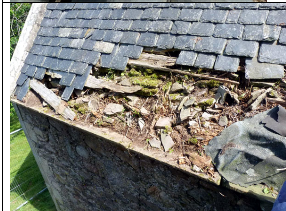
Fig 17 Extensive damage caused by loss of slates and sarking on the west side of the roof above the north vault: the condition of the rafter ends is uncertain, being covered in vegetation growth and debris trapped by the beamfilling and plaster and lath, but is bound to be poor, throwing the stability of the roof into question
