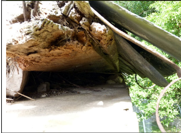
Fig 19 Photograph looking along the wallhead from the southeast corner, showing the wallplate (partially rotten with woodworm infestation) lifted clear from the stone tabling under the weight of the unsupported portion of the roof – this condition extends to as far as the internal wall to the north vault where the roof appears sound
