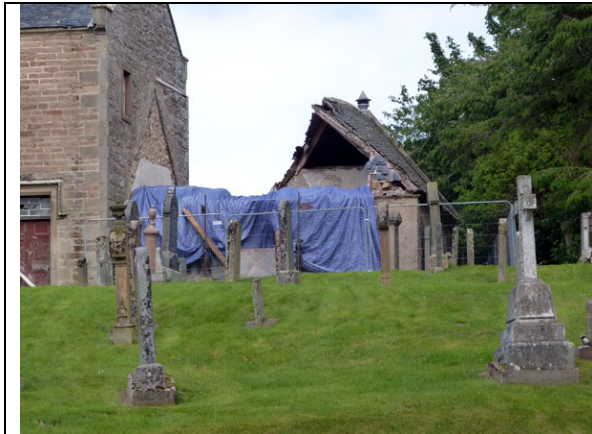
Fig 18 The unsupported part of the roof exposed after the collapse can be seen from the south, with the stone ridging dipping towards the unrestrained hip rafter
