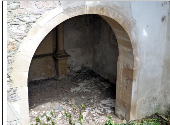
Fig 4 Wall monuments can be glimpsed through the arch at the entrance to the north vault on the north gable and east wall, of yellow sandstone and marble respectively; the panel to the right is believed to have been inserted in 1861 at which time the Venetian window would have been blocked up
