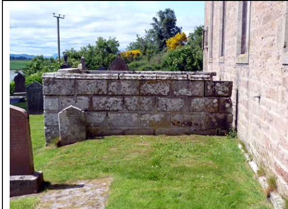
Fig 9 Family burial ground of c1700 of ashlar sandstone which became detached from the front wall of the church when it was rebuilt in the late 1830s
