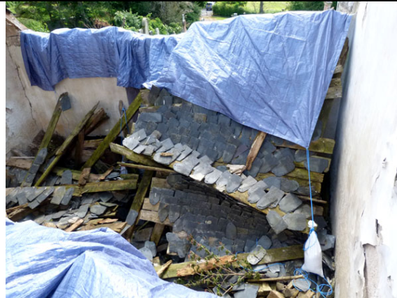
Fig 6 Interior of the mausoleum viewed from the north, showing collapsed sections of roofing with the sarking and slates still intact and the space littered with debris
