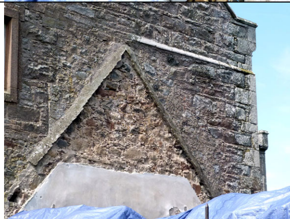
Fig 7 High level stringcourse above the roof ridge of the mausoleum at the east gable of the former church shows evidence a previous building on the site, possibly that of 1767
