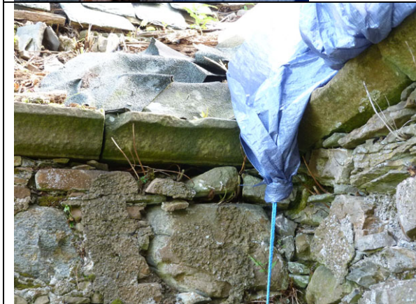
Fig 11 Internal junction between the late 17thc work and the mid-18thc extension to the north shows the differing patterns of wall tabling, from a plain chamfered stone in the earlier work to a more sophisticated cavetto moulding in the work of c1742; the rubble masonry has suffered from constant wetting from the base of the valley gutter and has open joints where the mortar has been lost
