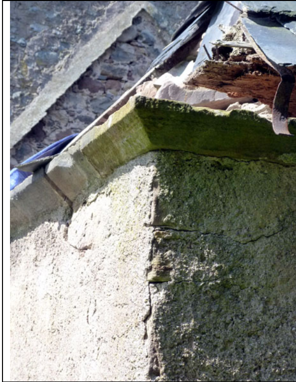
Fig 20 Detail of the wallhead at the southeast corner of the building, showing the wallplate lifted from the wall tabling course and rotation in the corner stone which has disturbed the harling, although this is thought to be unrelated to the roof collapse
