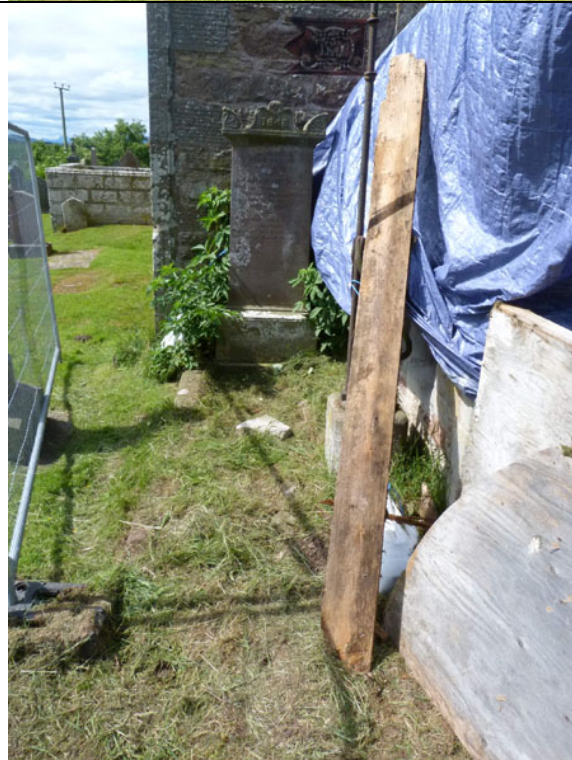
Fig 13 A burial lair with a stone kerb and headstone, dated 1848, is in close proximity to the south wall of the mausoleum and will require protection when erecting scaffolding
