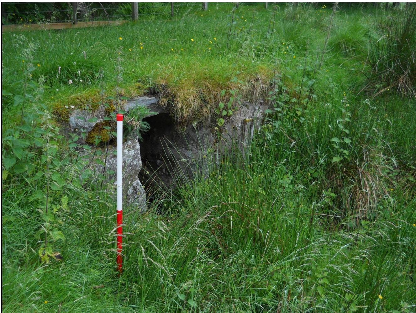
Plate 2 – Bridge Site 4 carrying access track Site 5
