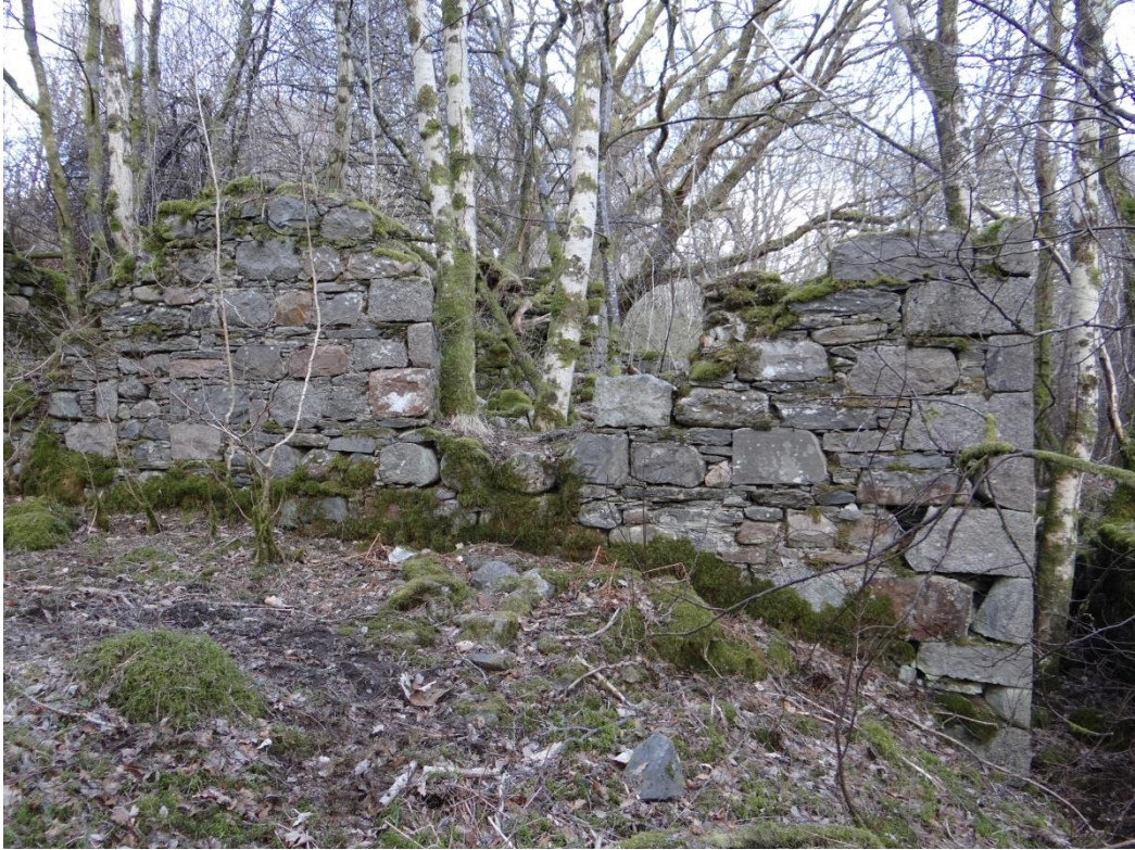
13 - Southern section of the western wall, viewed from the west facing east
