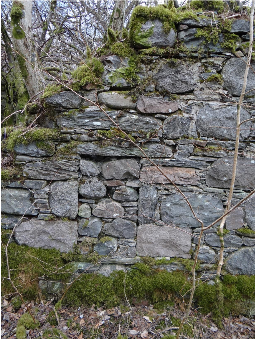
26 - Filled in window in the western wall of main building, facing east
