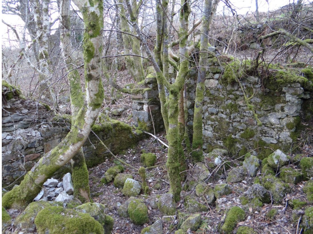
24 - Interior of the main room, facing north west taken from the south east corner
