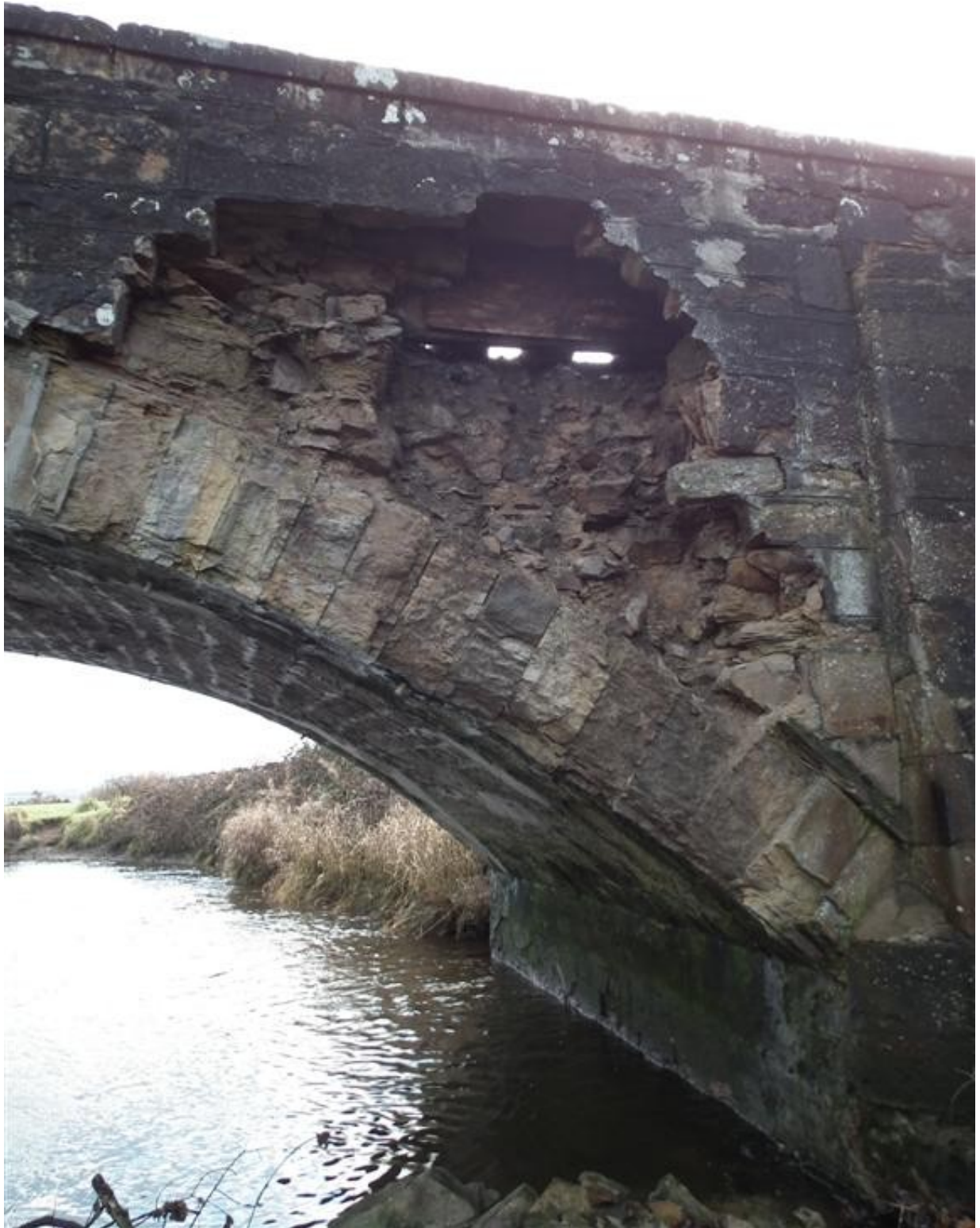
Damaged spandrel wall and arch voussoirs on upstream elevation
