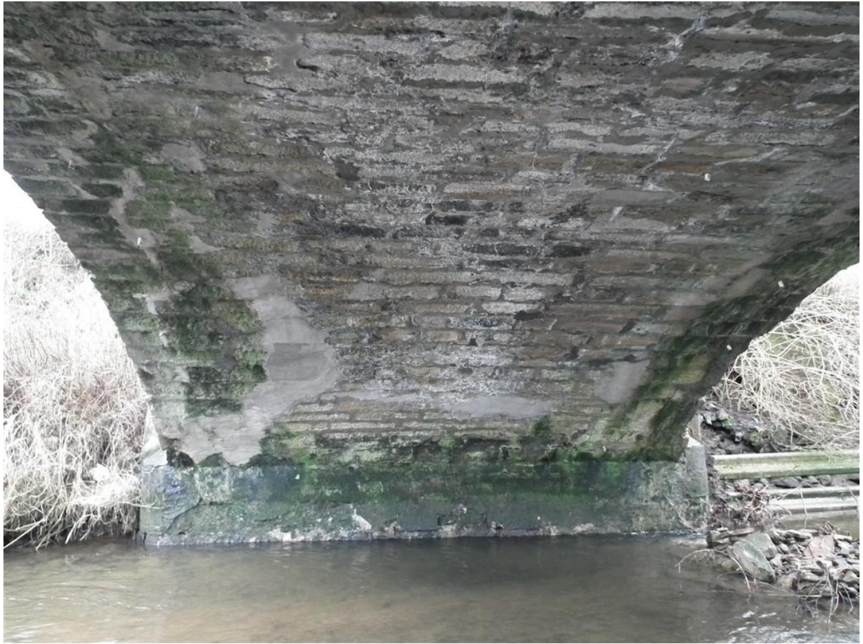
Arch with cement repairs evident and collapsed masonry in burn
