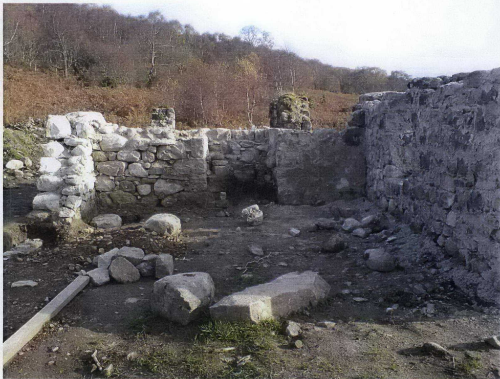
East Gable of Croft
