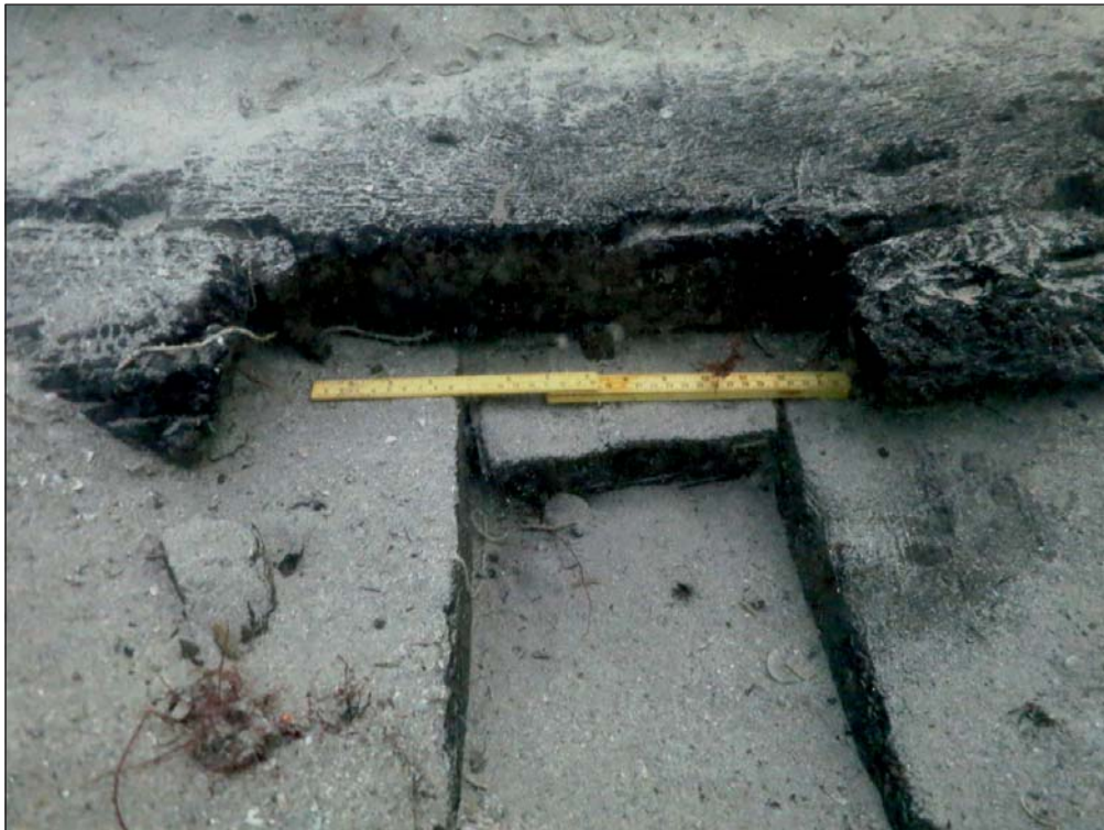
Plate 11: Section of timber framing
