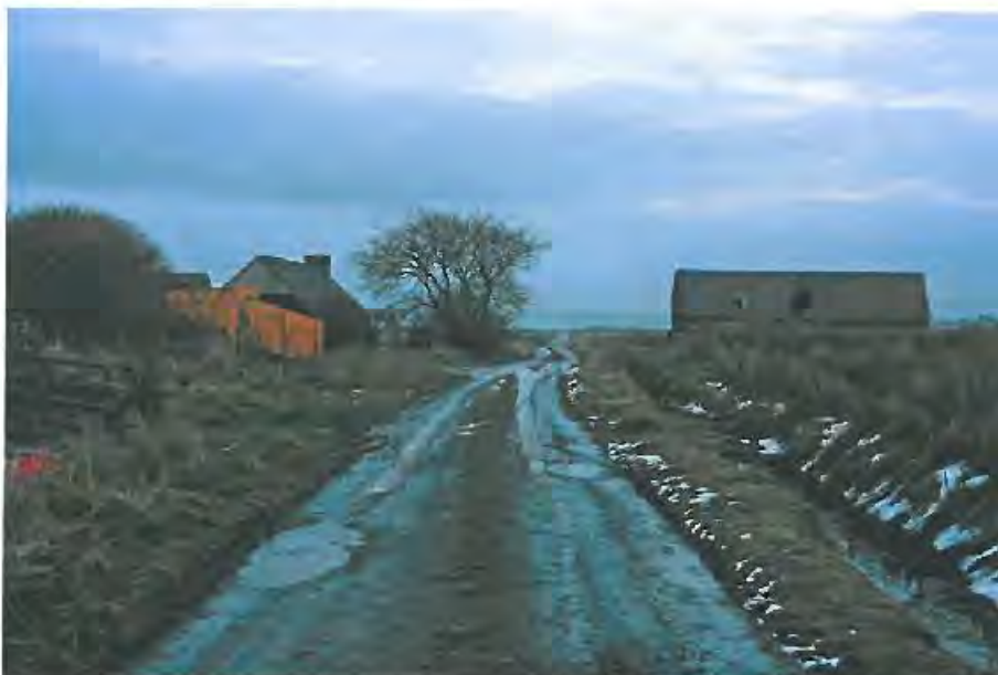
General view of buildings (Site 17) from SW
