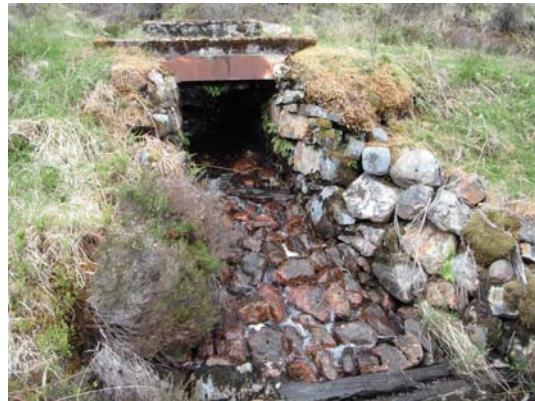
Photo No. 11: Culvert, from S.
