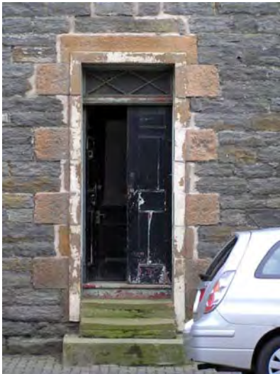
Front door to Princes Street
