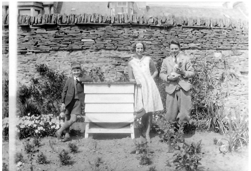
Photograph taken within the garden of 30 Princes Street showing the extension to the height of the wall © Manson Collection
