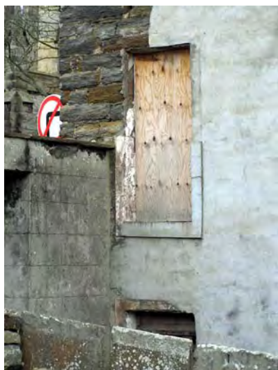
Windows inserted at the west gable
