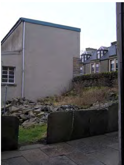
Spoil from demolitions within the garden
