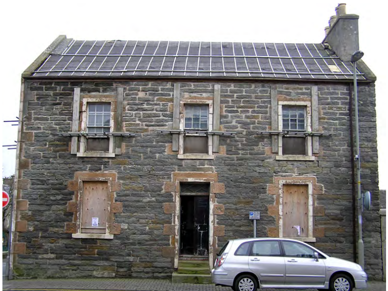
Elevation to Princes Street
