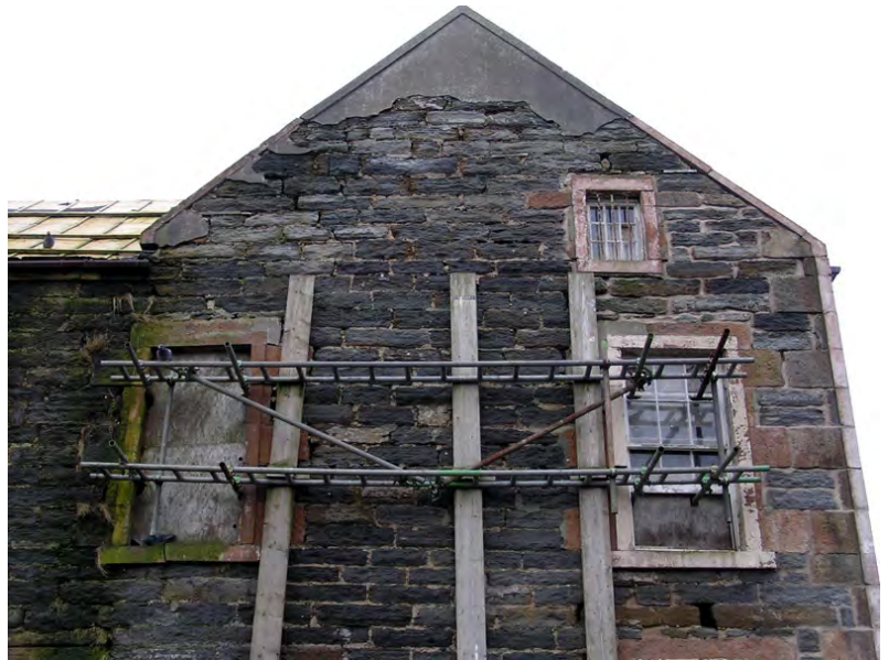
Temporary stabilisation works at the east gable
