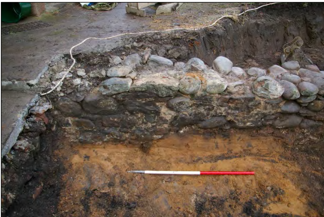
Plate 6 S end of wall from SE: no foundations, built on sand. This section was clearly a repair and contained lime mortar.
