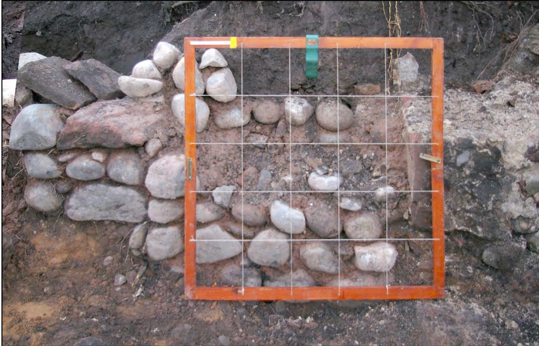
Plate 9 Blocking in wall between buildings A (left) and B (right).
