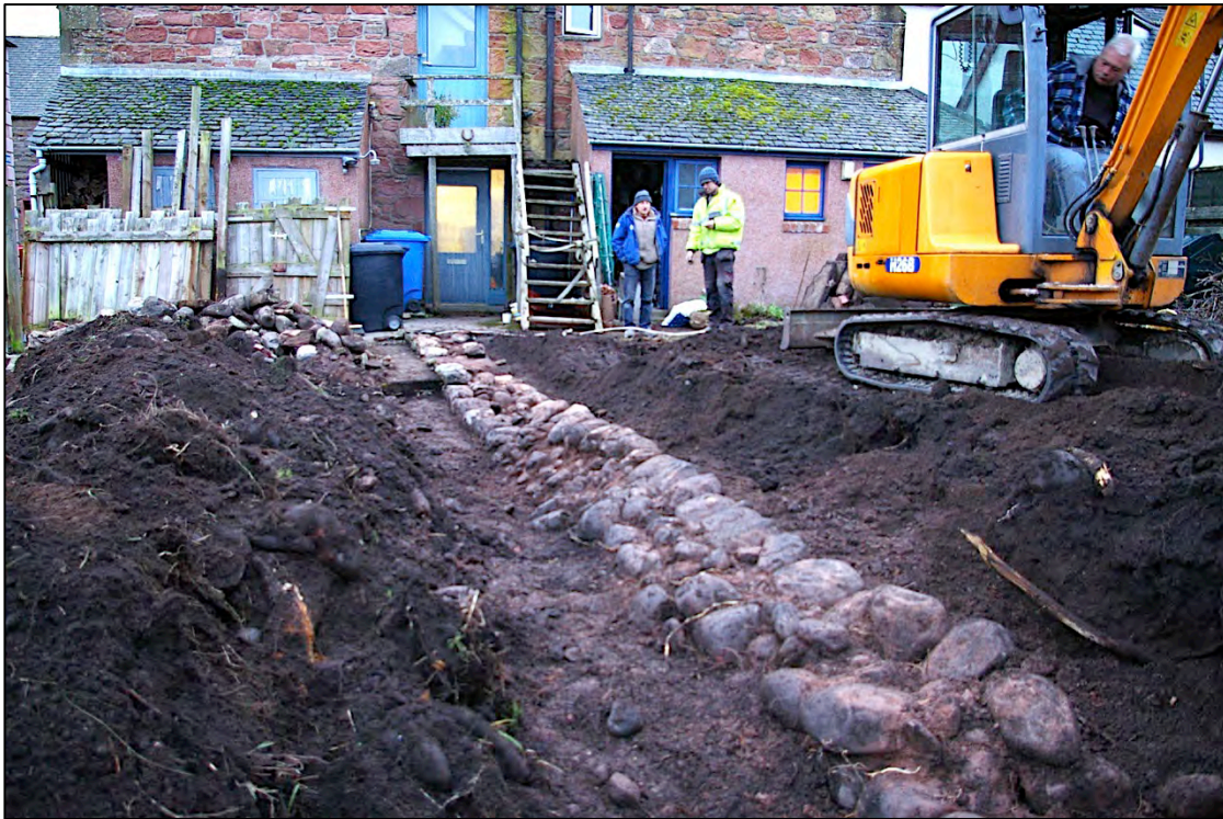
Plate 5 Wall (House A) as initially exposed
