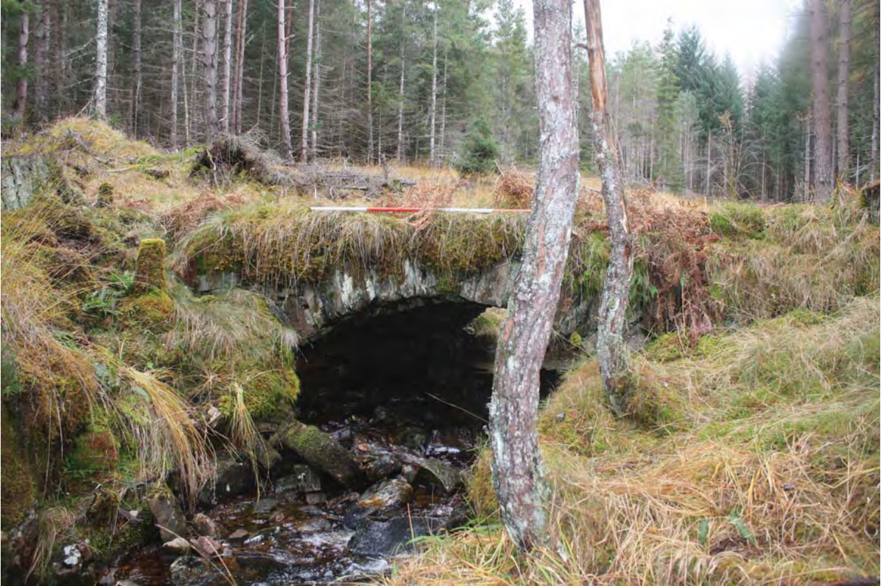
Plate 3: Bridge 007, general view of the north side from the NNW
