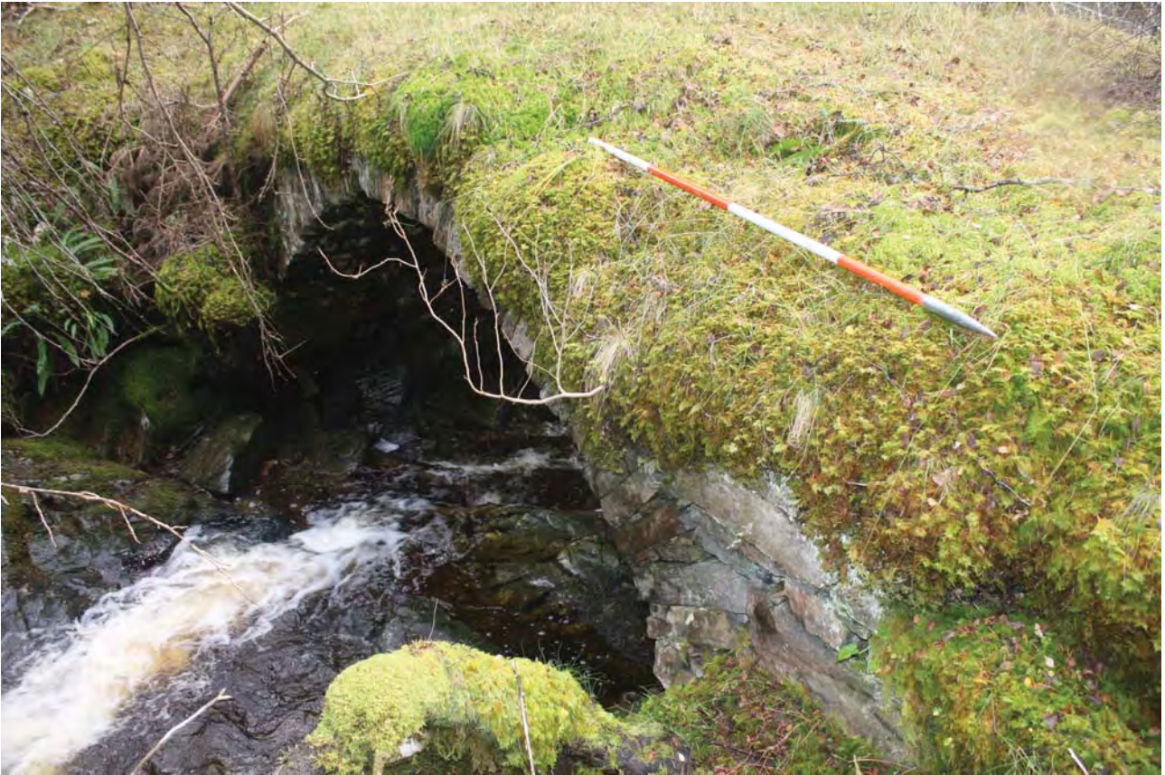
Plate 9: Bridge 009, general view of the south side from the SEE
