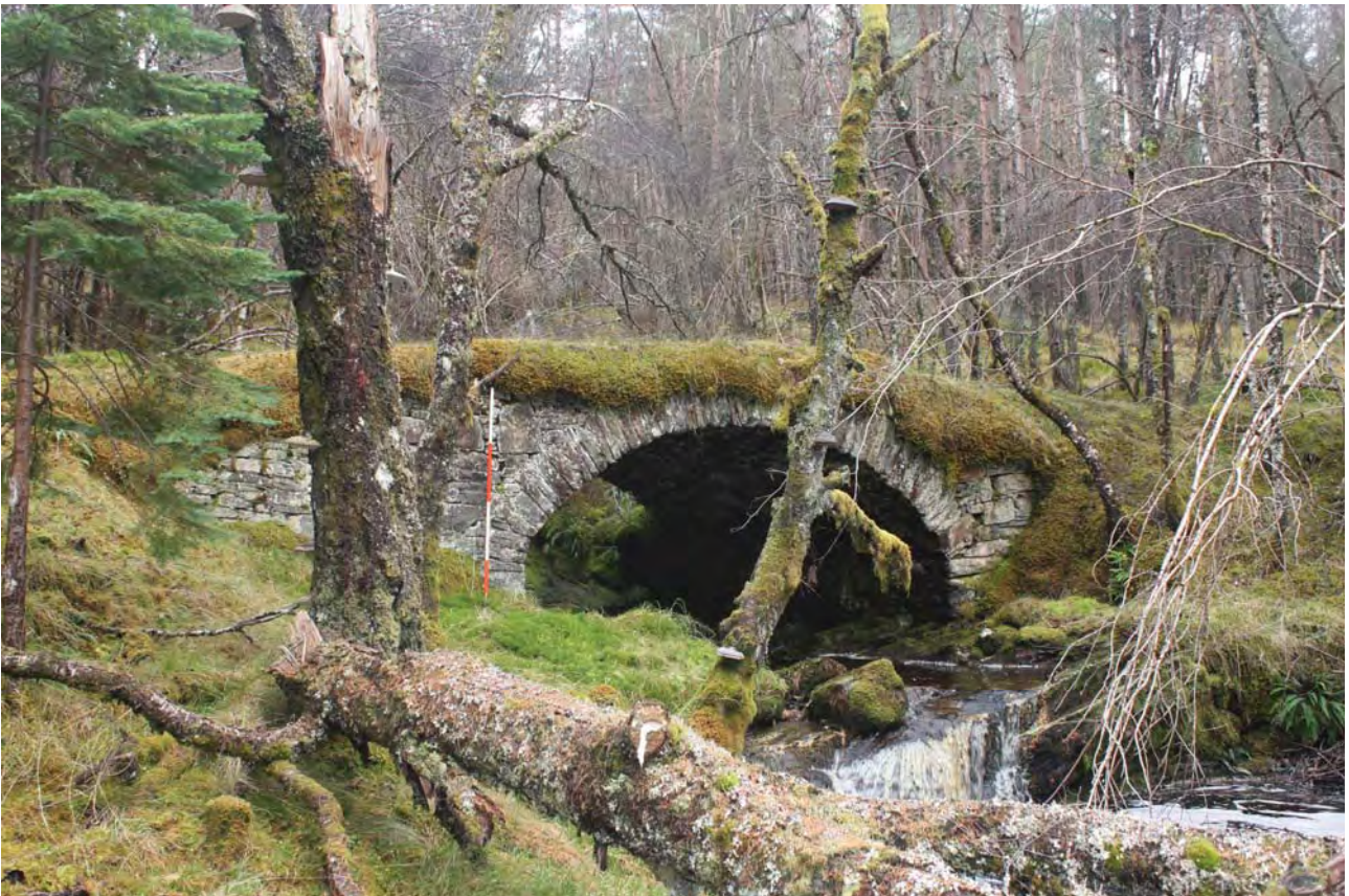
Plate 12: Bridge 009, general view of the north side from the north-east
