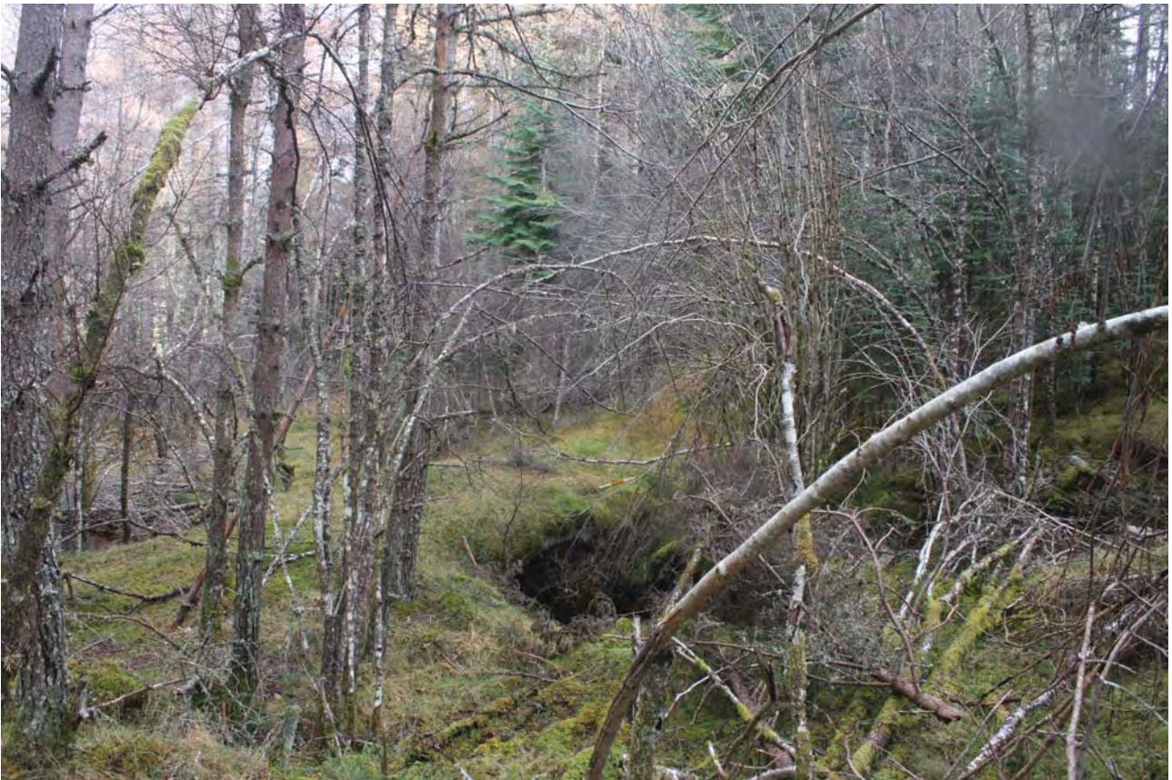
Plate 10: Bridge 009, general view of the south side of the bridge and the road over the bridge from the south-west
