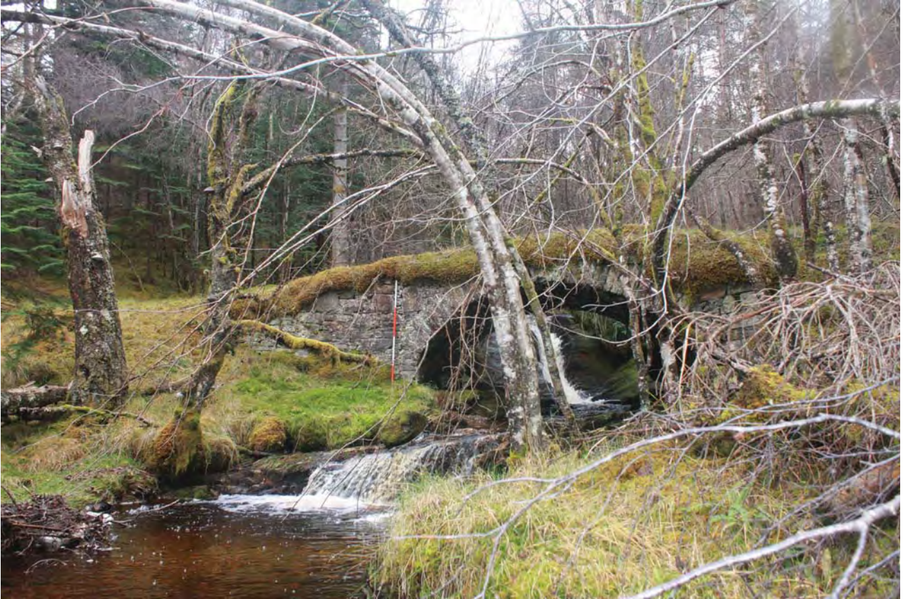
Plate 11: Bridge 009, general view of the north side from the NNW
