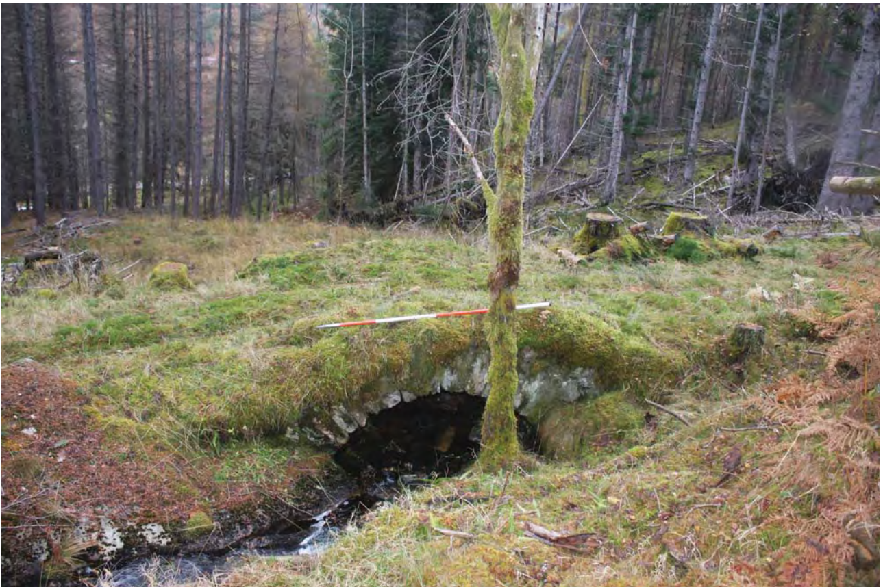
Plate 6: Bridge 008, general view of the south side from the south-west
