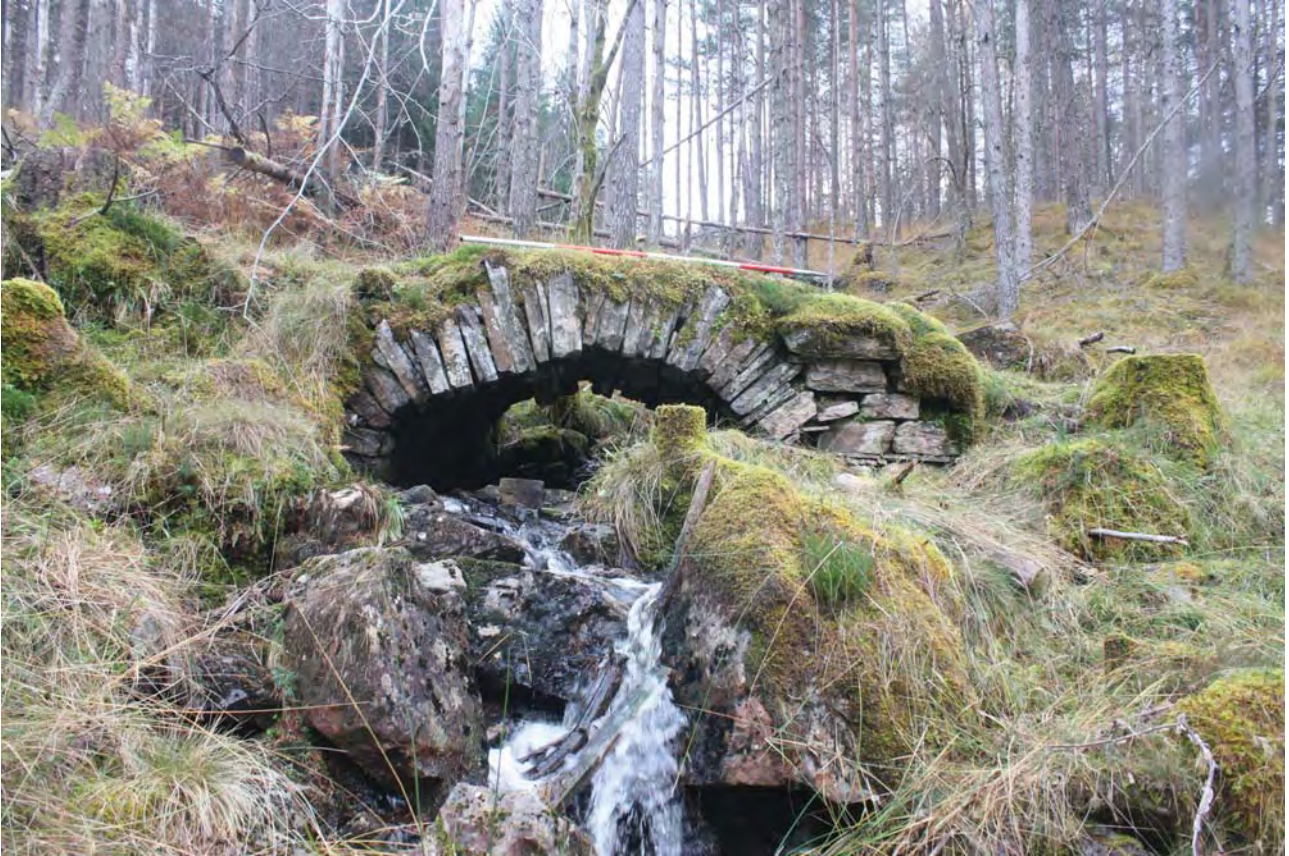
Plate 7: Bridge 008, general view of the north side from the north
