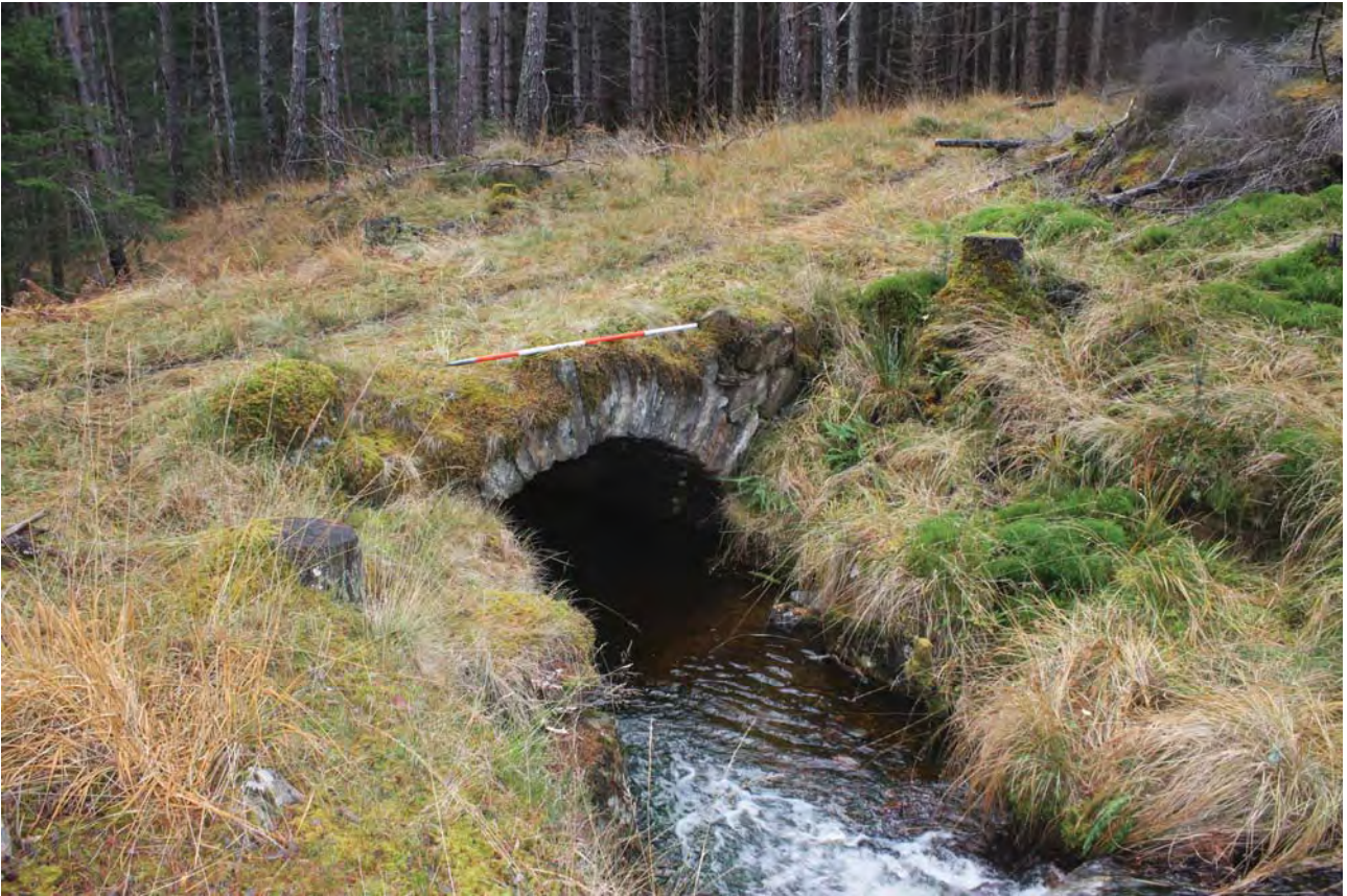
Plate 1: Bridge 007, general view of the south side from the south-west
