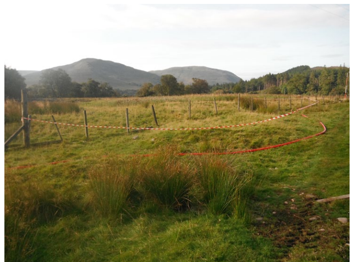
Fig. 18 - Demarcated structure on the cable trench route.
