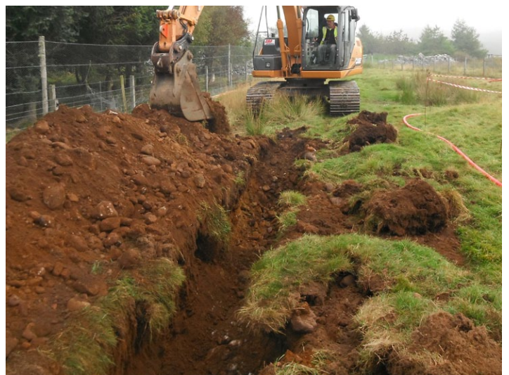
Fig. 20 - Cable trench alongside demarcated feature in Fig 18.
