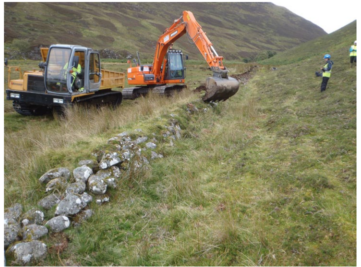
Fig. 10 - Removal of wall A2.
