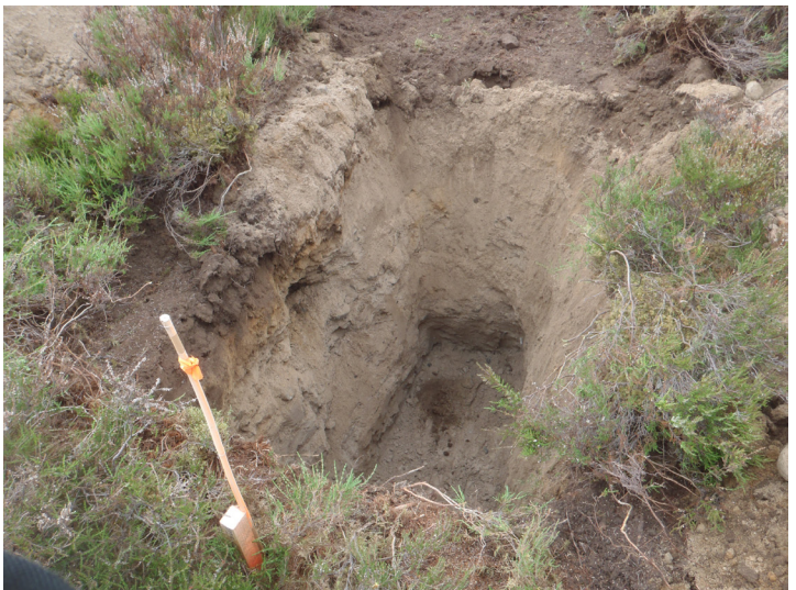
Fig. 20 - Excavation for pole 125
