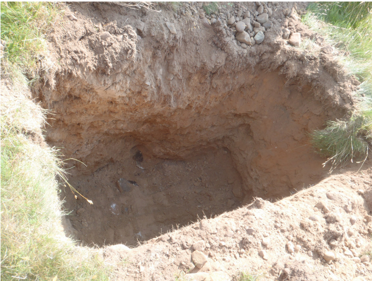
Fig. 13 - Excavation for pole 4
