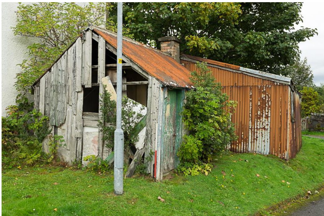
Plate 3: The cabin building, with the tin-clad garage situated behind
