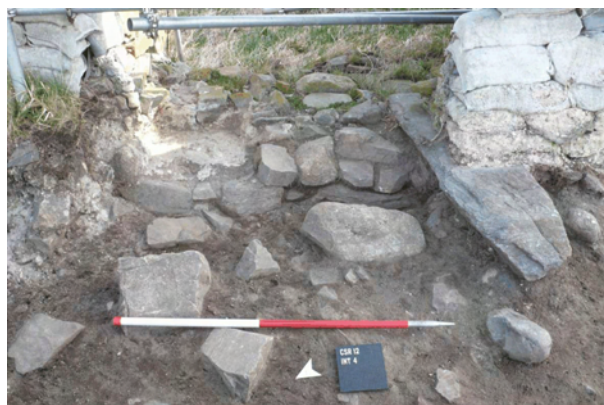
Plate 3 Evaluation trench showing the remains of foundations of garderobe turret (scale 1.0m)
