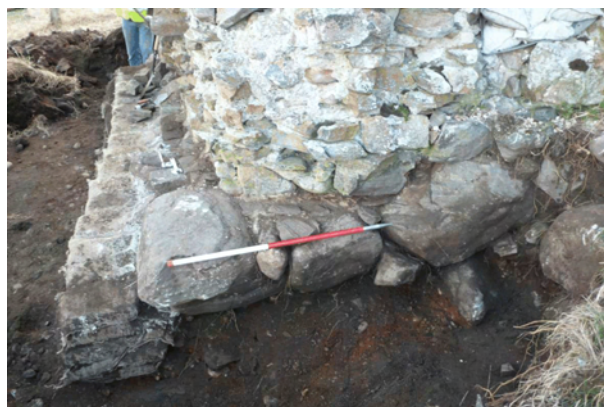
Plate 2 Foundations of northwest tower following consolidation (scale 1.0m)
