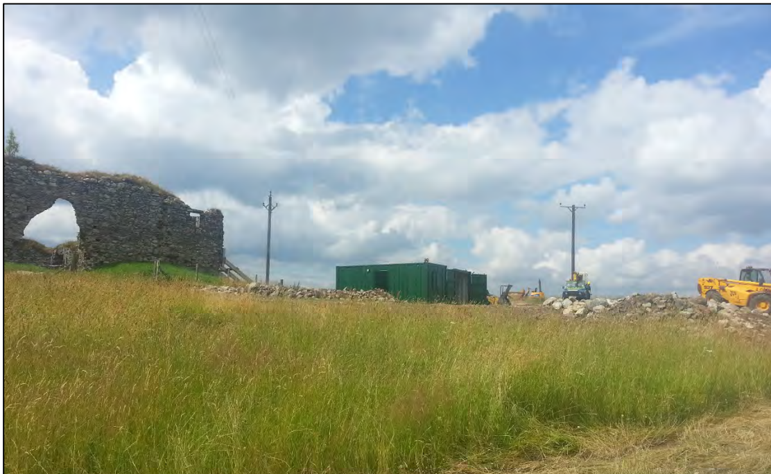
Plate 4: Old and new electricity poles
