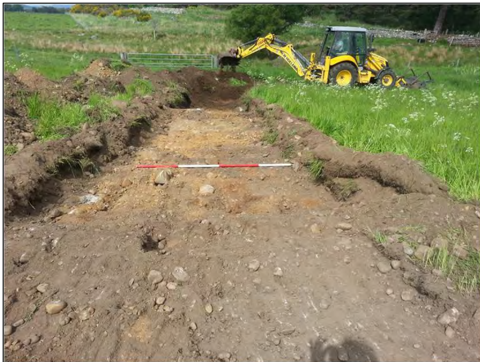
Plate 3: Stripping for contractor's compound (above) and access track
