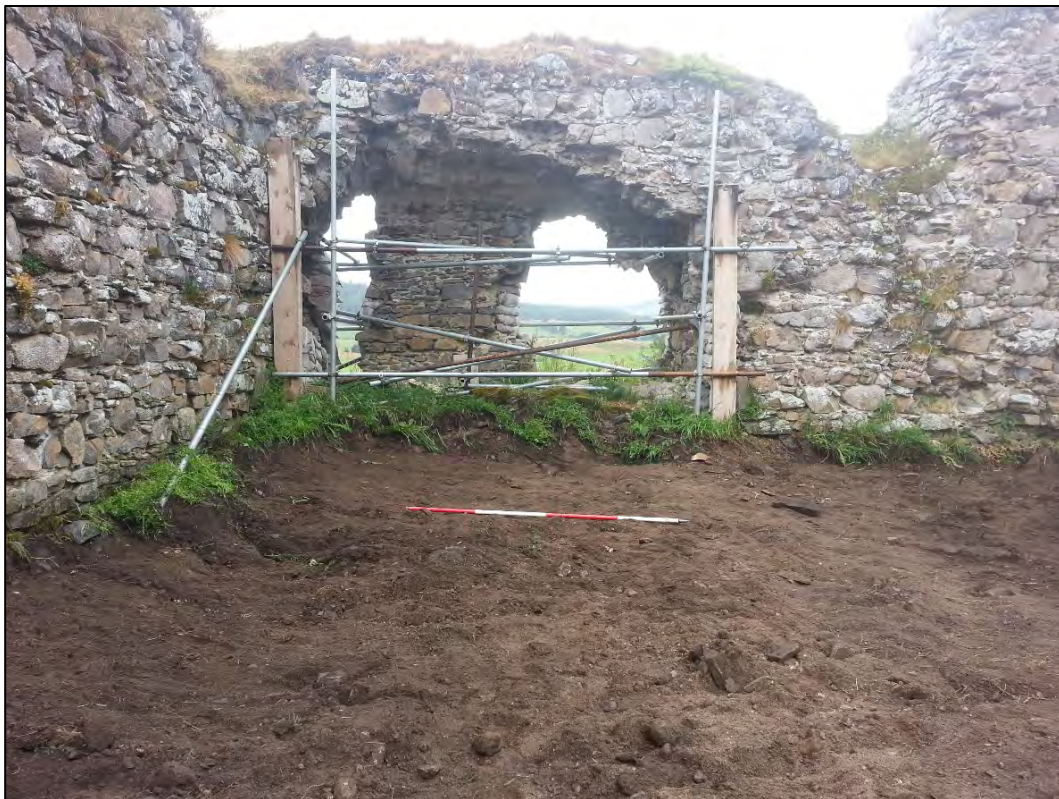
Plate 7: Interior view NW along SW wall, following turf removal
