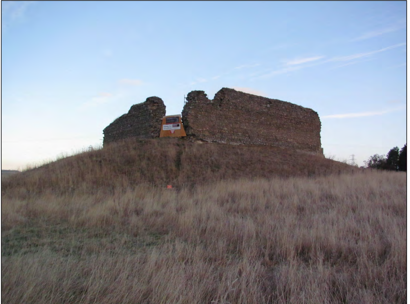
Plate 2 Castle under repair January 2014
