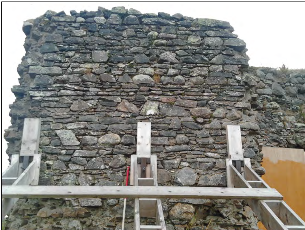
Plate 8: Ex-34 showing tower
