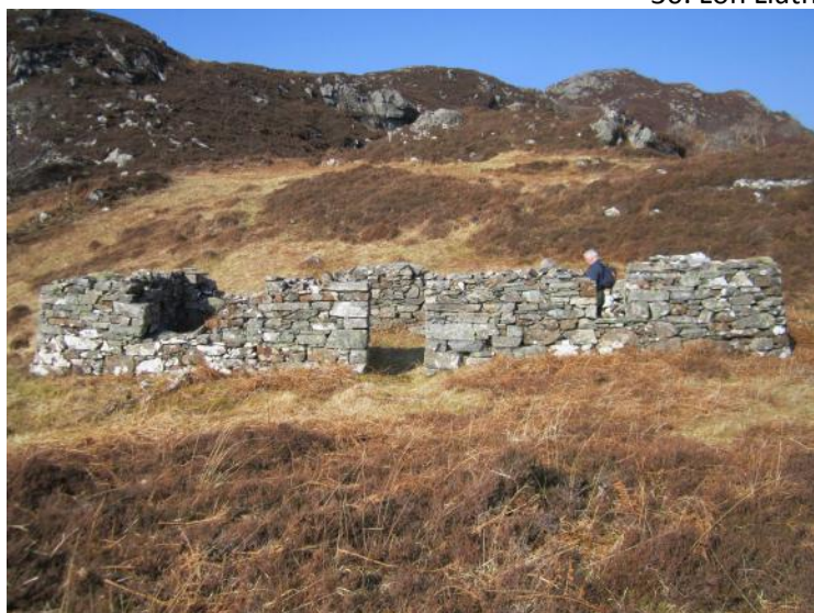
Wp 15 Building c. 11x6 metres looking north at NM 67402 83883
