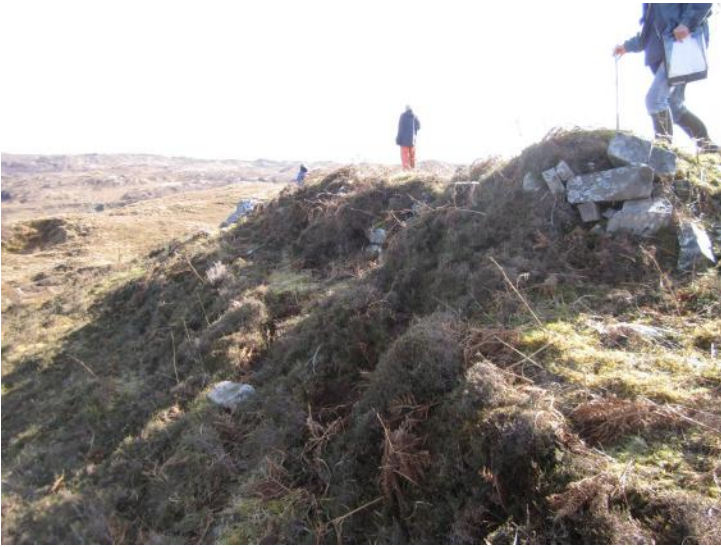
Wp 10 View east of the north side revetment of the feature at NM 63407 85064
