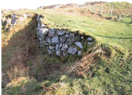
Wp 43 Causeway of old track at NM 64650 84989
