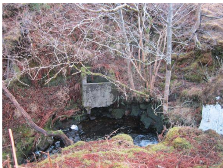
Wp 3 Concrete tank on the An Garbh Uillt at NM 65385 84984
