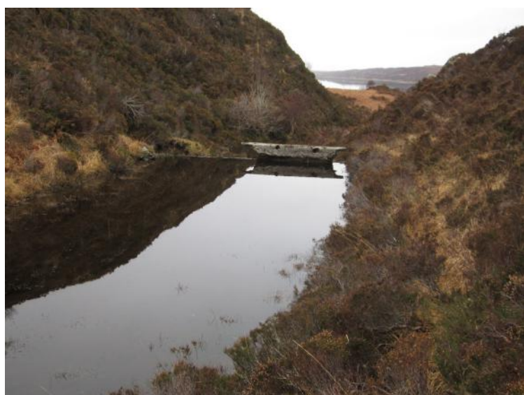
Wp 19 Looking NNW to dam on the An Garbh Uillt at NM 65518 84649
