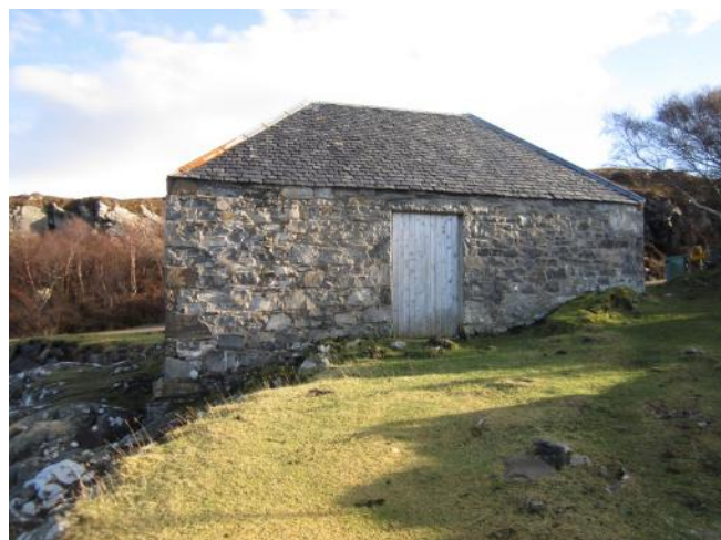
Wp 3 Storehouse built 1885 NM 62722 85110
