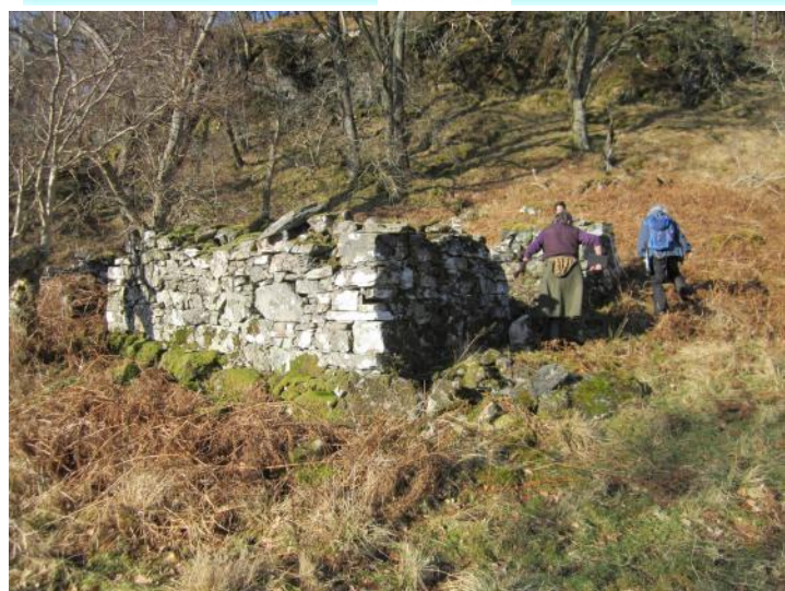
Wp 17 View to the north-east of building at NM 68078 84142
