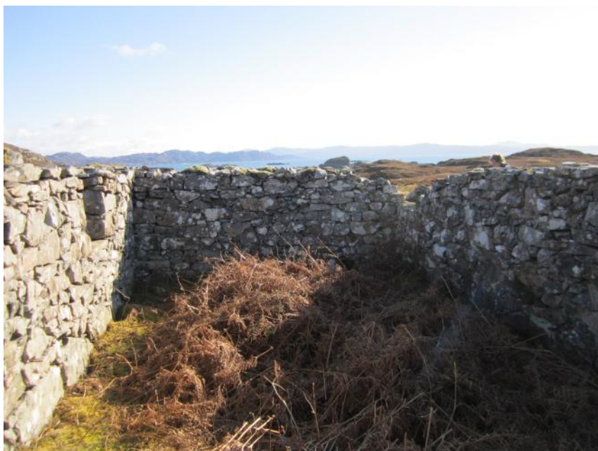
Wp 30 Interior view looking south of the large ruin 10 x 5 mtrs with walls to c. 1.5 mtrs high at NM 62810 83412
