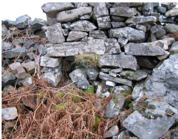
Wp 30 NM 64324 83959 Detail of stone work in 'Winnowing Barn'
