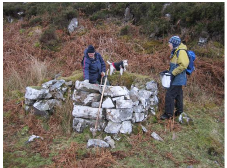
Wp 16 Small storage building at NM 65201 84901
