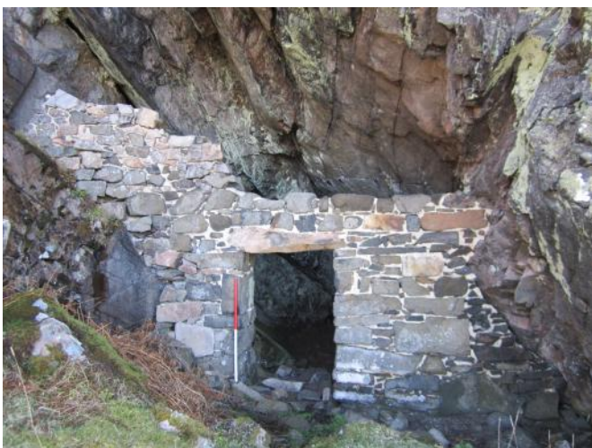
Wp 26 Detail of the wall at the Soap Cave at NM 62080 84797
