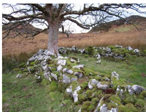
Wp33 NM 64365 83946 Detail of ruined walling on SE corner
