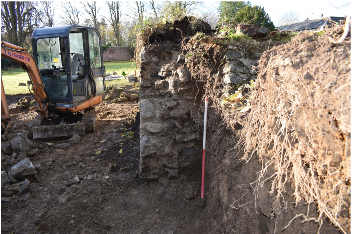
Plate 6 Machine dug section through the revetment wall (006)
