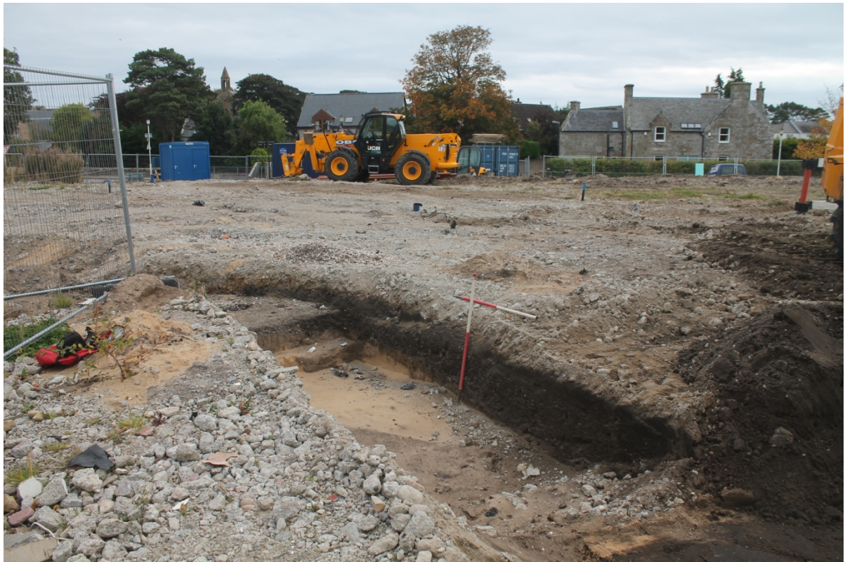
Plate 1: Development site prior to excavation with demolition rubble (201) spread across it
