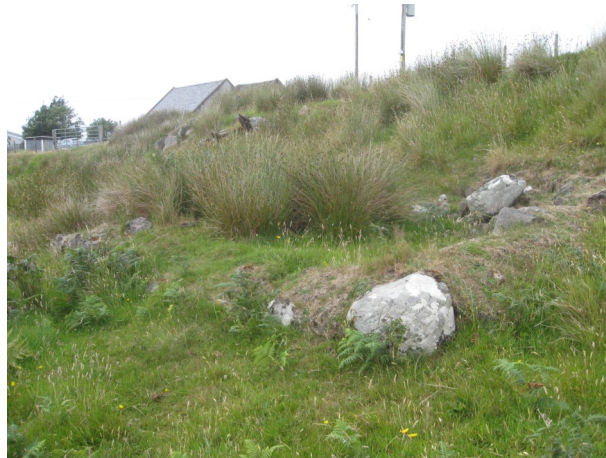
35 NG 74253 86391 41m footings of building down bank
