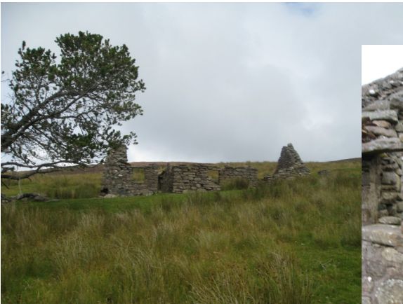
52 NG 74640 86547 95m ruined house
