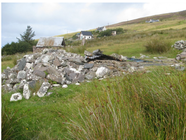
50 NG 74569 86516 78m stone footings of building overlain by concrete platform filled with stones
