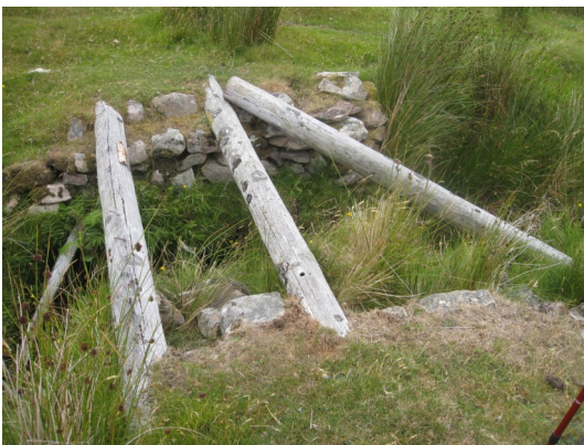
19 NG 73930 87042 40m stone bridge
