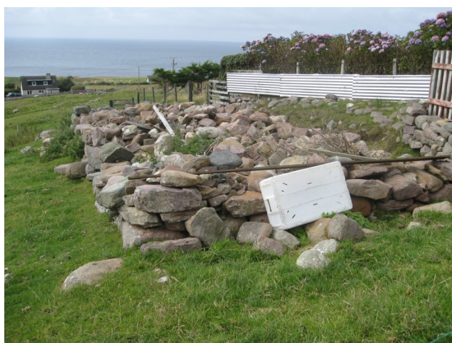
65 NG 74402 86486 57m ruined building partly reused as shed , otherwise filled with stone clearance
