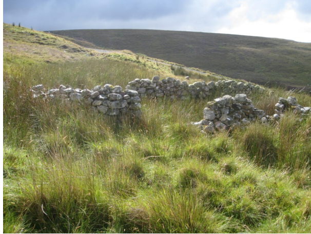
39 NG 74698 86679 118m ruined barn/byre
