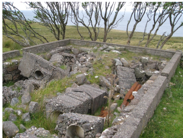
20 NG 74028 87068 52m ruin of concrete shuttering overlying older sandstone footings
