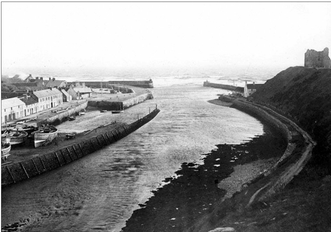
Plate 1: View of Helmsdale and the harbour completed in 1818. Above the harbour on the right are the ruins of Helmsdale castle, now destroyed. Copyright SCRAN, ID 000-000-574-765-C.
