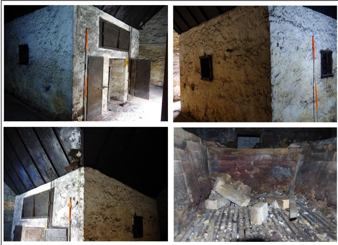
Figure 26 – The Kiln Room including view of brick kiln-chamber. Scales 2m
