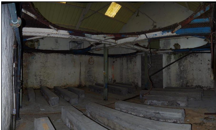
Figure 22 – Interior of the Wash Room. Facing W. Scale 2m
