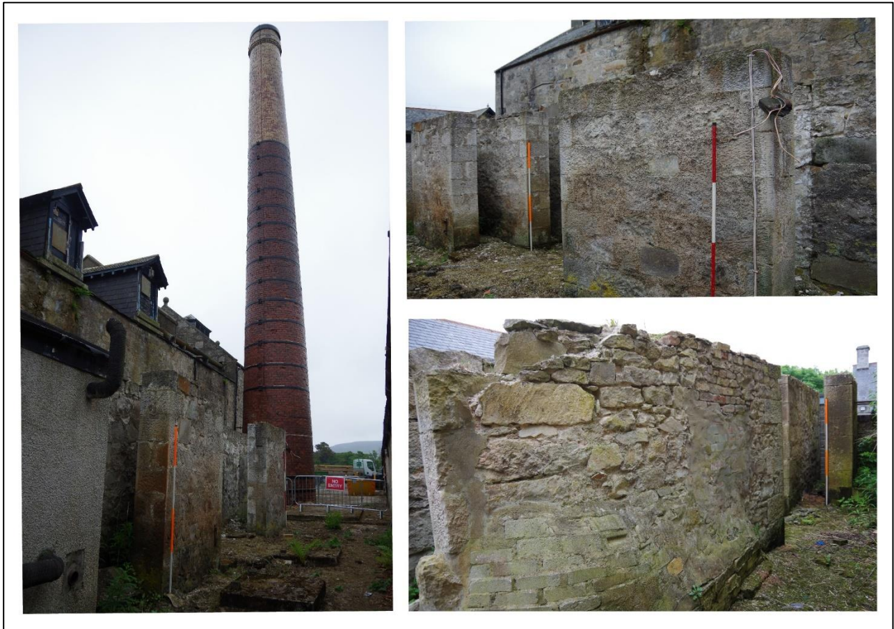
Figure 30 – The Worm Tub foundations and Chimney. Scales 2m
