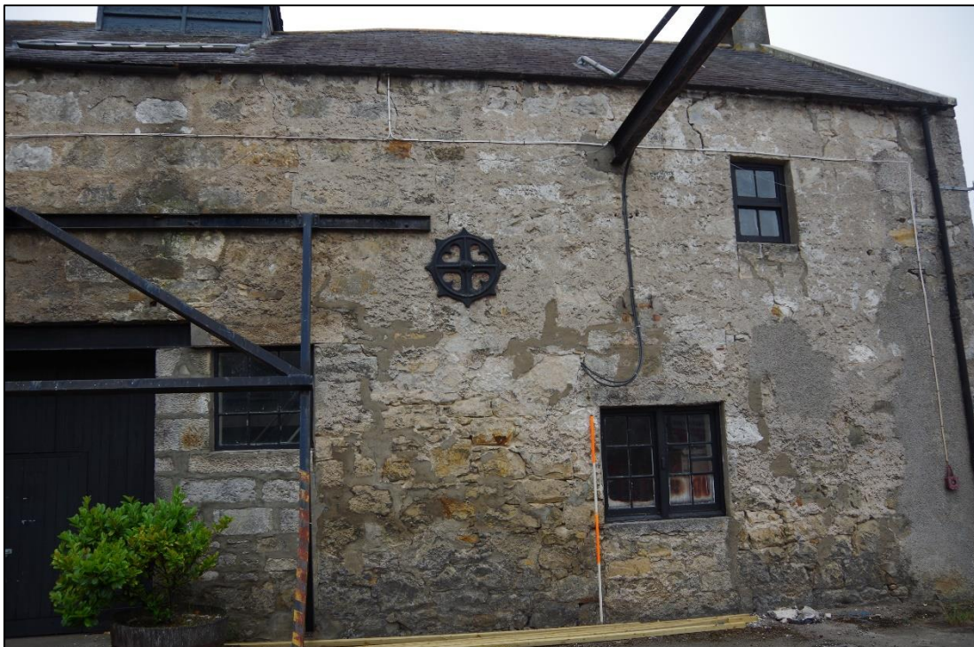
Figure 19 – The south facing elevation of the Stills Room. Scale 2m
