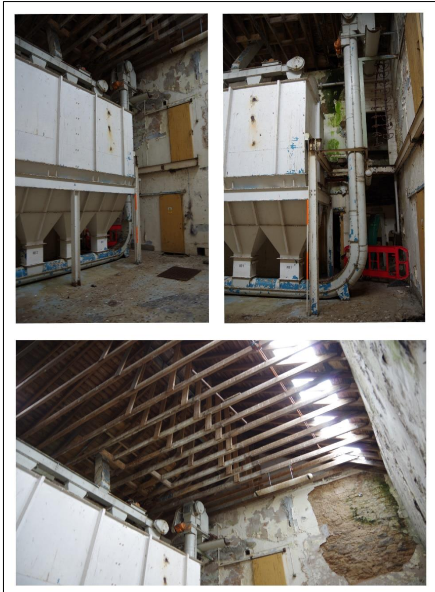
Figure 21 –Interior hoppers and roof structure of the Grist Room. Scales 2m
