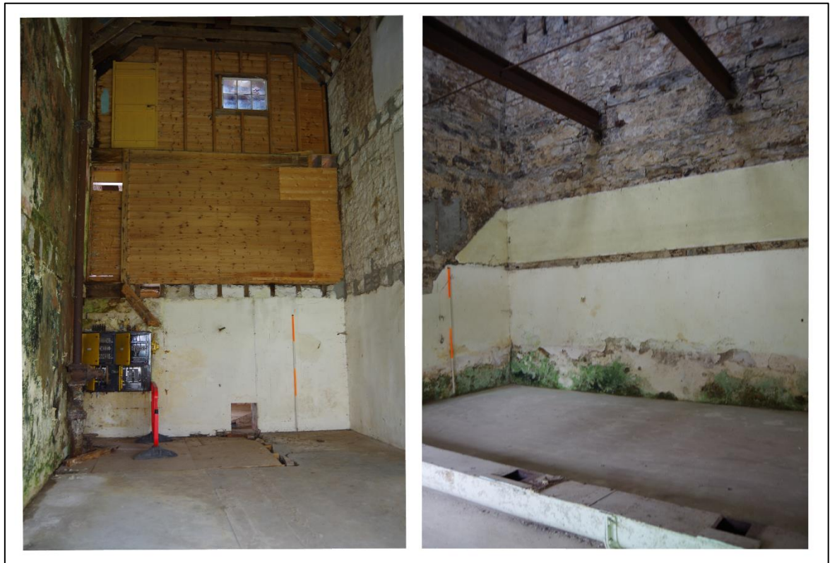
Figure 27 – (from left) The interior of Rooms V and W. Scales 2m
