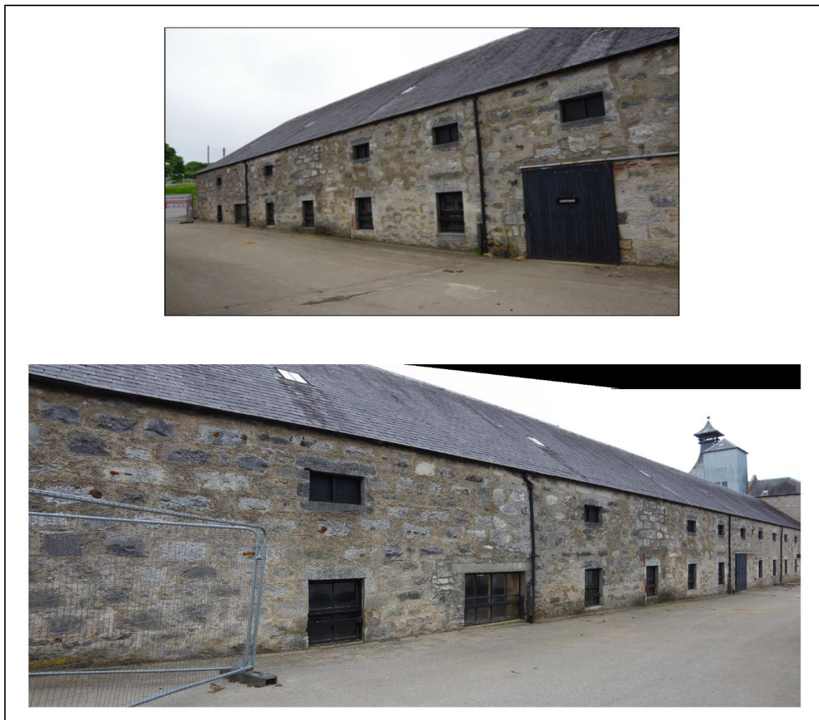
Figure 7 – The east facing elevation of the Cooperage building. Facing SW (top) and N. Scales 2m
