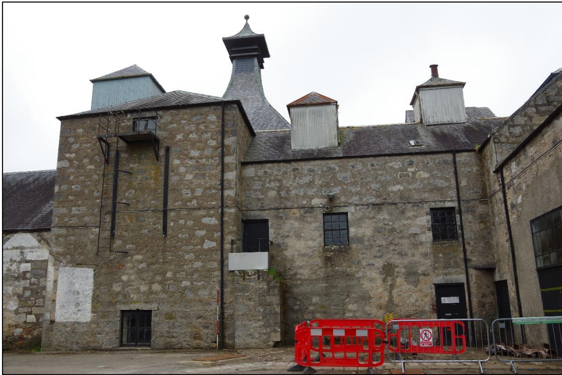
Figure 18 – The east facing elevation of the Milling Room and Room W with the Kiln cupola behind. Scale 2m
