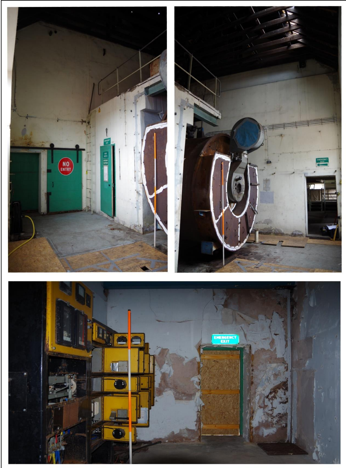
Figure 25 – The Boiler and Switch Rooms. Scale 2m
