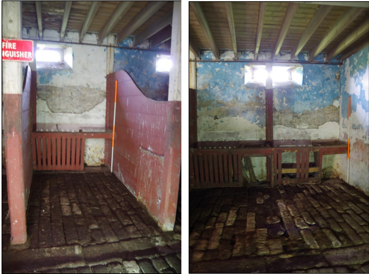
Figures 15 a and b – Horse stalls and sett floors in the Stable Block. Scales 2m
