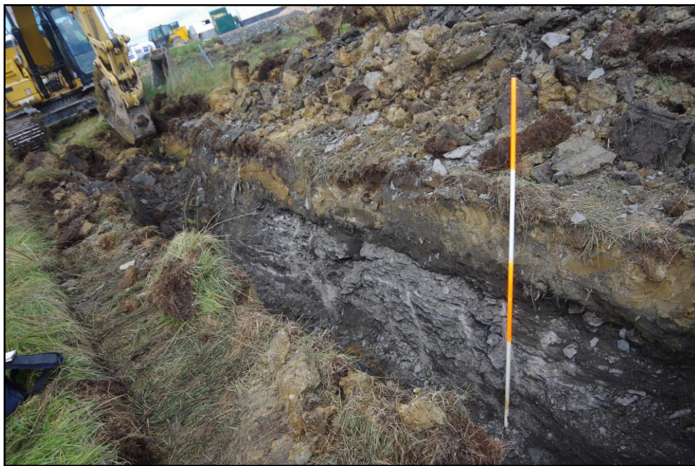
Plate 5 – Excavation using the ripper of bedded sandstone outcrop 104 in the northwest return, from CP22, looking N. Scale 2m
