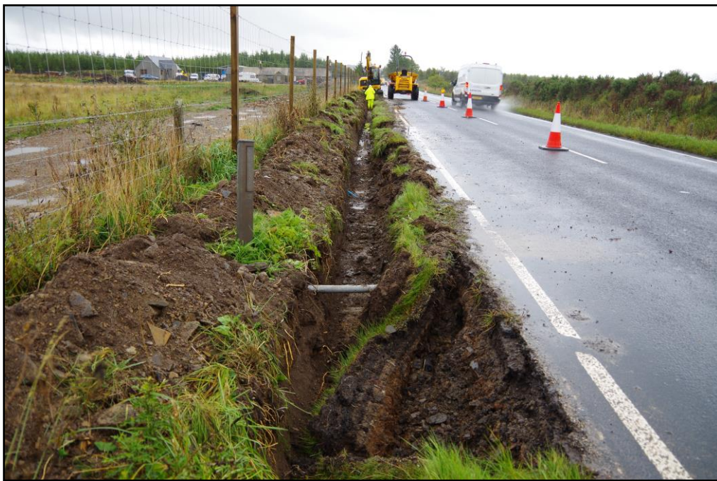
Plate 7 – General view of final stretch of cable trench excavated alongside the A9 carriageway, from CP46, looking N. No scale
