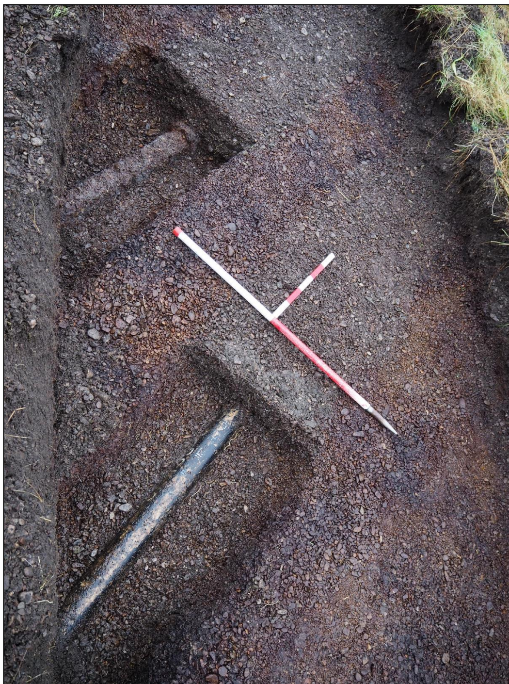
Plate 12: View of the two water main trenches and their respective cast-iron and asbestos pipes
