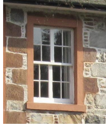
Fig. 44 8 over 8-pane sash and case window
