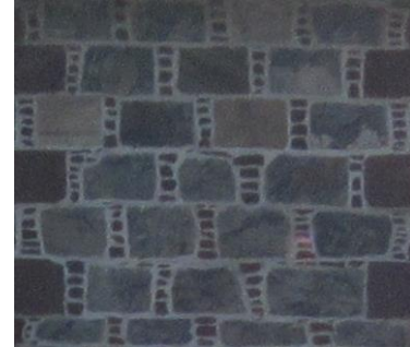
Fig. 41 Ladder pinning detail, lime mortar
