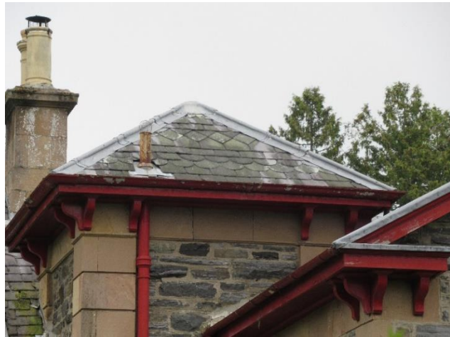
Fig. 38 Fish-scale and diamond slate tiling detail
