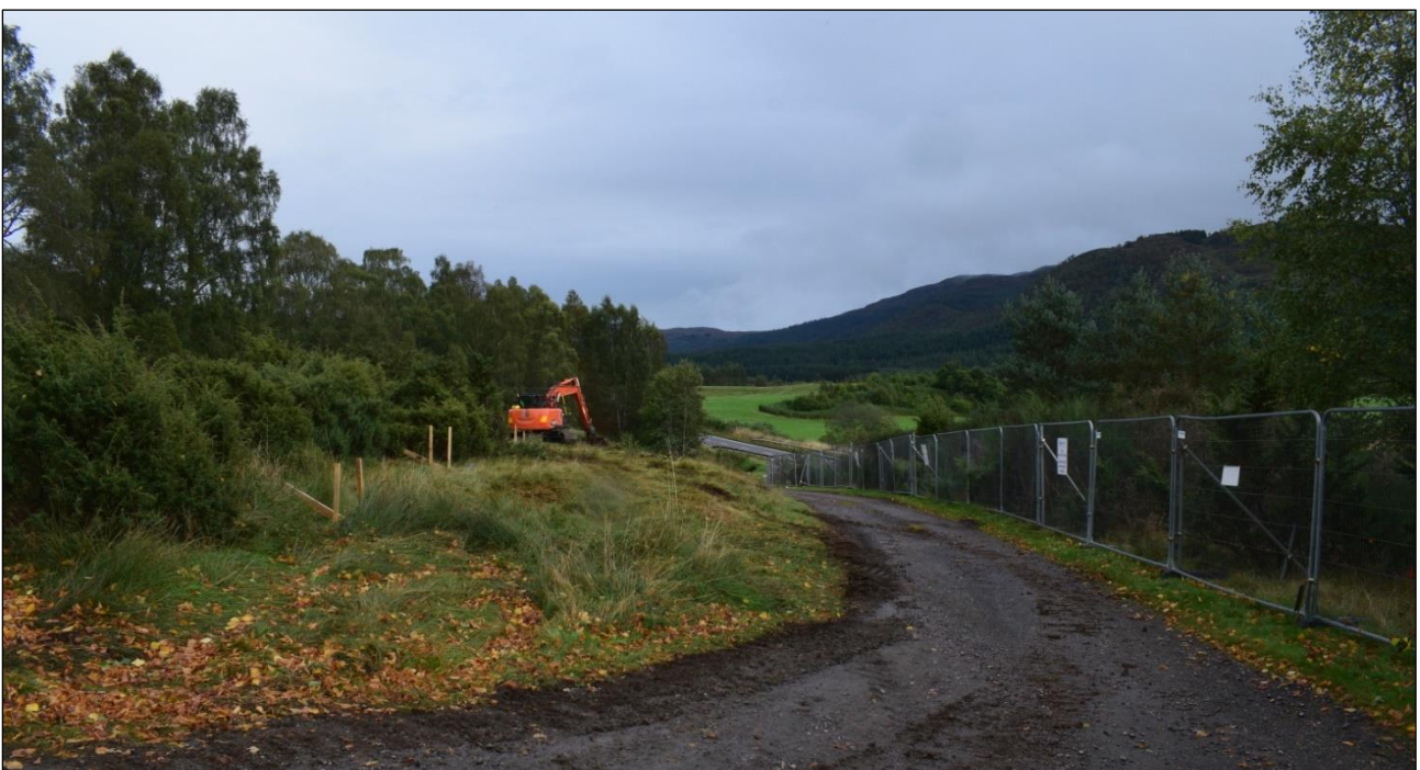
Plate 3: Pre-works view of Area 3 (access track from A887), facing east-southeast
