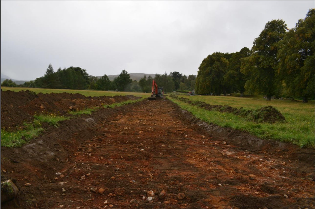
Plate 30: Post topsoil strip of Area 4 (access track), facing west-northwest
