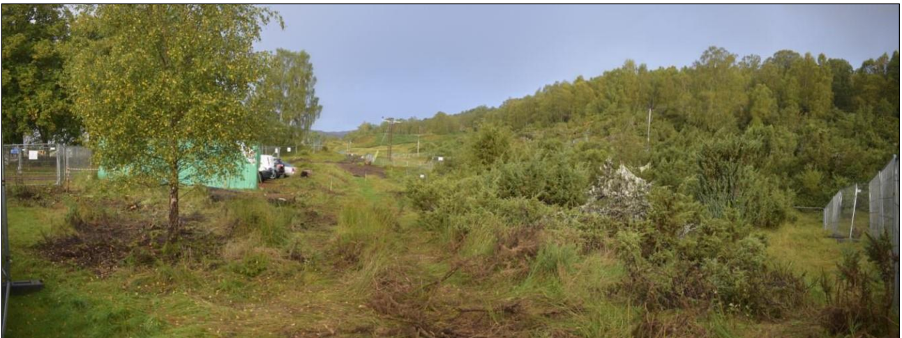
Plate 5: Pre-works image of Area 5 (substation and compound area), facing northwest
