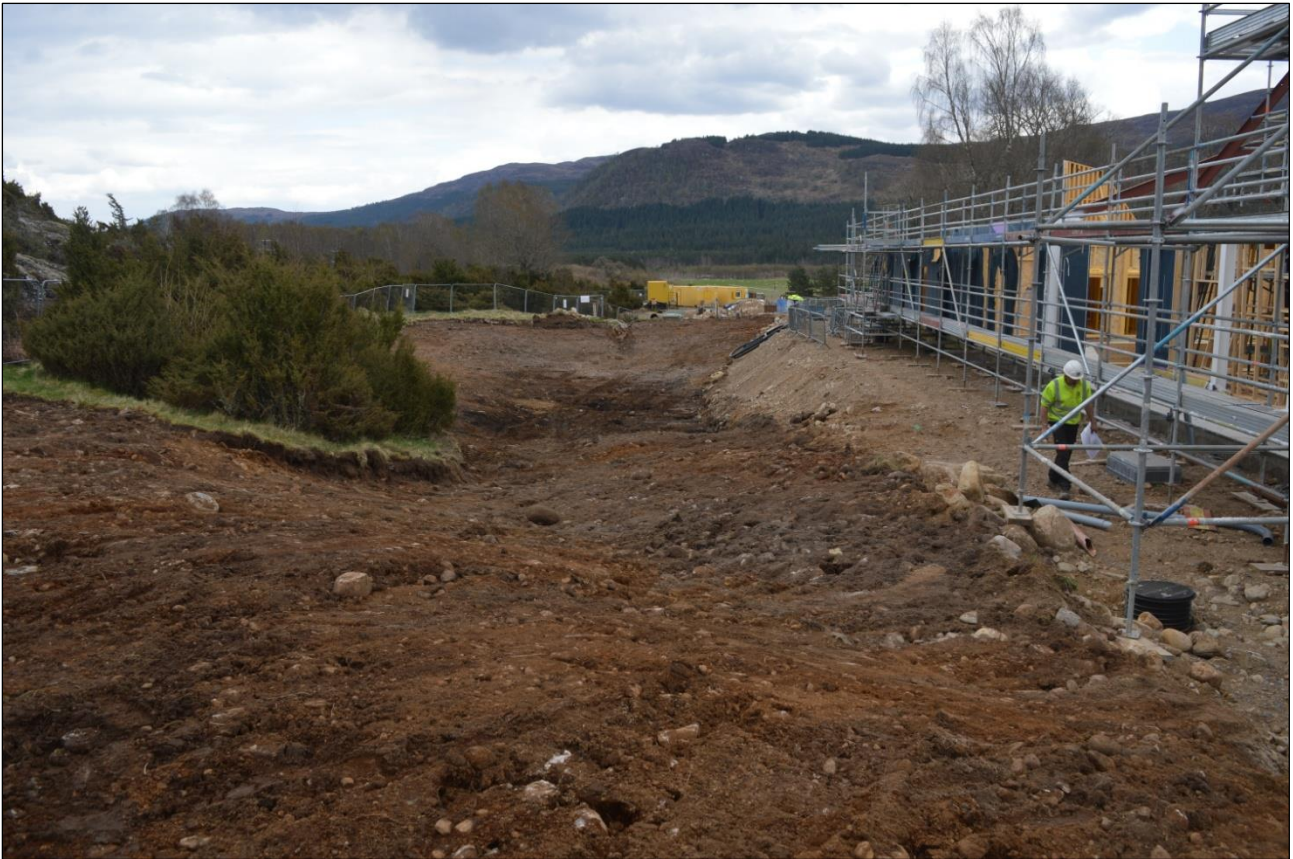
Plate 21: Post topsoil strip of the north side of Area 2, facing east
