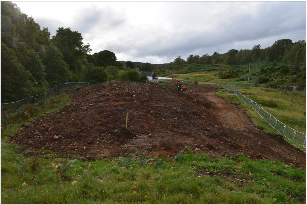
Plate 20: Post topsoil strip of Area 2, facing west
