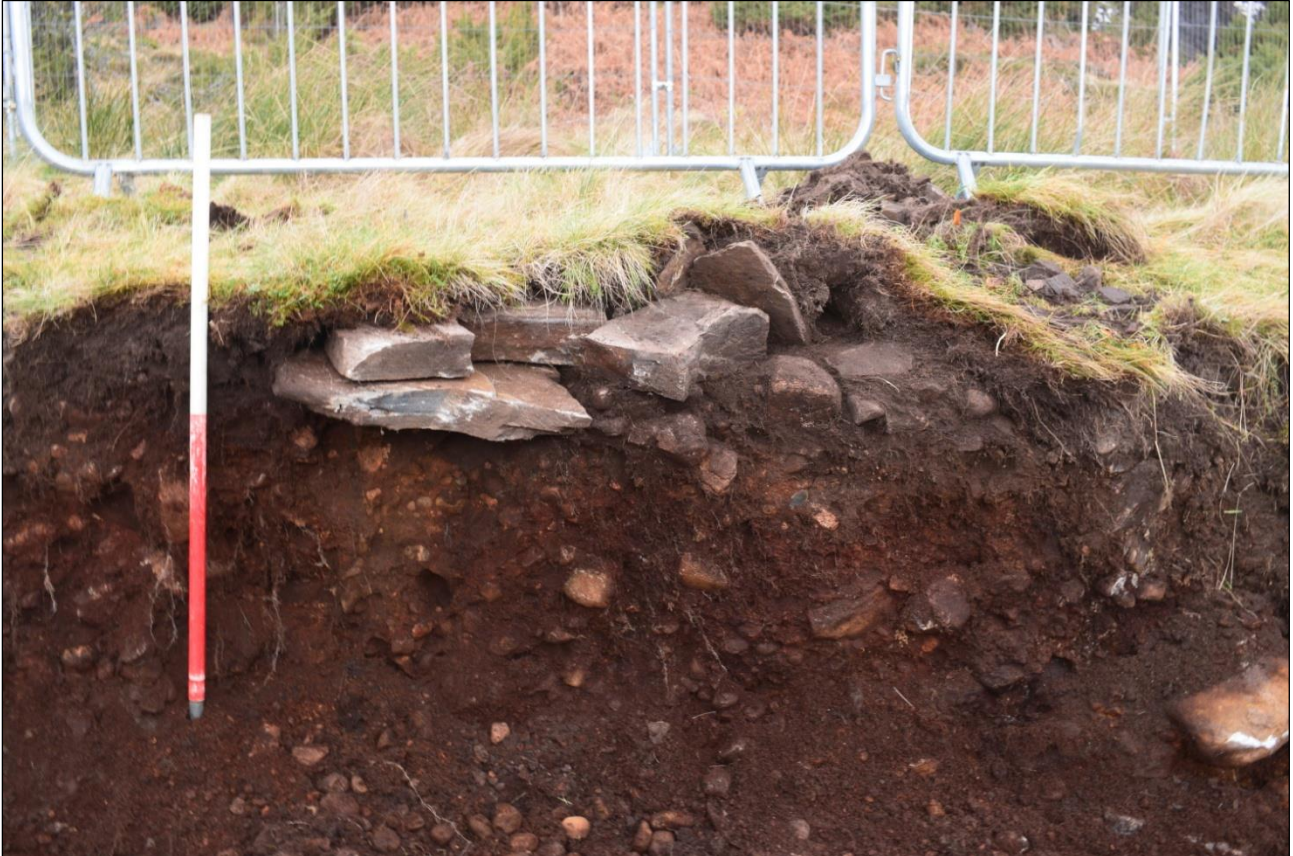
Plate 40: South-facing section of possible boundary wall [030] in cable trench
