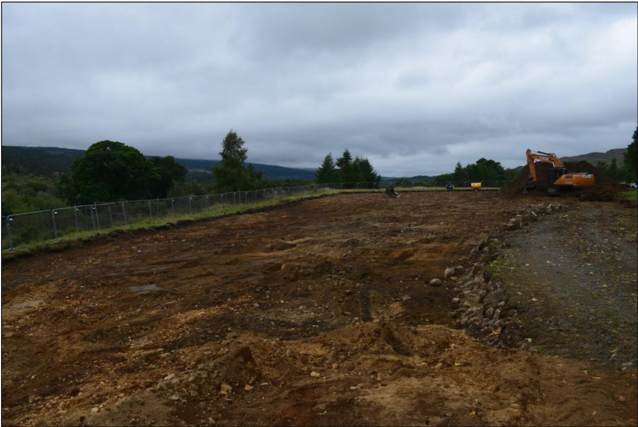
Plate 18: Image showing Area 1 post topsoil strip, facing west
