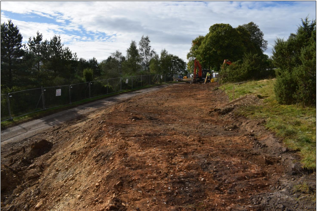
Plate 27: Post topsoil strip of Area 3, facing west
