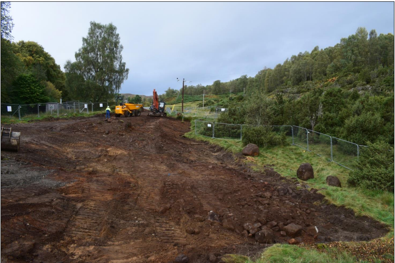
Plate 32: Post topsoil strip of Area 5, facing west
