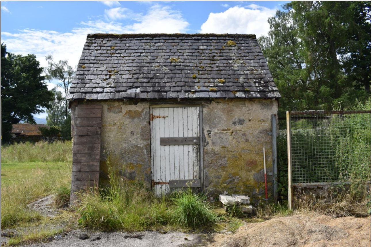
Plate 16: East-northeast elevation of cold store
