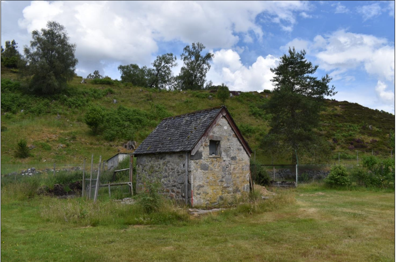
Plate 15: Record view of cold store, facing north-northeast
