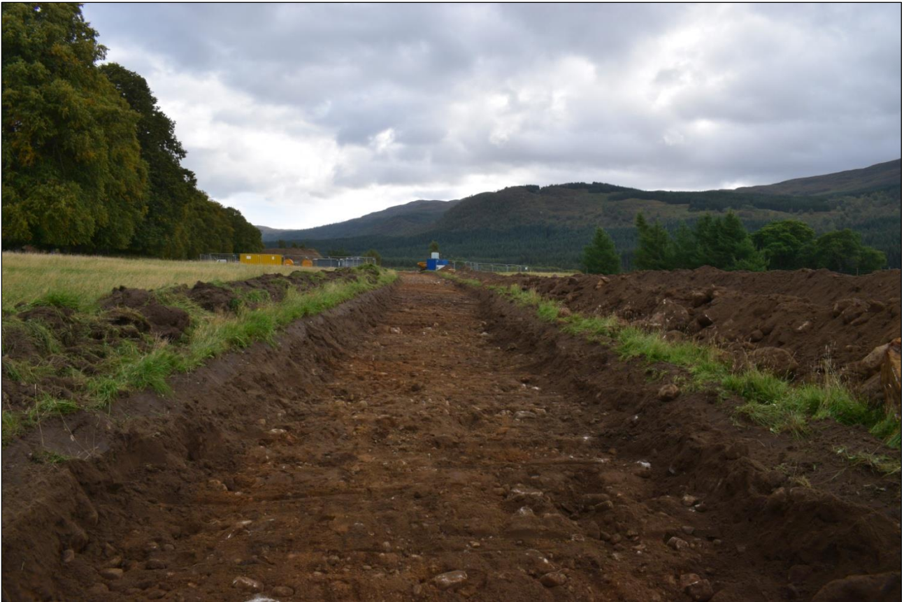
Plate 31: Post topsoil strip of Area 4 (access track), facing east-southeast
