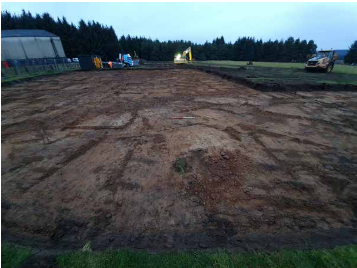
Plate 2: Post excavation of construction compound, facing north
