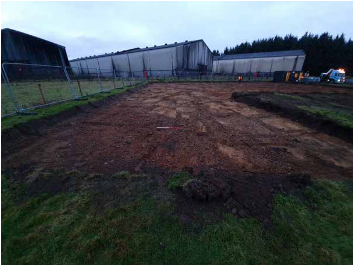
Plate 3: Post excavation of construction compound, facing west-northwest
