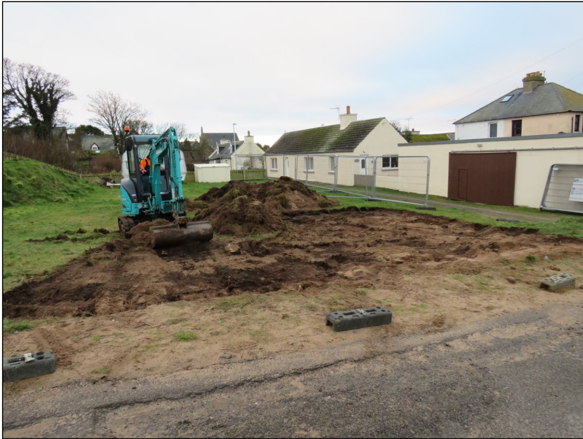
Figure 11 – Topsoil stripping in progress. Facing W
