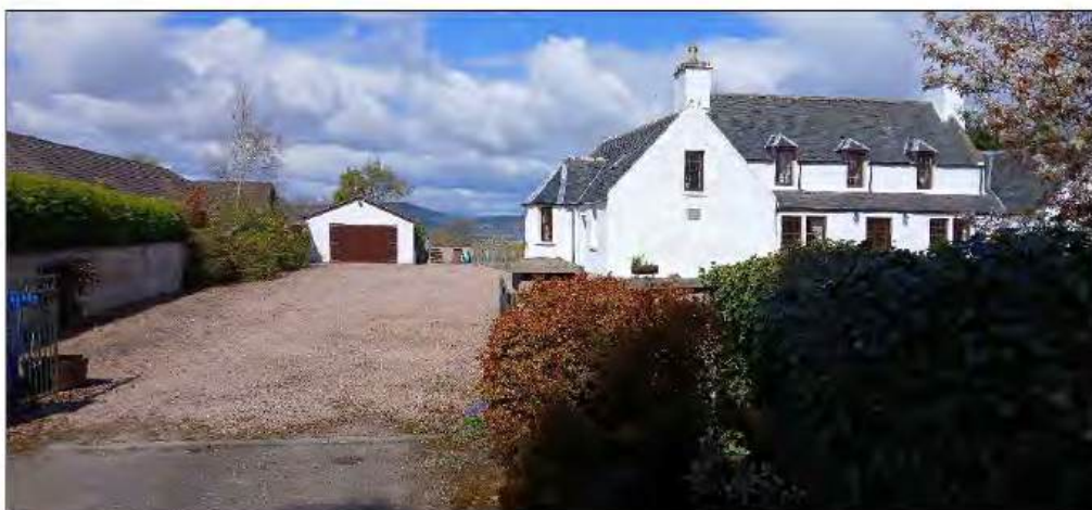
Plate 18: NW facing view of Cradle House (Asset 4)
