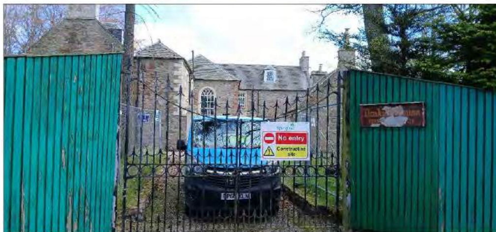
Plate 22: East facing view of Drakies House (Asset 9)
